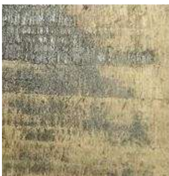
Fig. 9 Wood without coating
