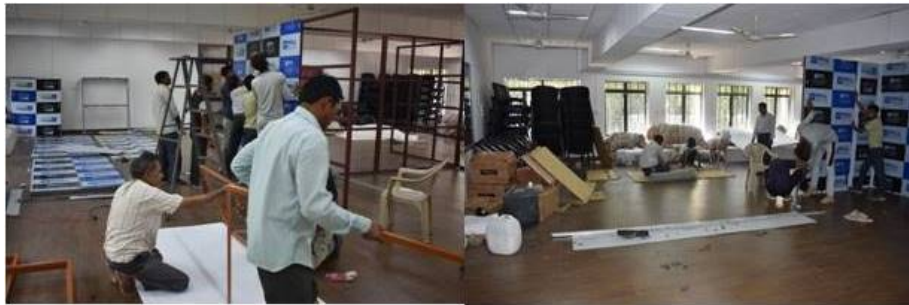
Fig. 48 Paneling work of TDC at IFP, Ranchi
