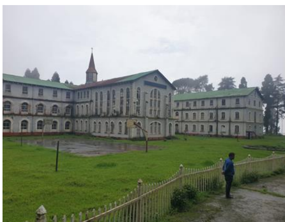
Front view of the building
