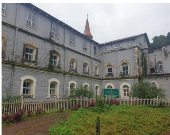
Rear view of the main building hostel rooms
