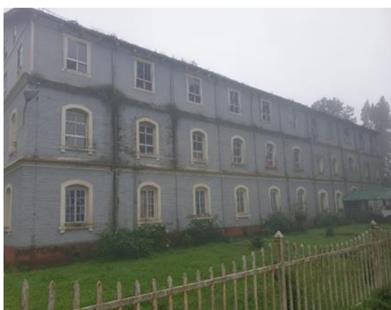
Side view of the west wing of the building
