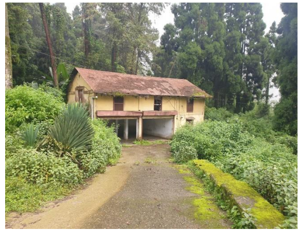
Garage and generator room
