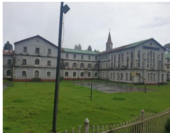
Building view of middle and east wings
