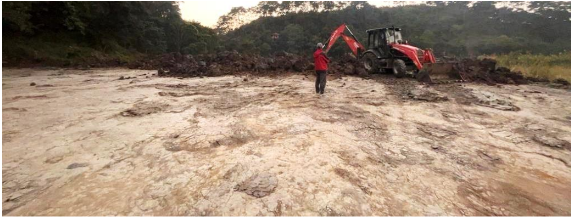
Figure 3: Landfilling activity using tipper and earth-movers in the CBC site
