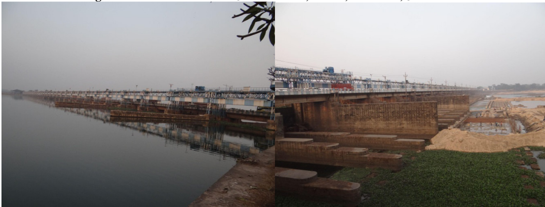
Fig. 13 Durgapur Barrage on Damodar River near Durgapur City, West Bengal
