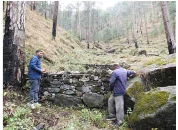
Team First, Uttarkashi Division, Dunda Range, Dhanari C.No. 13 site, Activity: Gully Plugging, Latitude: 30.66297222, Longitude: 78.45898889.
