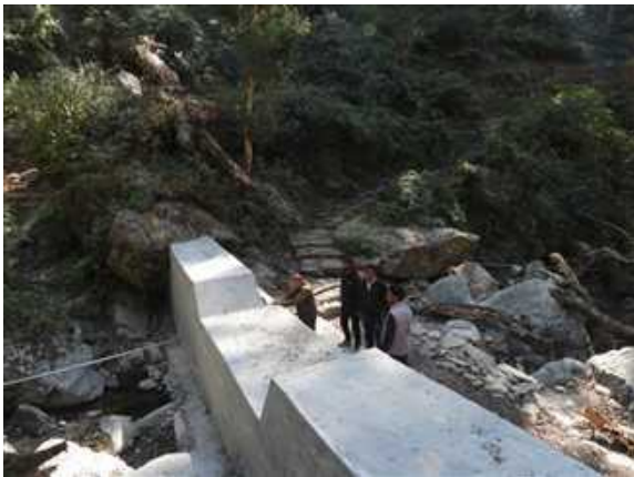
Team Three, Nainital Division, South Gaula Range, Burtoli Nala Okhalkanda site, Activity: Not specified, Latitude: 29.31811111, Longitude: 79.79088889.
