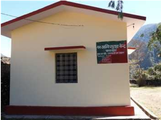
Team First, Uttarkashi Division, Dunda Range, Bandarkot site, Activity: Fire Crew Station, Latitude: 30.74194444, Longitude: 78.36055556.
