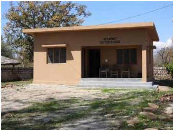
Team Fifth, Rajaji Tiger Reserve, Beribada Range, Activity: Chowki Repairment, Latitude: 30.03583333, Longitude: 78.02027778.
