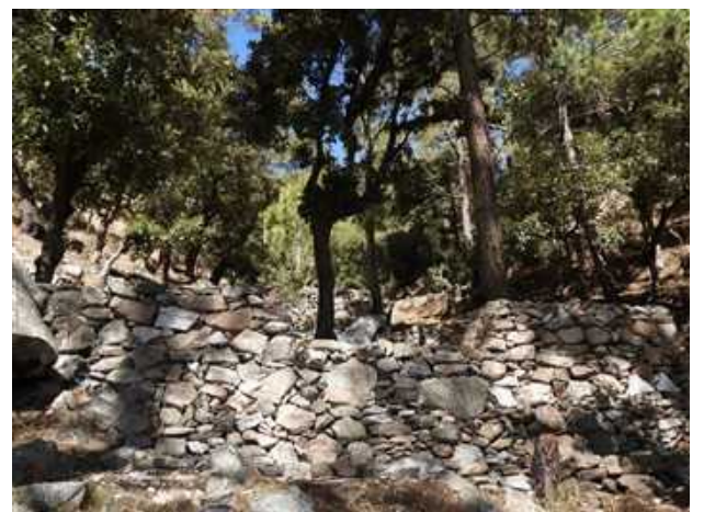
Team First, Uttarkashi Division, Dhanarigaad Range, Kumrada Nala site, Activity: Cratewire Checkdam, Latitude: 30.56423889, Longitude: 78.36522778.
