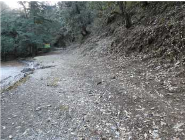
Team Fifth, Mussoorie Wildlife Sanctuary, Activity: 7 kms Walkway Construction, Latitude: 30.46808056, Longitude: 78.17787222.
