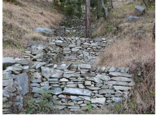
Team First, Uttarkashi Division, Nagungaad Range, Ghiyakoti site, Activity: Gully Plugging, Latitude: 30.54494722, Longitude: 78.29702778.
