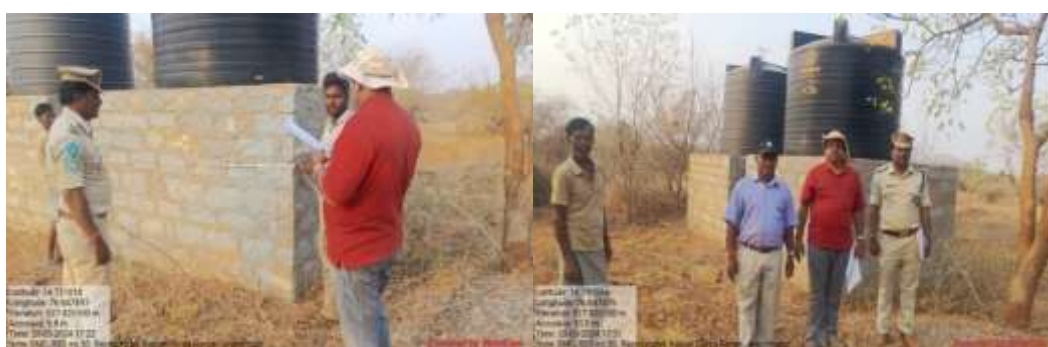
Platform for tank in Bondanakal field nursery of Rayadurg beat of Kalyandurg range
