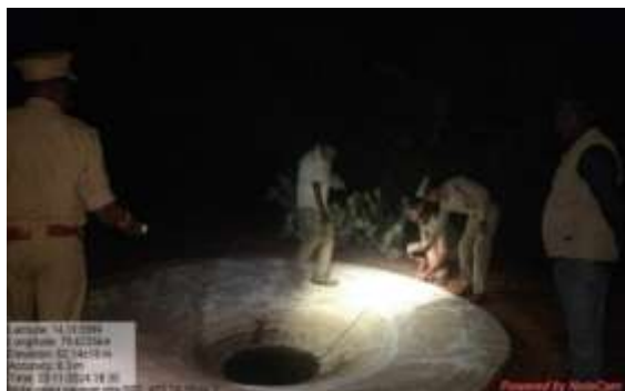
Saucer pits in Kandaleru dam area
