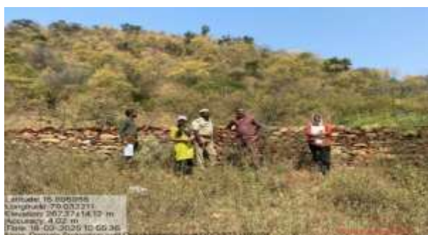
Protection wall in Dornala range
