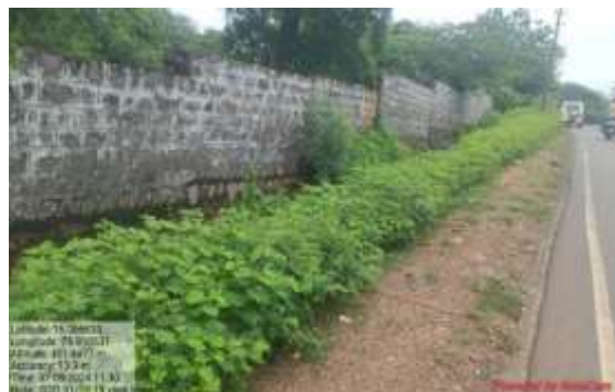
Fire lines at Sundipenta
