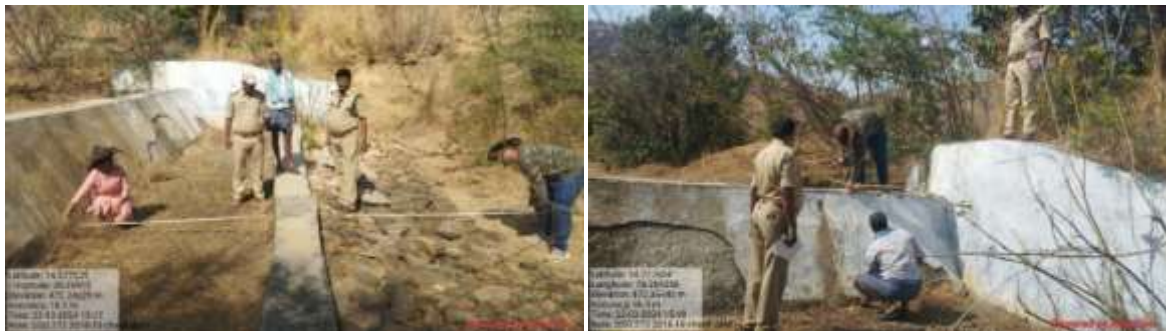
New cement check dam at Gorivikanuma RF in Talupula beat of Kurli section, Kadiri
