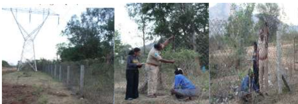
Chain-link mesh fencing around the Irala CN of Chittoor West range
