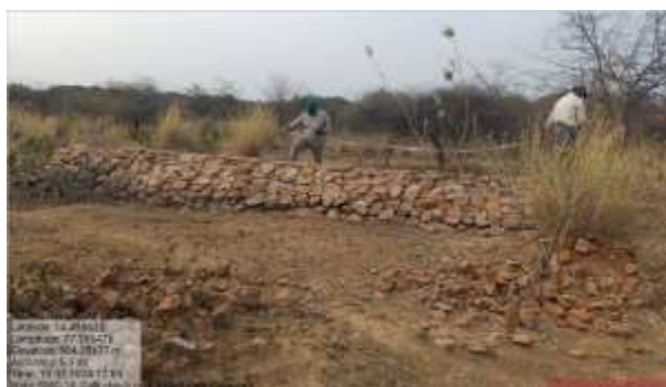
Gully checks (rock fill dams) in the CA land of Kondapalli beat
