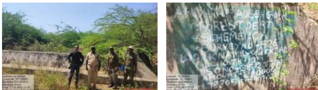
Check dam across Mekalabonda Vagu in Markapur
