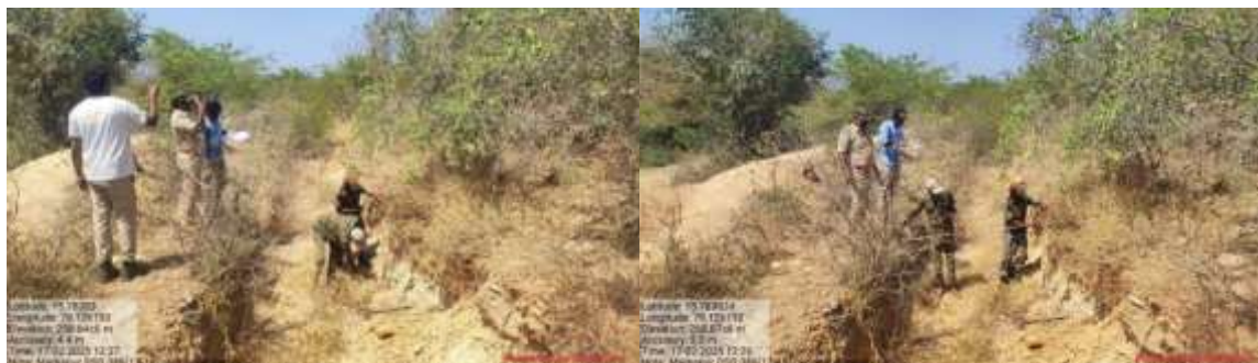
Peripheral trench around Inamakula CA land bit II in Markapur range
