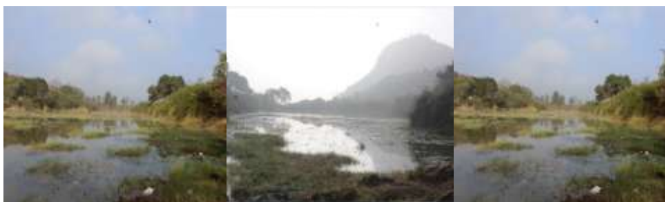
New percolation tank at Damarakunta near Betrayaswamy temple in Nadimur beat
