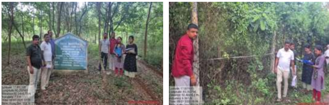
RCC Fence posts and Chain-link Fence fixing in Mudasarlova beat
