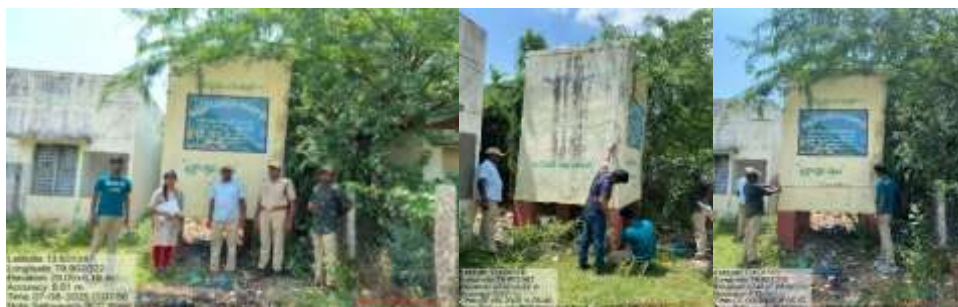
RCC water tank in Kurinjalam of Kambakam section
