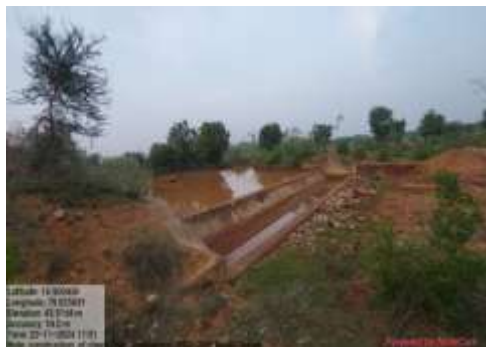
Check dam at Peddavagu
