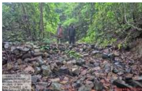
Rock fill dam at Lakkonda CA area
