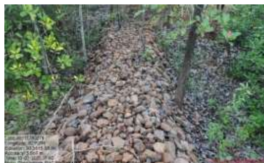
Rock fill dams in Chodavaram range
