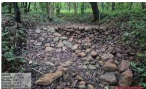
Rock fill dam at Geddada beat
