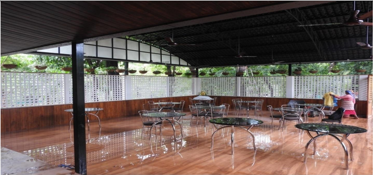
Providing work of flooring painting and steel work for the construction of the cafeteria in Bio Diversity Park, Mollem
