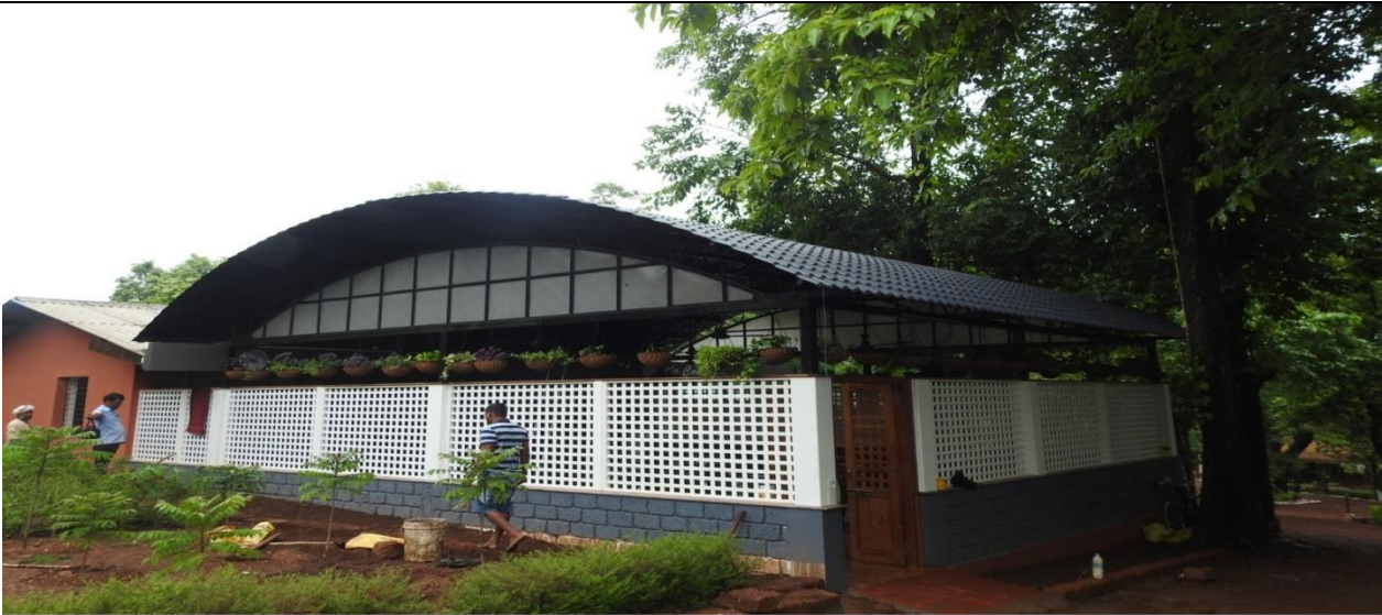
Earthwork excavation and laterite masonry for construction of outside canteen sit out in Bio Diversity Park, Mollem
