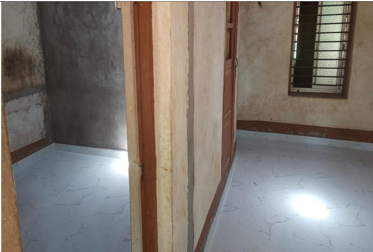
Maintenance of 'A' type quarter used as Protection Camp at Codal in Madei Wildlife Sanctuary, Madei Range
