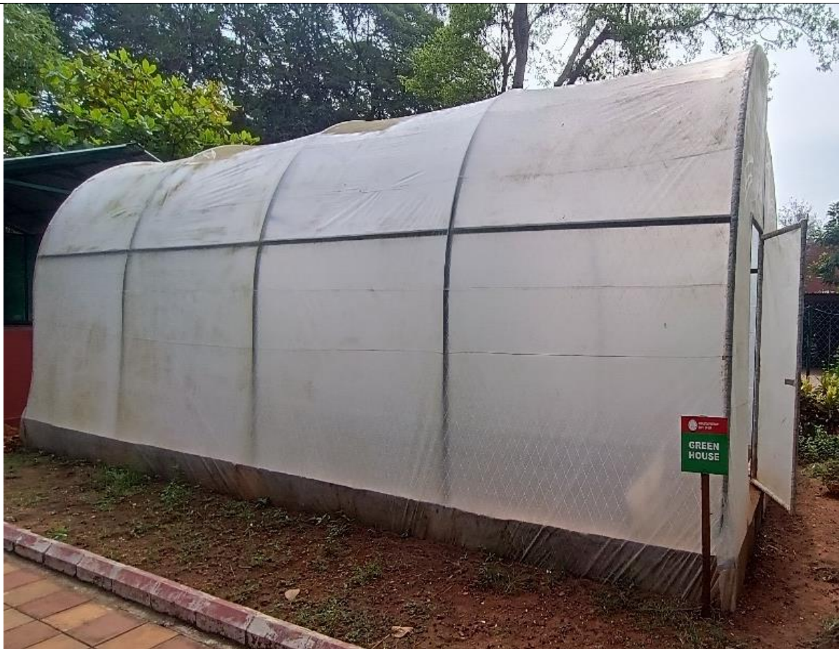
Providing Design, Supply & erection of Green House at Campal.
