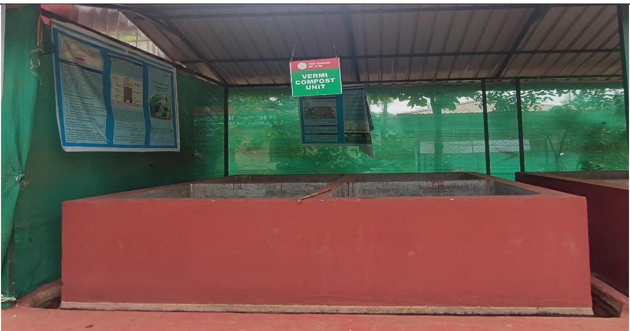
Construction of Vermi Compost unit at Campal Nursery.
