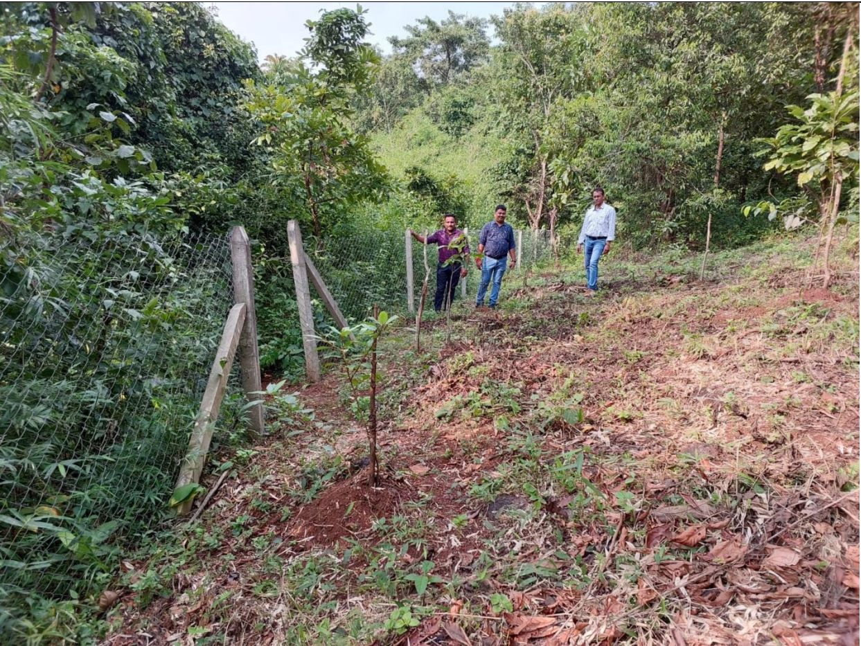
Chain Link Fencing using R.C.C Poles at 3.5mtrs intervals for 7Ha C.A. Plantation at Alorna Beat
