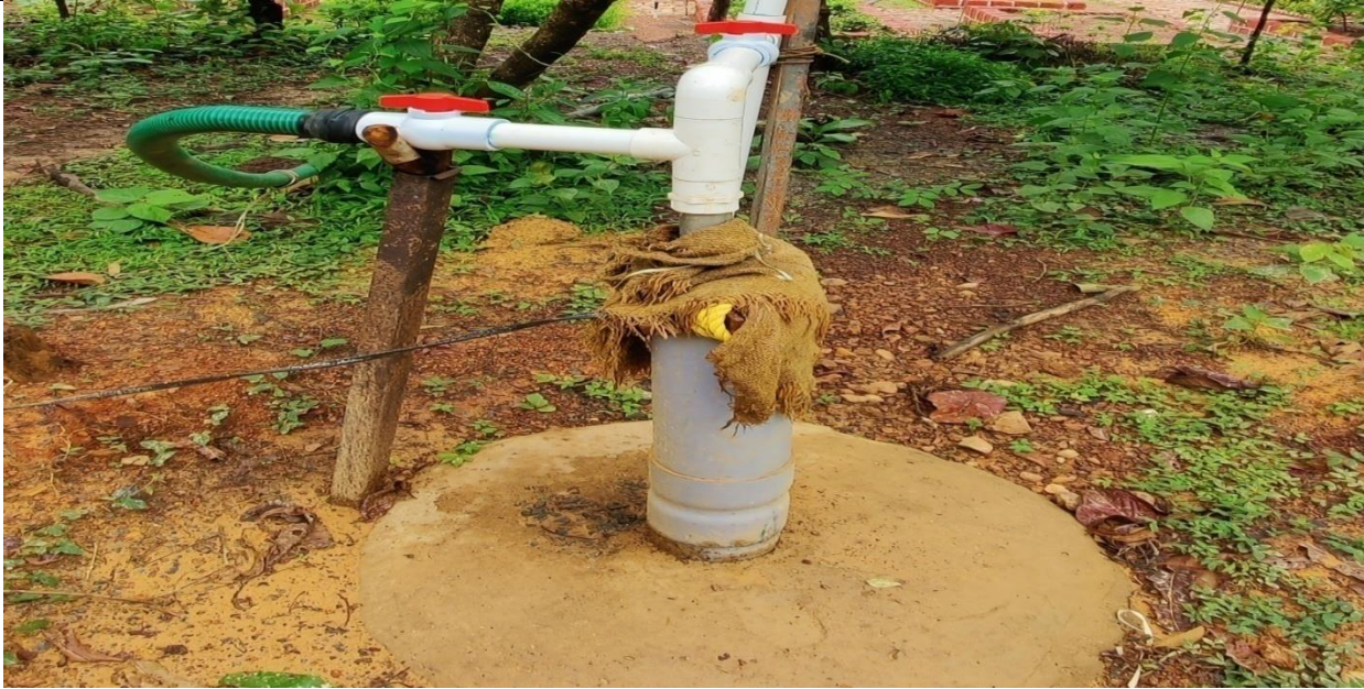
Supply and fixing of 3 HP pump for Bore well at Bio Diversity Park, Mollem
