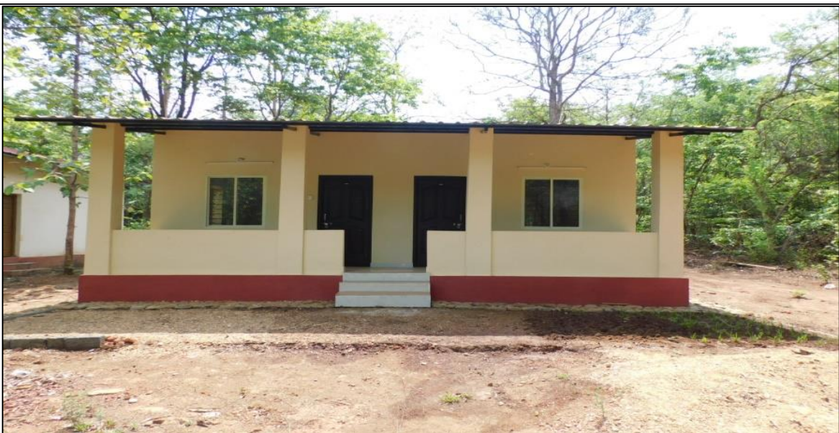
Construction of labour shed at Mollem Wildlife Range
