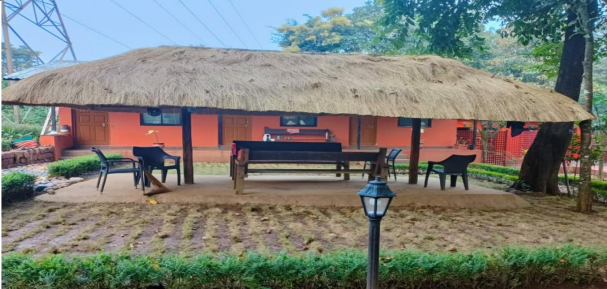
Raising of Lawn plot Max lawn grass within an area of 110 sq. mtrs. in front of the park office/labour Room/store room building at Bio Diversity Park, Mollem
