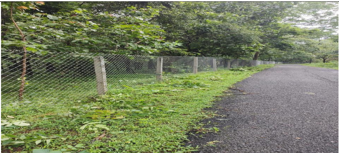
Providing Protective Chain link fencing in the plantation at Melauli Plantation
