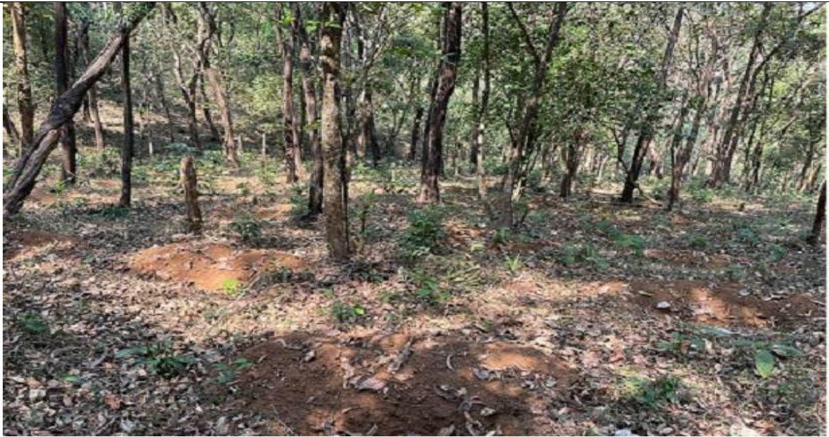
Digging of staggered contour soil trenches of size 1.00 mts. x 0.50 mts. x 0.50 mts at Gullem
