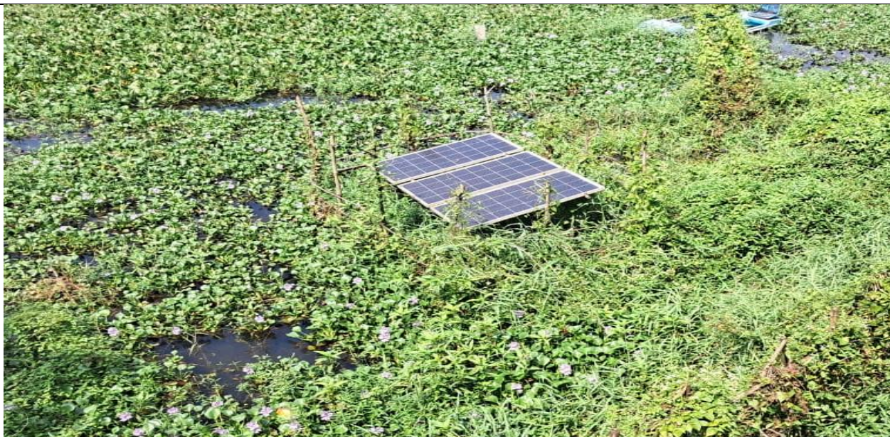
Design, installation fabrication fixing commissioning of solar off-grid system 1kv with 14 hours of backup after sunset at Carambolim patrolling.
