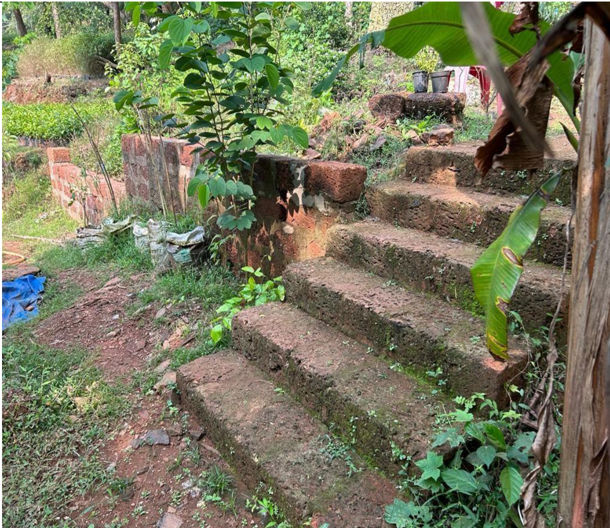
Construction of access to labour shed at Dhavali Ponda
