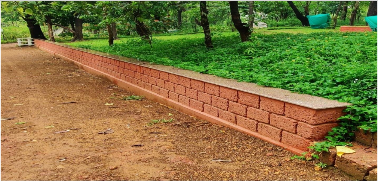
Construction of 33 meters. retaining cum parapet wall in the butterfly section of Bio Diversity Park, Mollem
