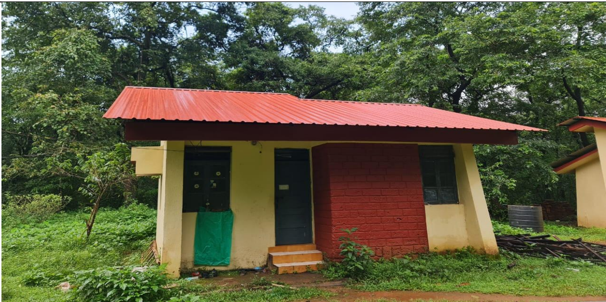
Repair of A-type quarter near Range office at Mollem Range
