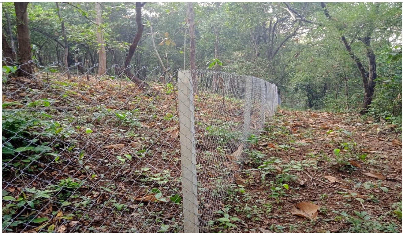
Providing Protective Chain link fencing in the plantation at Nagvem Plantation
