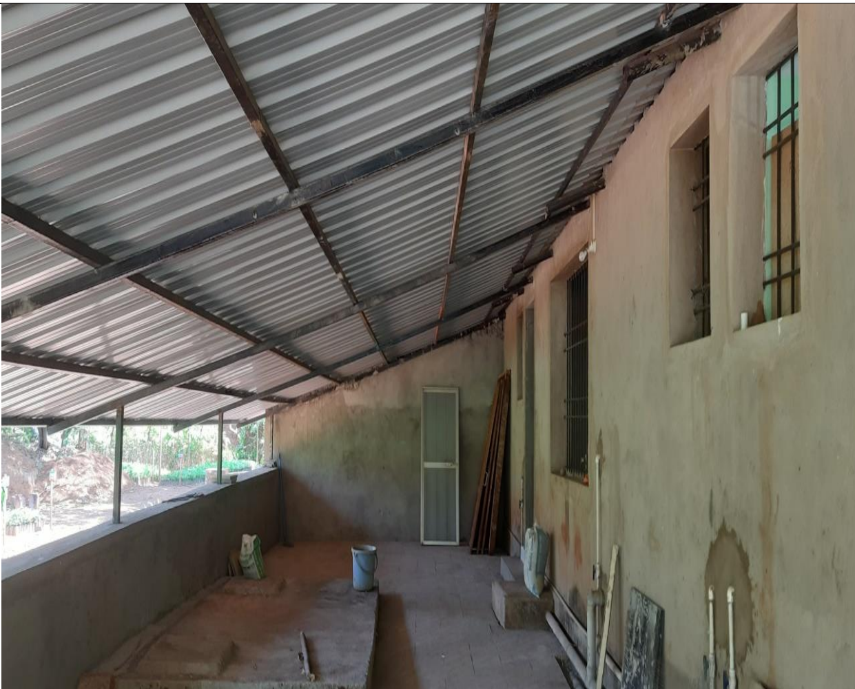
Construction of Labour Shed for Nursery at Codal Nursery in Codal Round of MWLS
