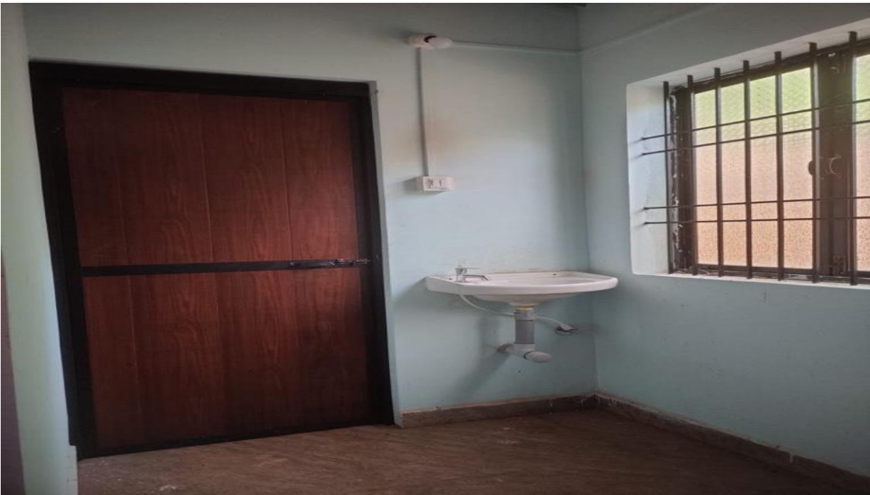
Construction of labour shed and toilet at modern nursery Dhavali
