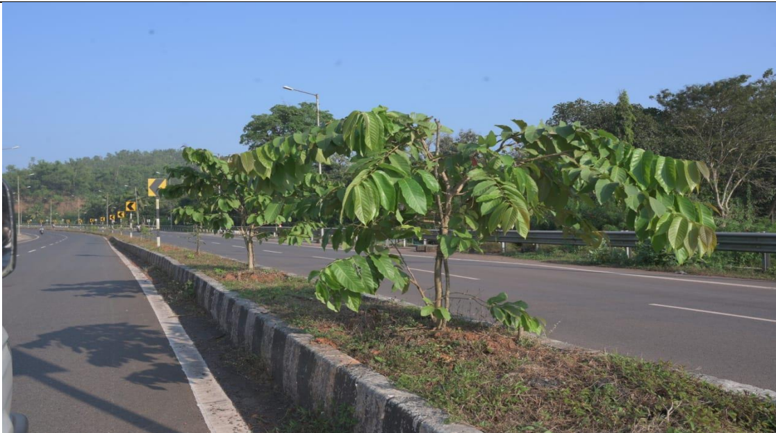
Maintenance of Road divider from R.T.O. Office to Khandepar.5 R /km
