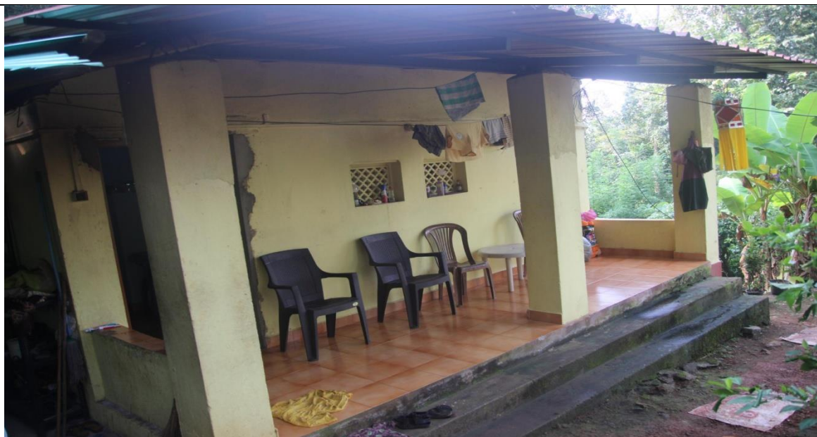
Repair of Labour shed painting and roofing at Dhavali-Ponda.
