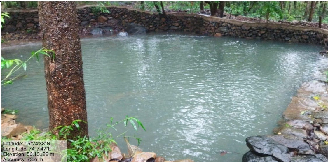
Creation of water retaining sunken pond/water hole of size 12.00mts X 8.50mts at Gurkhe Dharbandora under CAMPA.
