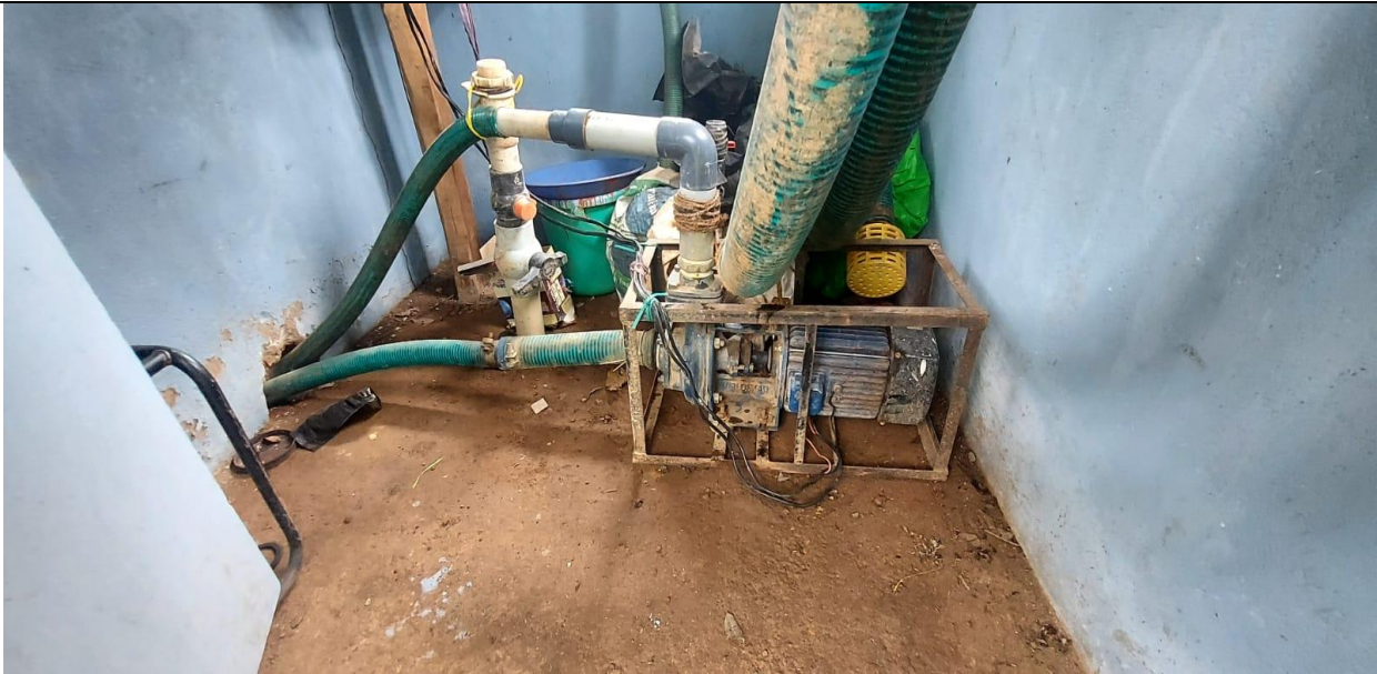
Procurement of 5 HP submersible water pump and Electrical fitting for irrigation network system at Bio Diversity Park, Mollem
