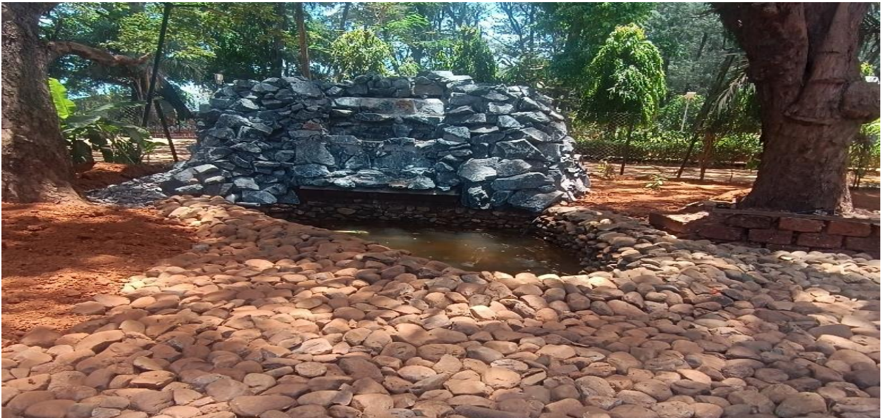
Construction of Decorative Cascade water and water pond at Campal
