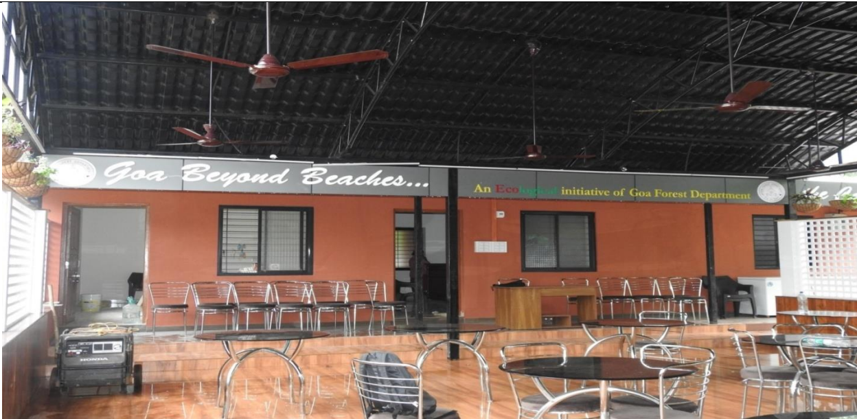
Providing work of Earthwork excavation laterite masonry plastering and construction of cafeteria at Bio Diversity Park, Mollem
