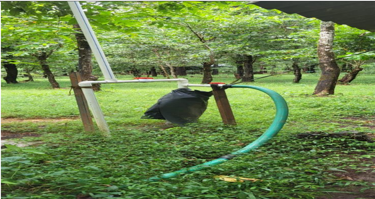
Digging of bore well in Bio Diversity Park, Mollem
