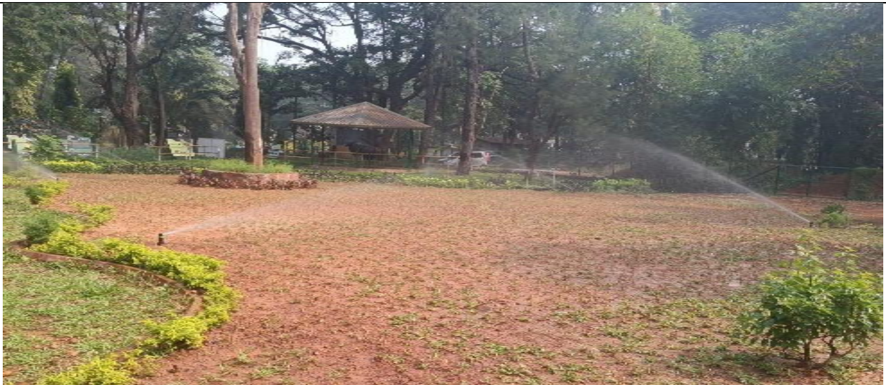
Providing UPVC pipelines setup with pump and clappet value at Nature Education Centre at Campal.
