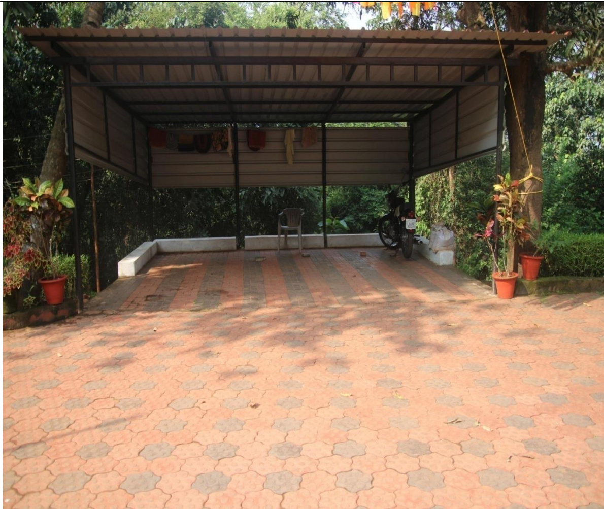
Construction of parking shed in front of Range office, Dhavali-Ponda under CAMPA
