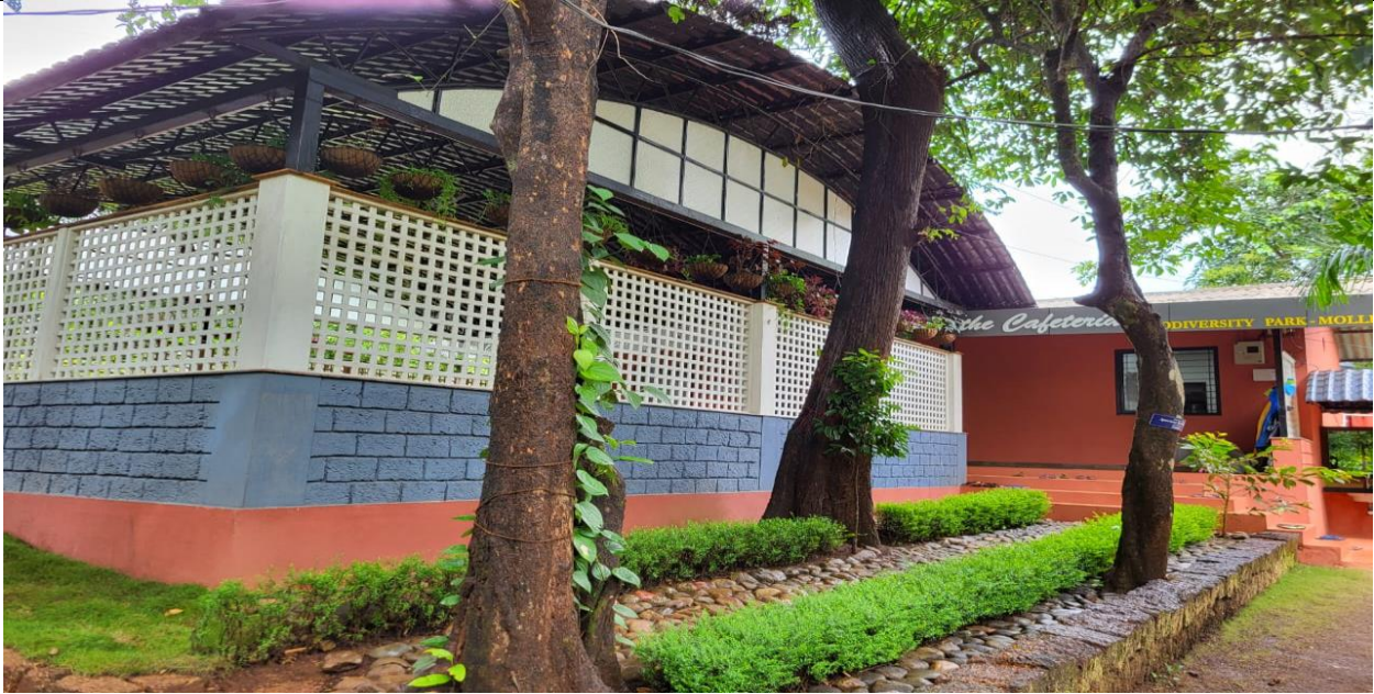
Construction of outside canteen sit out in Bio-Diversity Park, Mollem
