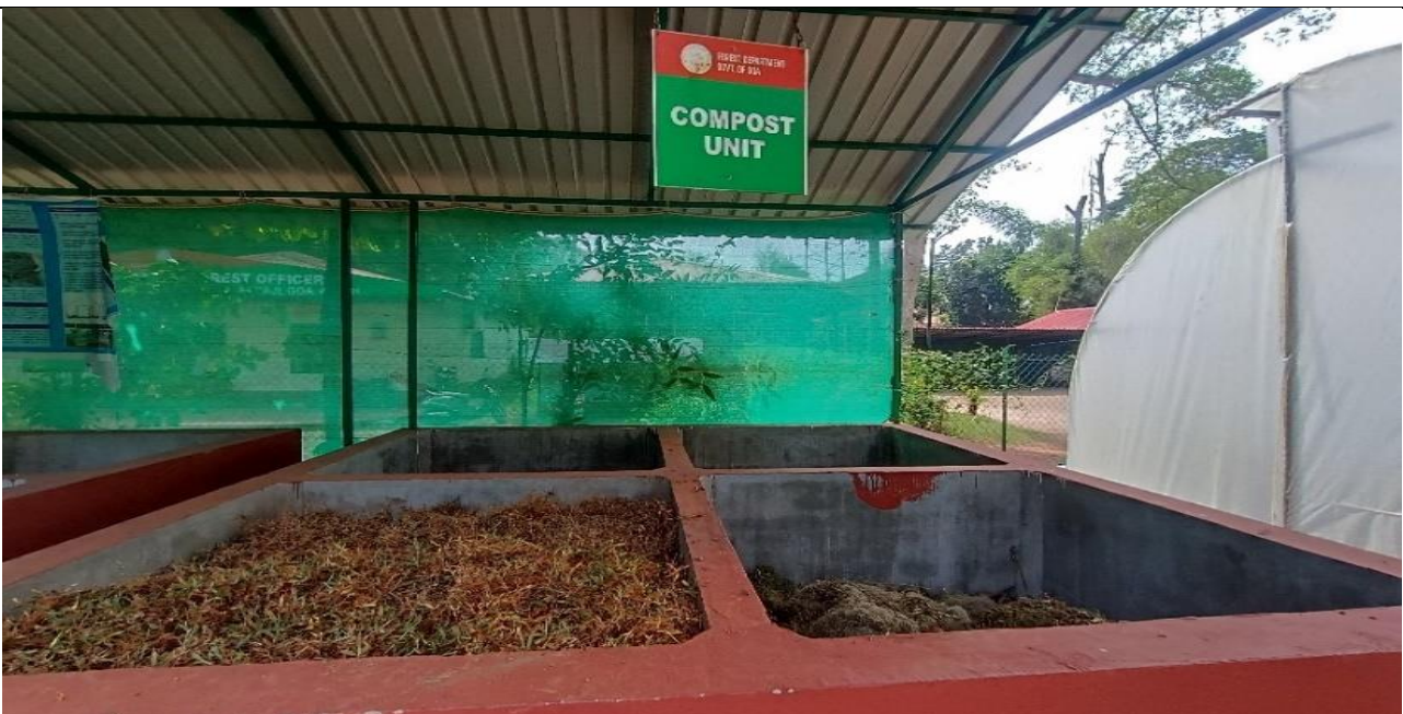
Construction of Compost unit at Campal Nursery.
