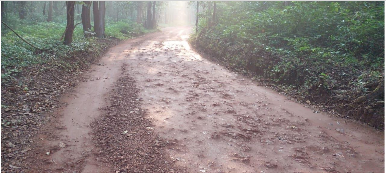
Repair and maintenance of the road from Sonaulim to Dudhsagar at Mollem Wildlife Range
