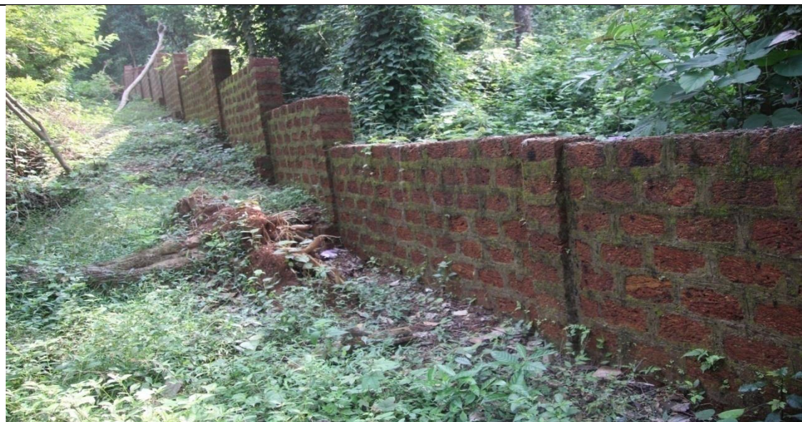
Construction of compound wall near 'B' type quarters in Forest colony Dhavali, Ponda-Goa
