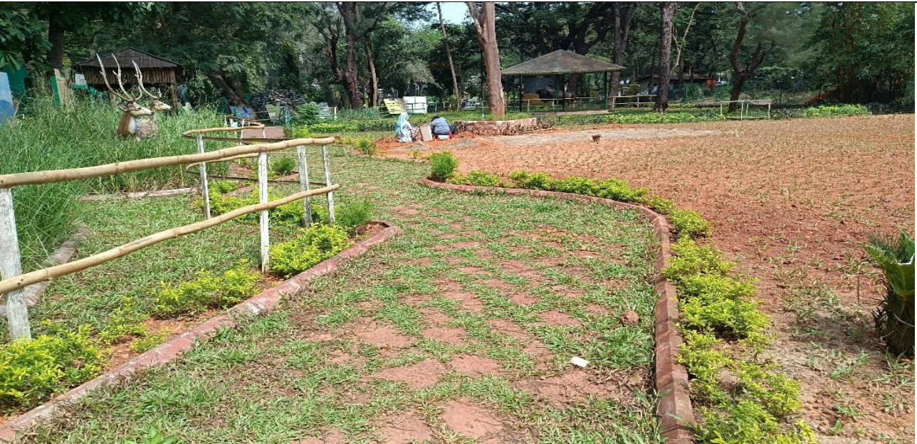
Construction of 80 mtrs pathway for open Interpretation Centre & briefing centre
