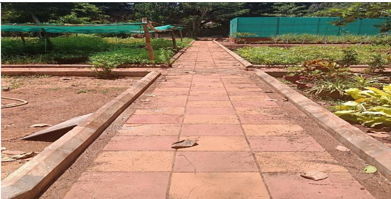
Construction of Inspection paths for Campal Nursery.
