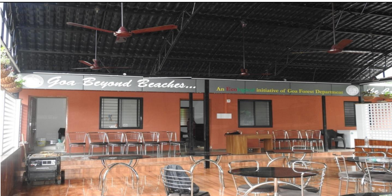
Providing fancy roofing PVC sheet to outside canteen sit out in Bio-Diversity Park, Mollem
