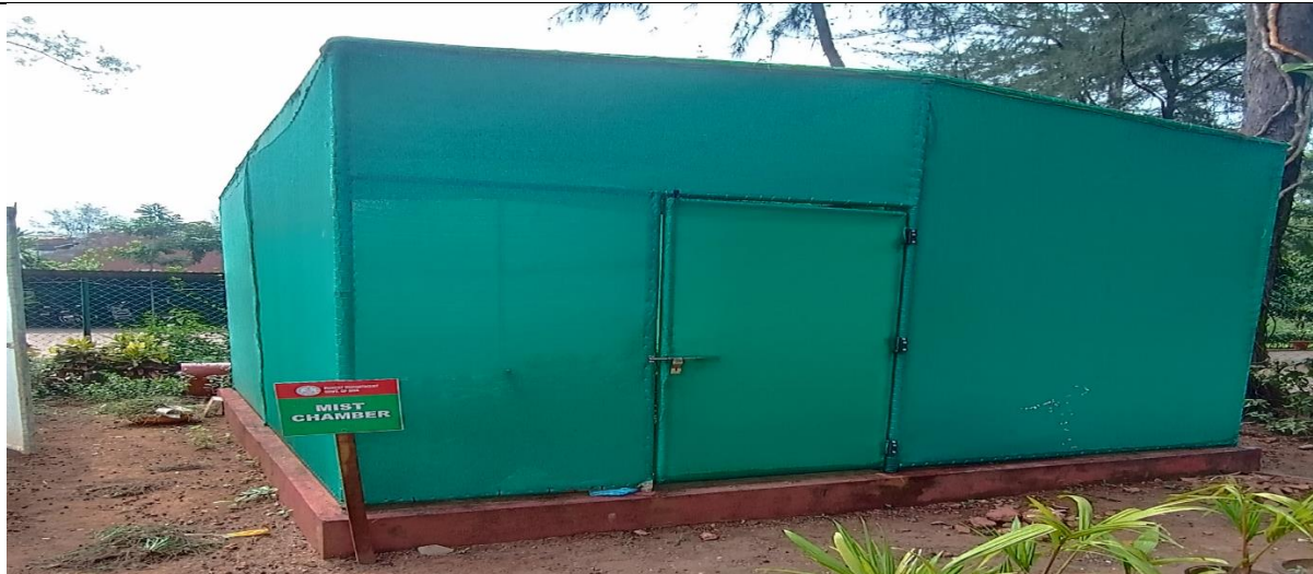
Providing Design, Supply & erection of Mist Chamber with GI Pipe structure 90% Shed Net with pump and Irrigation System
