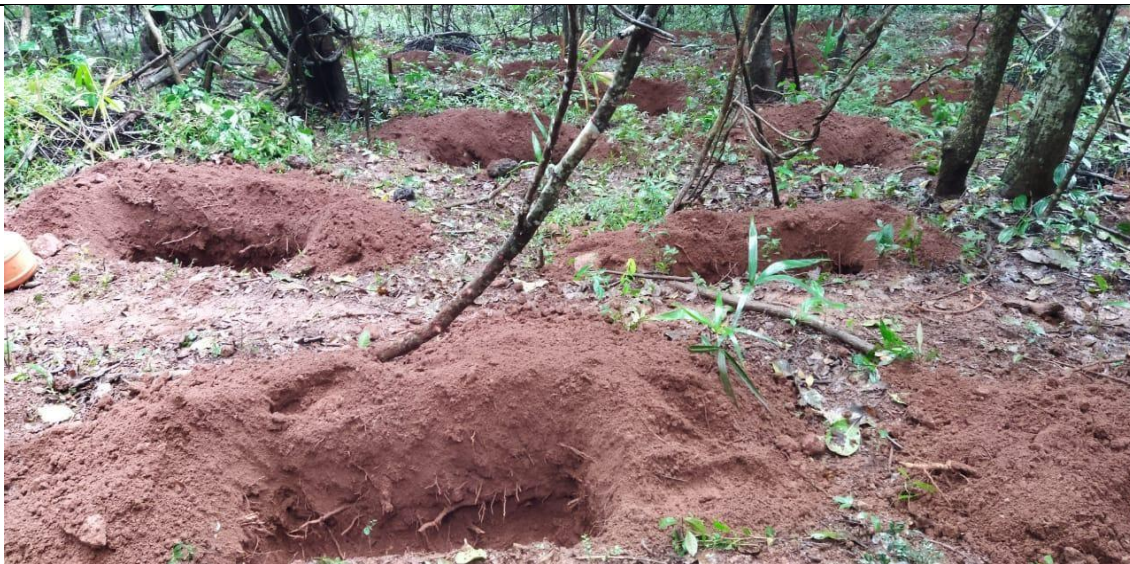
Digging of staggered contour soil trenches of size 1.00mts x 0.50mts x 0.50mts at Ganjem under CAMPA.
