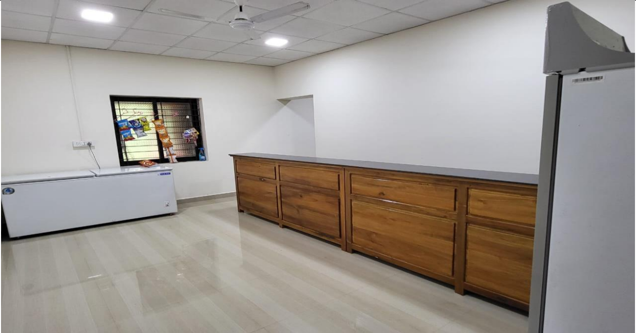
Providing work of laterite and PVC false ceiling of internal Room of Cafeteria in Bio Diversity Park, Mollem
