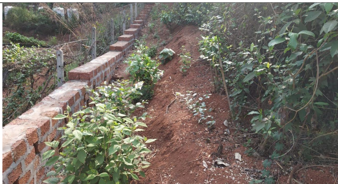
Construction of retaining wall 37.00mts near Range office under CAMPA.
