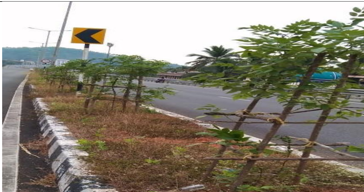
Maintenance of Road divider from Farmagudi to Dhavli Bypass Road.(1st year) 4 R/Km
