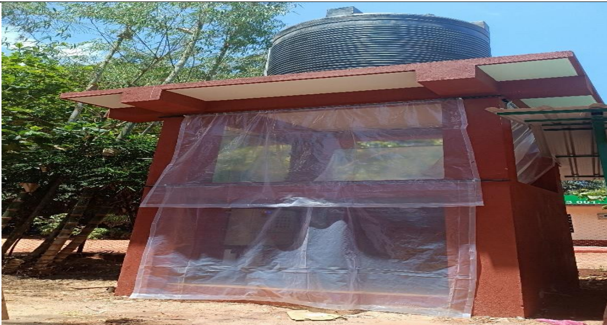
Construction of Pedestrian platform for Water Tank at Campal Nursery.
