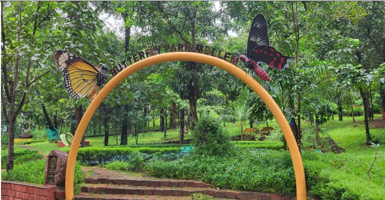
Design casting construction and installation of mural and butterfly shape on already casted entry gate of Butterfly Park at Bio Diversity Park, Mollem.
