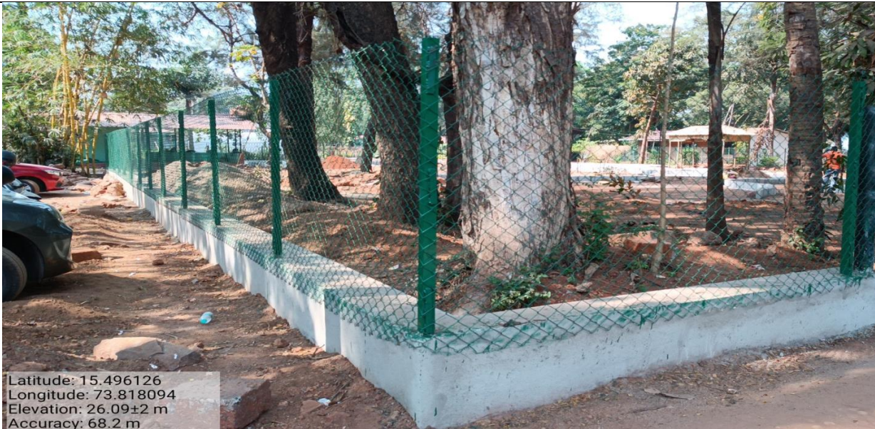
Construction of Chainlink fencing for extending area at Open Interpretation Centre at Campal Nursery.
