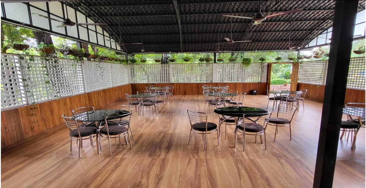
Providing flooring work of cafeteria in Bio Diversity Park, Mollem
