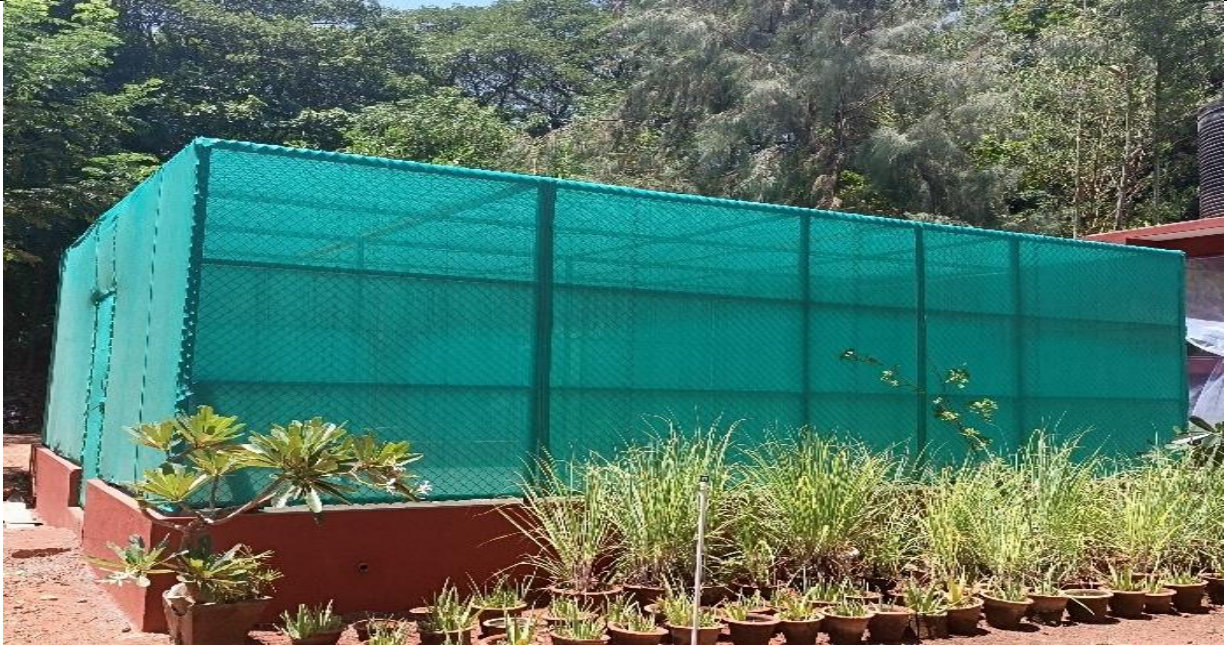
Construction of New Green net shed at Campal Nursery, Range.
