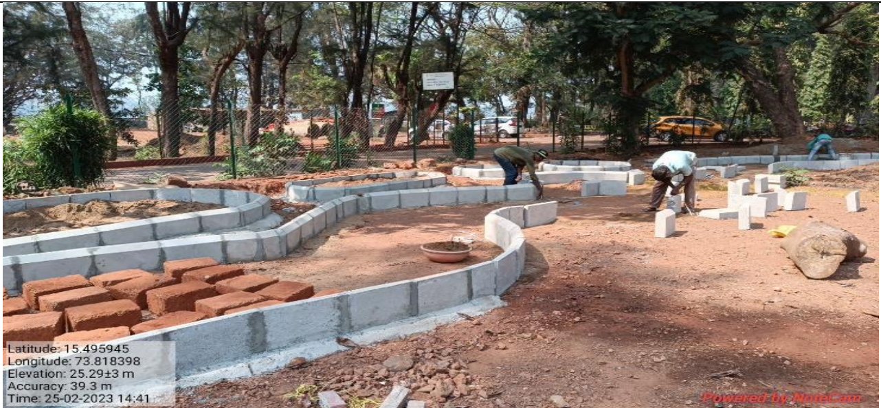
Construction of 3mtrs Diameter Circular platform with kerb stones at Cam for open interpretation Centre & briefing centre.
