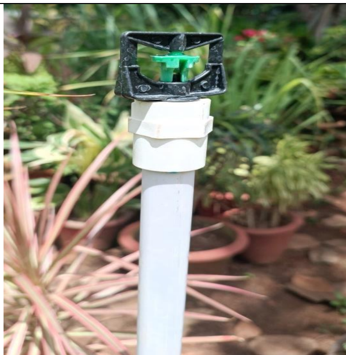
Providing Installation of Micro Sprinkler with pump at Campal Nursery
