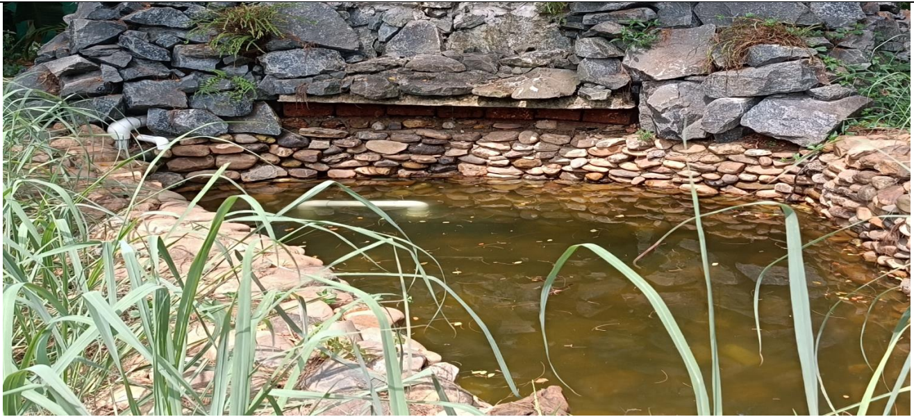
Providing Installation of Irrigation System along with filter pump with suitable Nozzle for water Cascade at Nature Education Centre at Campal
