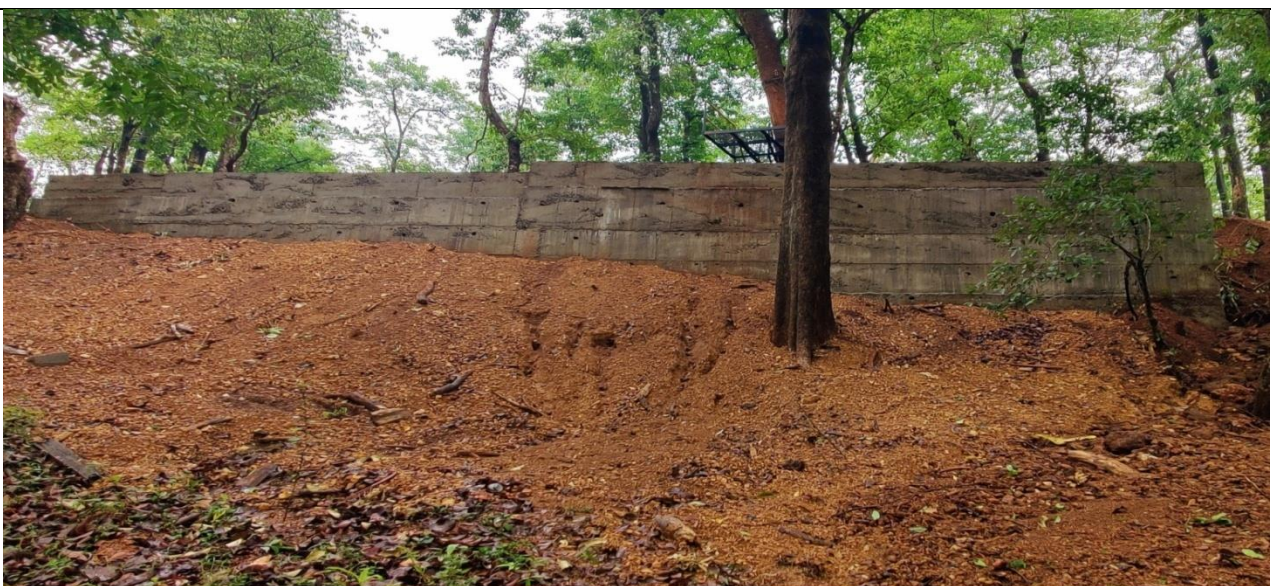
Construction of retaining wall near Amphi theatre in Bio-Diversity Park, Mollem
