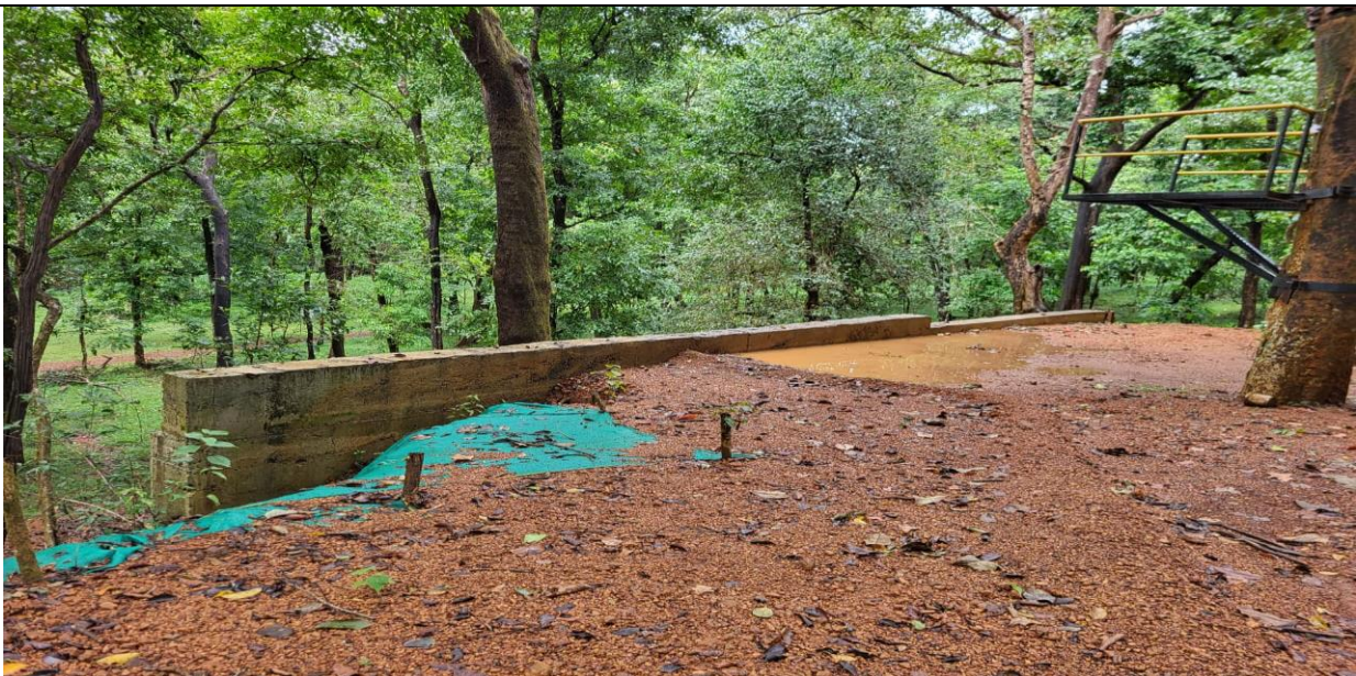
Construction of retaining wall near Zipline in Bio Diversity Park, Mollem.
