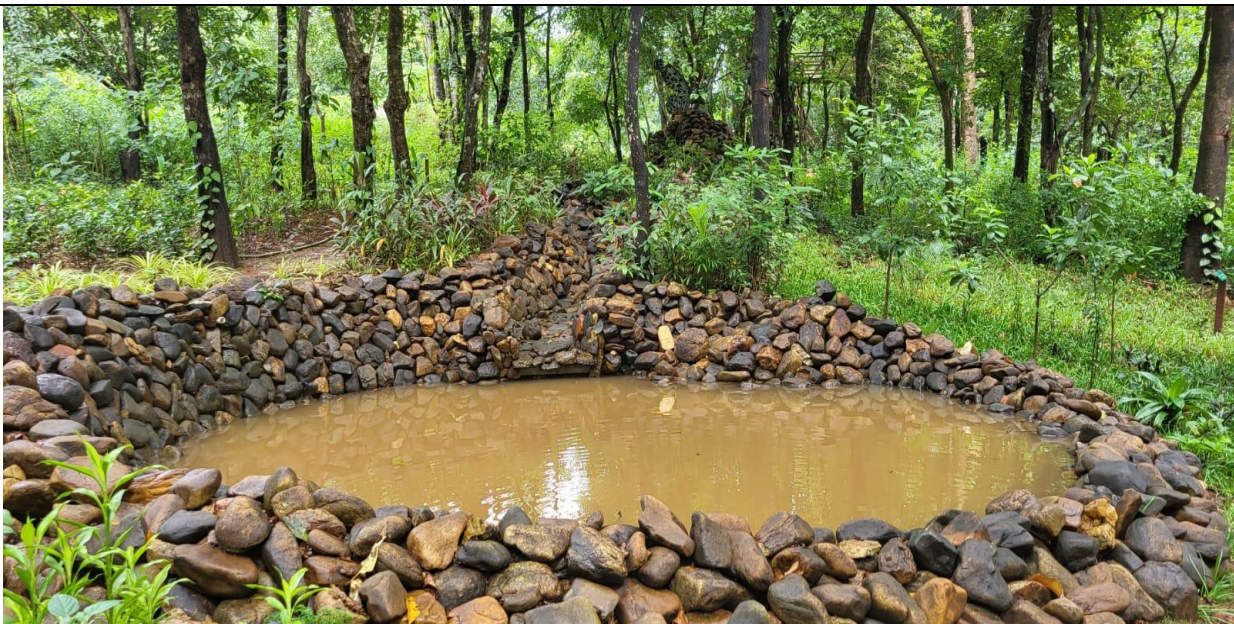
Construction of water pond and cutter in Bio Diversity Park, Mollem
