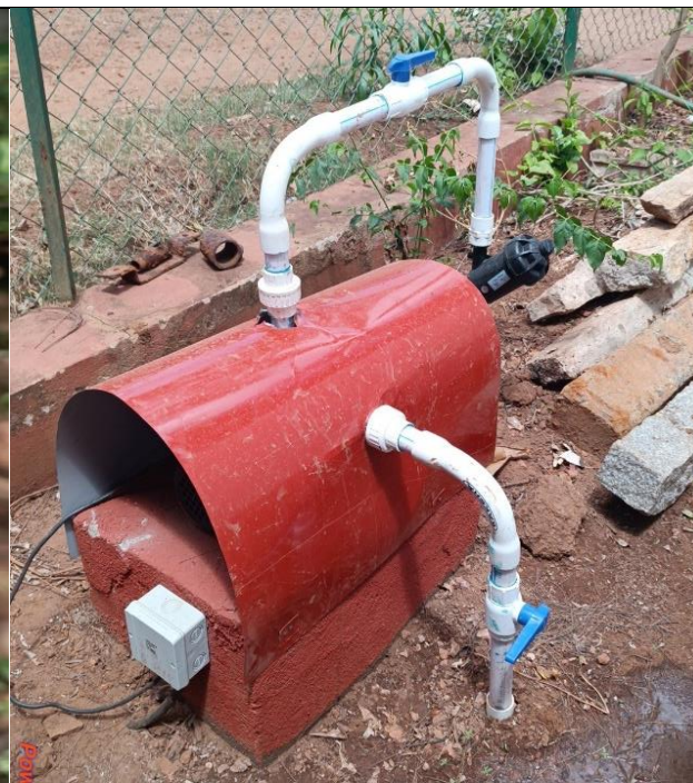
Providing Installation of Micro Sprinkler with pump at Campal Nursery
