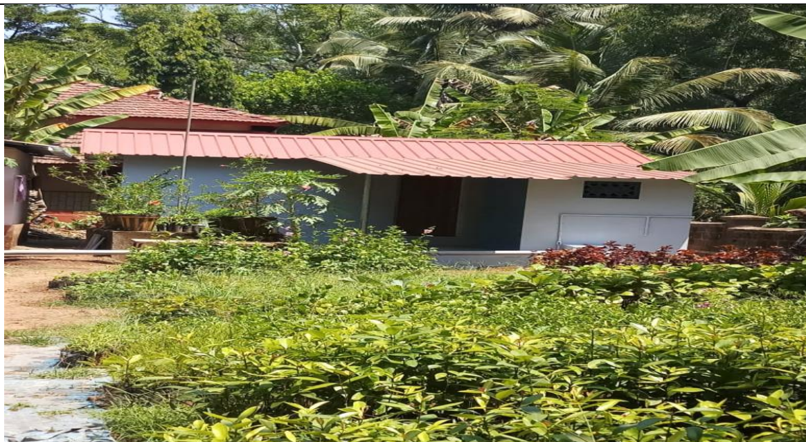
Construction of Labour shed behind Range Forest Office at Quepem
