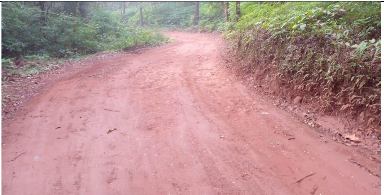
Repair and maintenance of road from Collem entry gate to Bhindifator and Bhindifator to Shiregal at Mollem Wildlife Range
