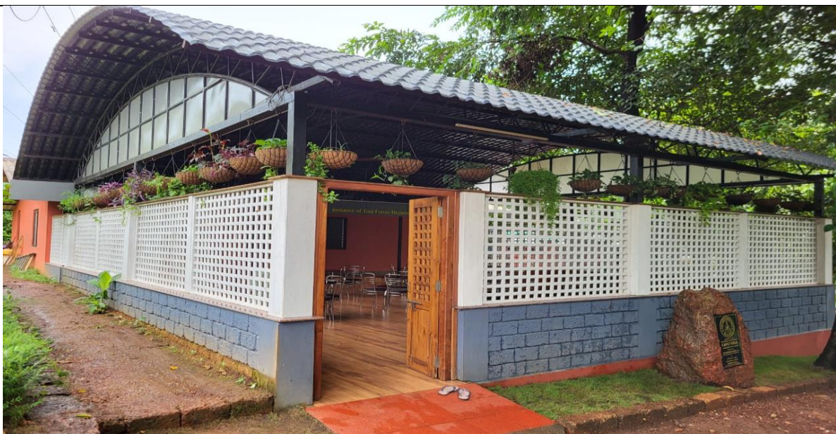
Providing Steelwork for roofing & woodwork for construction of outside canteen sit-out in Bio-Diversity Park in Mollem village
