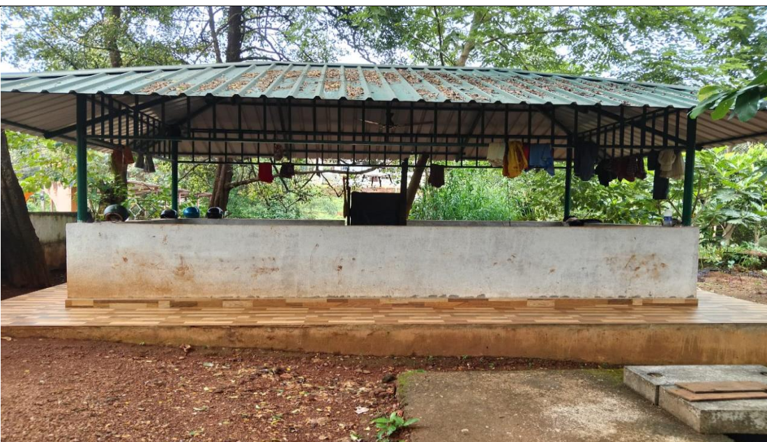
Construction of labour shed at Netaji Subhas Chandra Bose Gram Upvan, Sankhalim
