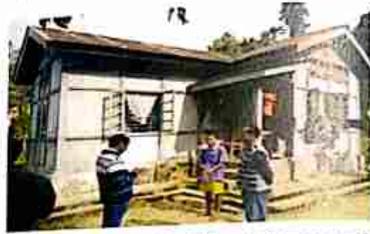
Photo-40b. SPT-I building at Namsangmukh
