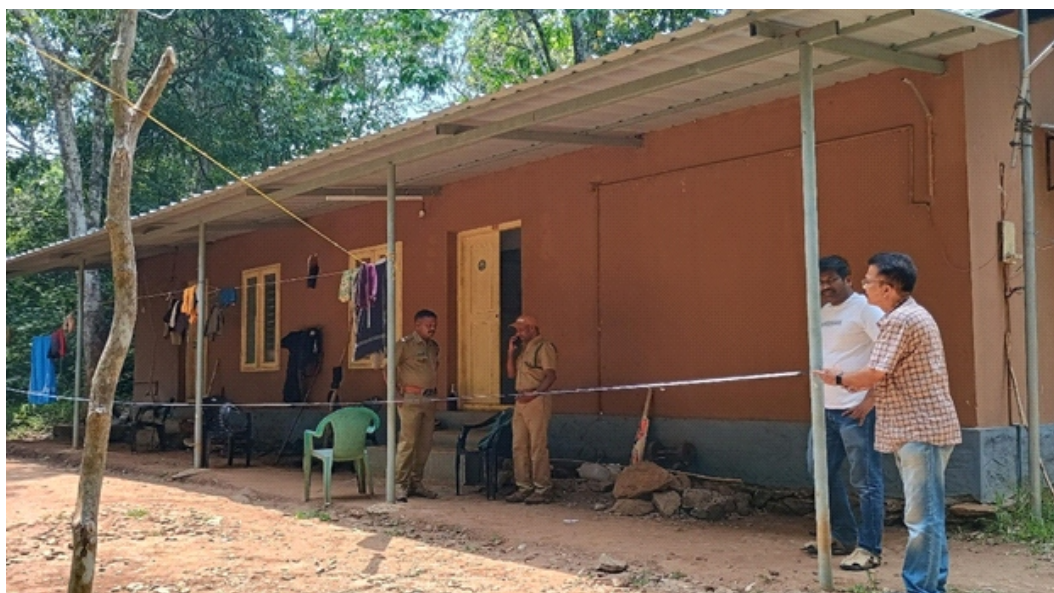
Inspection of camp shed at Vallakadavu/ PTR East
