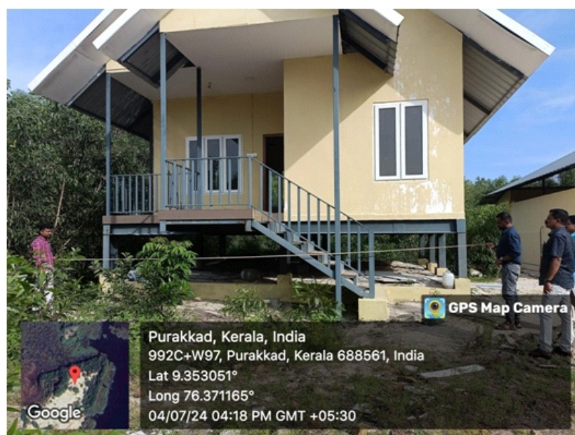
Semi-permanent eco-friendly Office room for District Permanent Nursery at Purakkad
