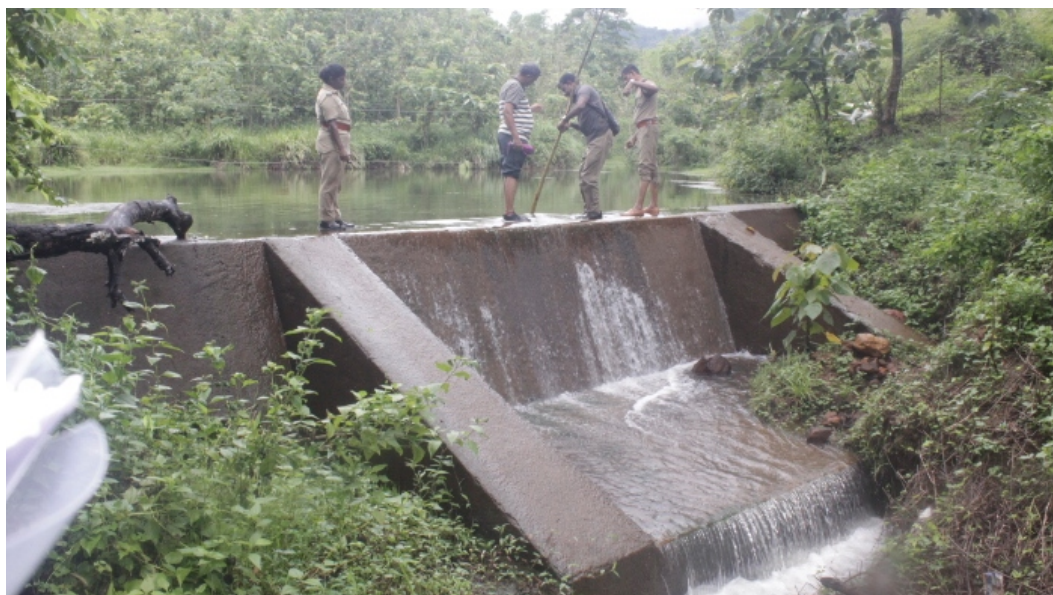
Desilting of Check dam at Achenkovil
