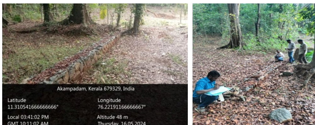
Inspection of the gully plugged at Pokkode, Edavanna range, Nilambur division
