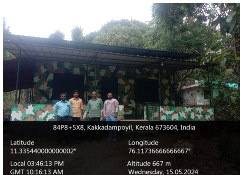
Inspection of camp shed maintenance in Nilambur range
