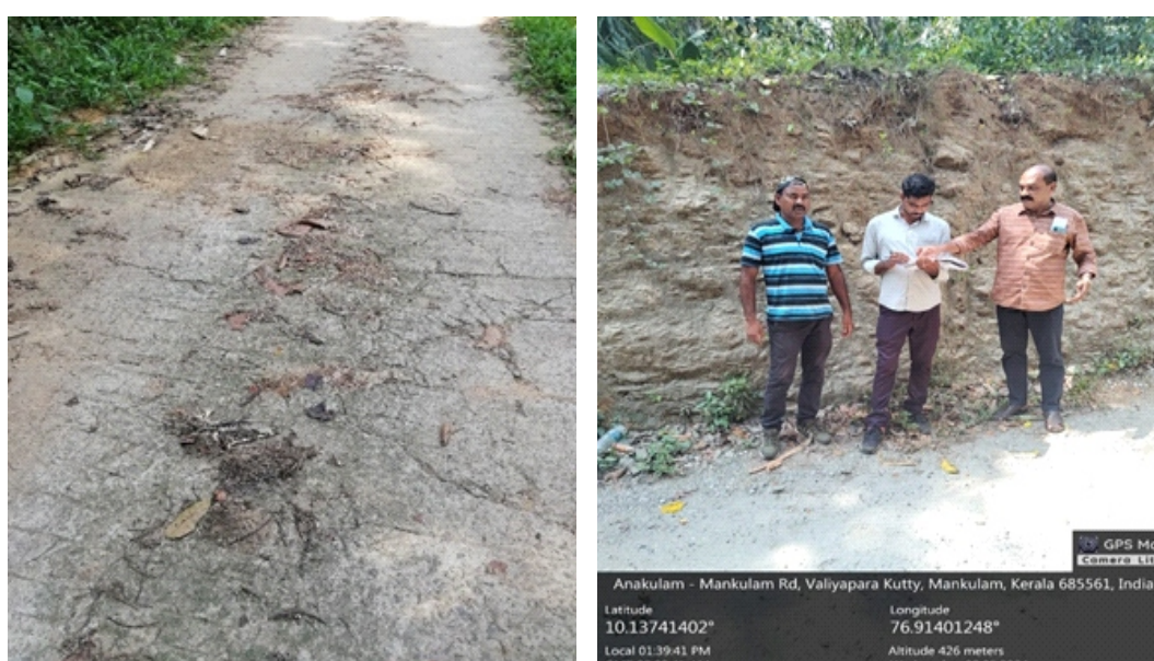
Inspecting the maintenance work of forest road in Munnar division
