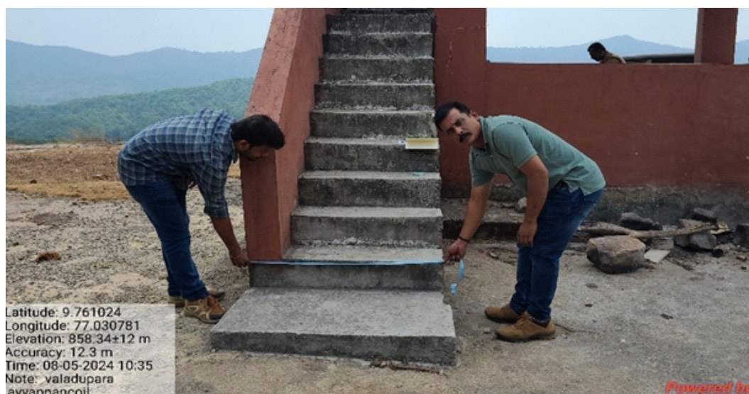
Construction of staircase for camp shed at Valadupara, Ayyappancoil, Kottayam
