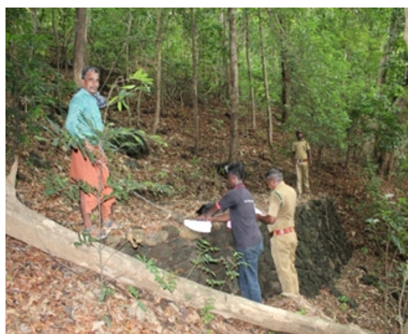
Gully plugging at Elival 1959 TP at Olavakkode range, Palakkad division
