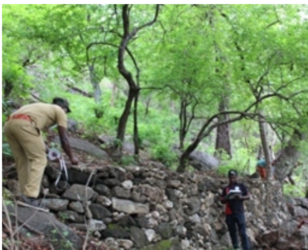
Gully plugging at Elival 1965 TP at Olavakkode range, Palakkad division
