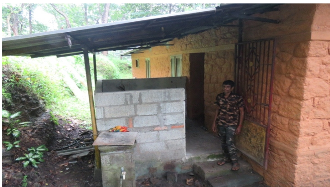
Karakladu Anti Poaching CampShed, Peppara - construction of kitchen and extension of the campshed
