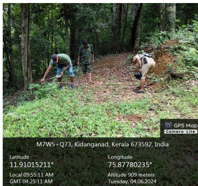
Maintenance of trek path in Aralam division
