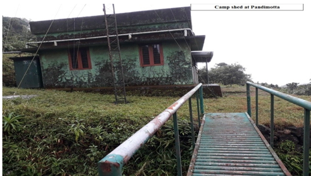
Campshed maintenance at Pandimotta, Eattapadappu range in Shendurney
