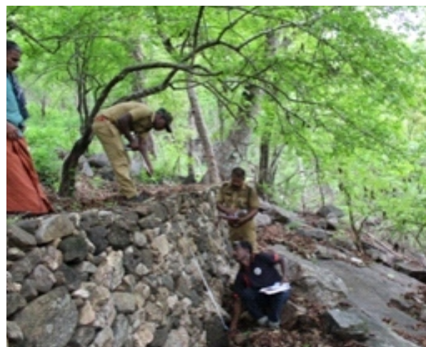
Gully plugging at Elival 1965 TP at Olavakkode range, Palakkad division
