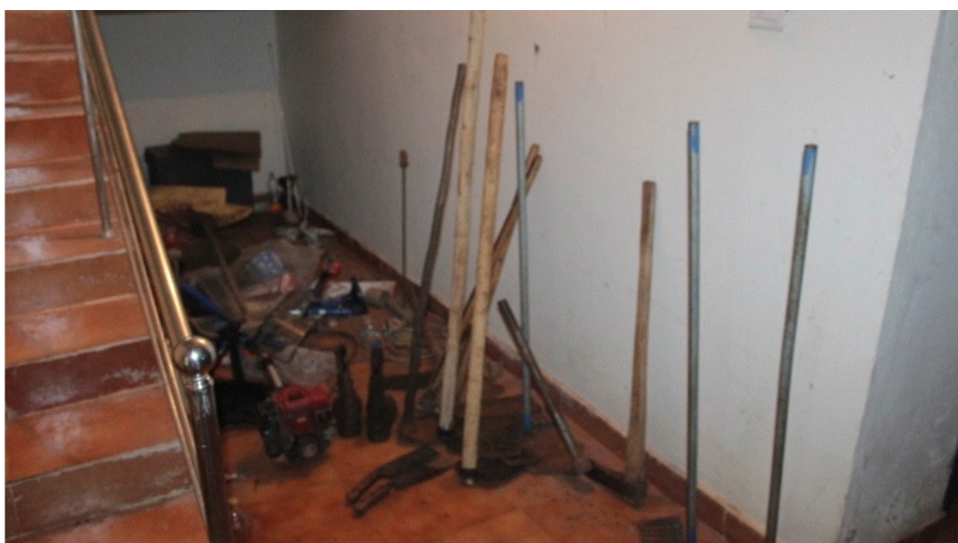
Fire fighting equipments at Konni
