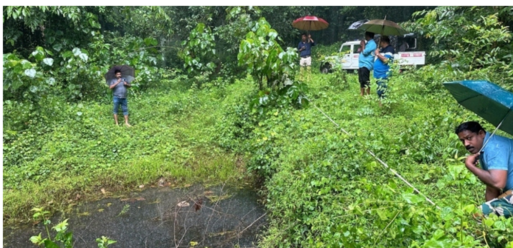
Desilting water hole at Mahagony Check dam, Anachatthapara Water hole, Idukki section
