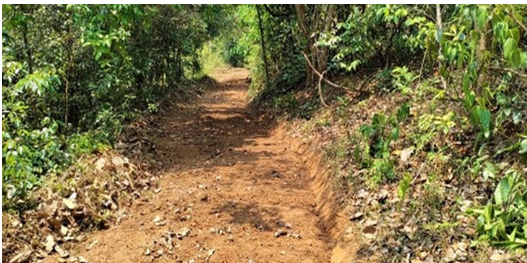
Maintenance of trek path at Kalamkunnu
