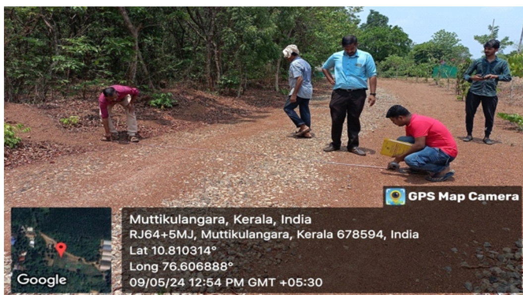
Construction of road facilities in DPN nursery, Vallikode, Palakkad
