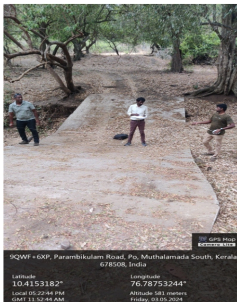
Maintenance of concrete chappath build across Thekkali river near Koochimudi APC
