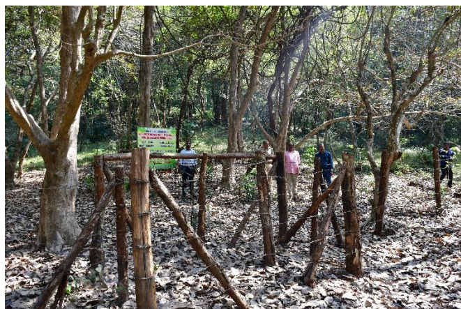
Work of fencing with Barbed wire using wooden Poles at Ganjem
