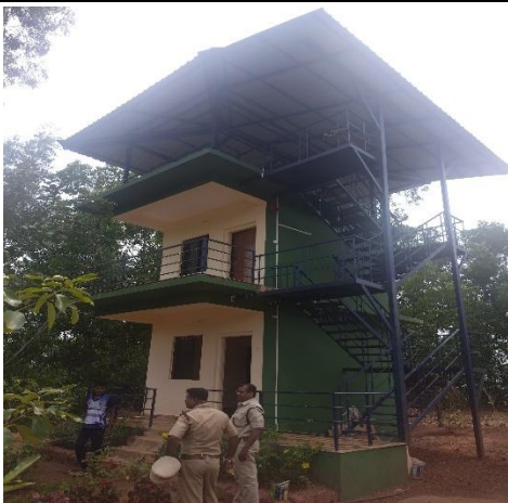
Construction of watch tower at Portem beat
