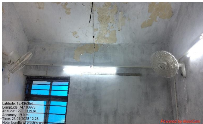
Repairing and Extension of Electrification of RFO Quarter
