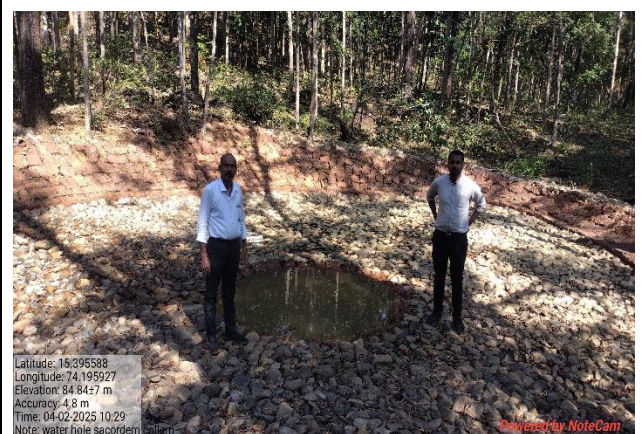
Water retaining structure at Sacorda
