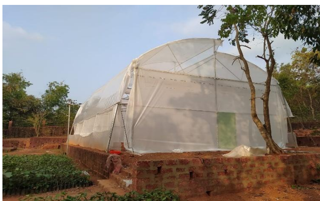
Construction of Polyhouse at Pal Usgao Nursery
