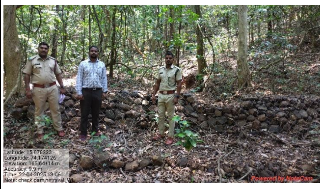
Construction of Gabion check dam at Netravali beat
