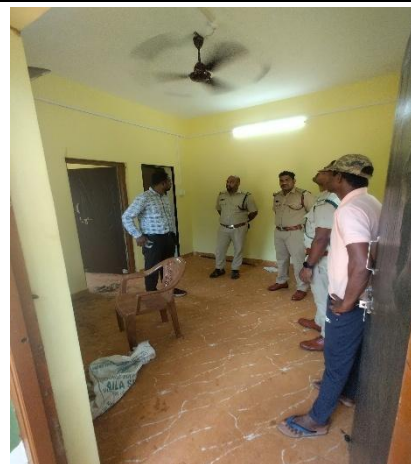
Renovation of A type quarters
