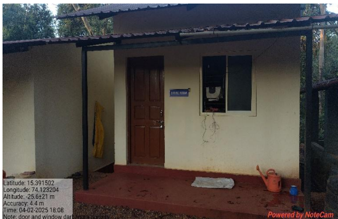
Physical verification of doors and windows for existing store room in Dharbandora Nursery
