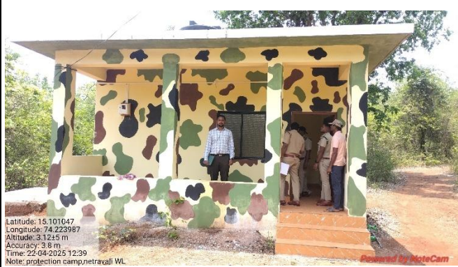
Construction of Protection camp at Netravali beat
