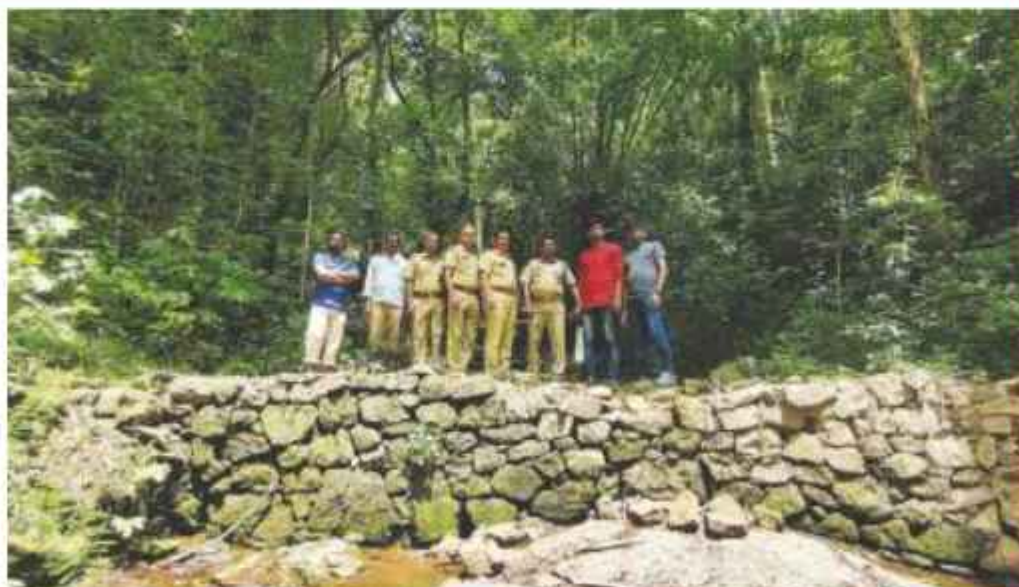
Gully Plug at Ayyappancoil
