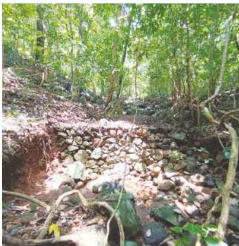
Gully Plugging at Kattikuzhy
