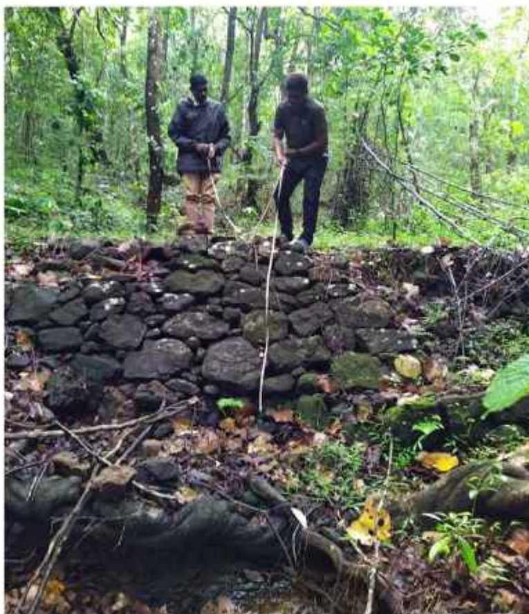
Gully Plugging at Idukki WLS
