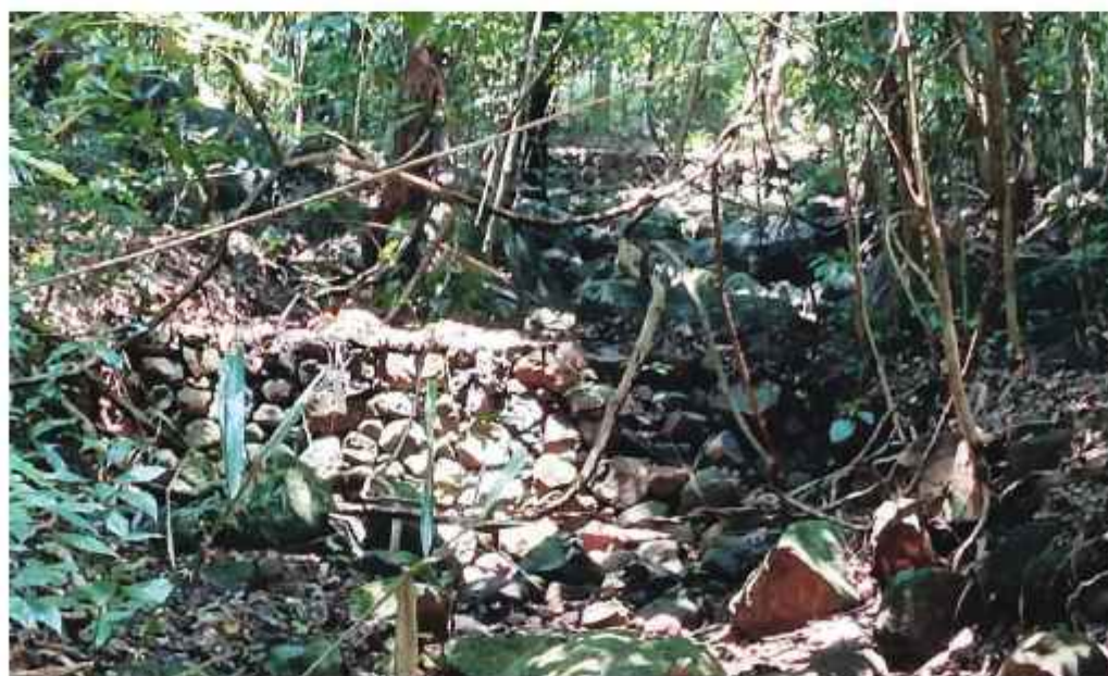
Gully plugging at Kattikuzhi
