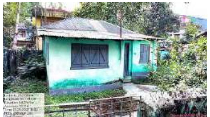
Jalpaiguri Division: Maintenance/renovation of staff quarter
