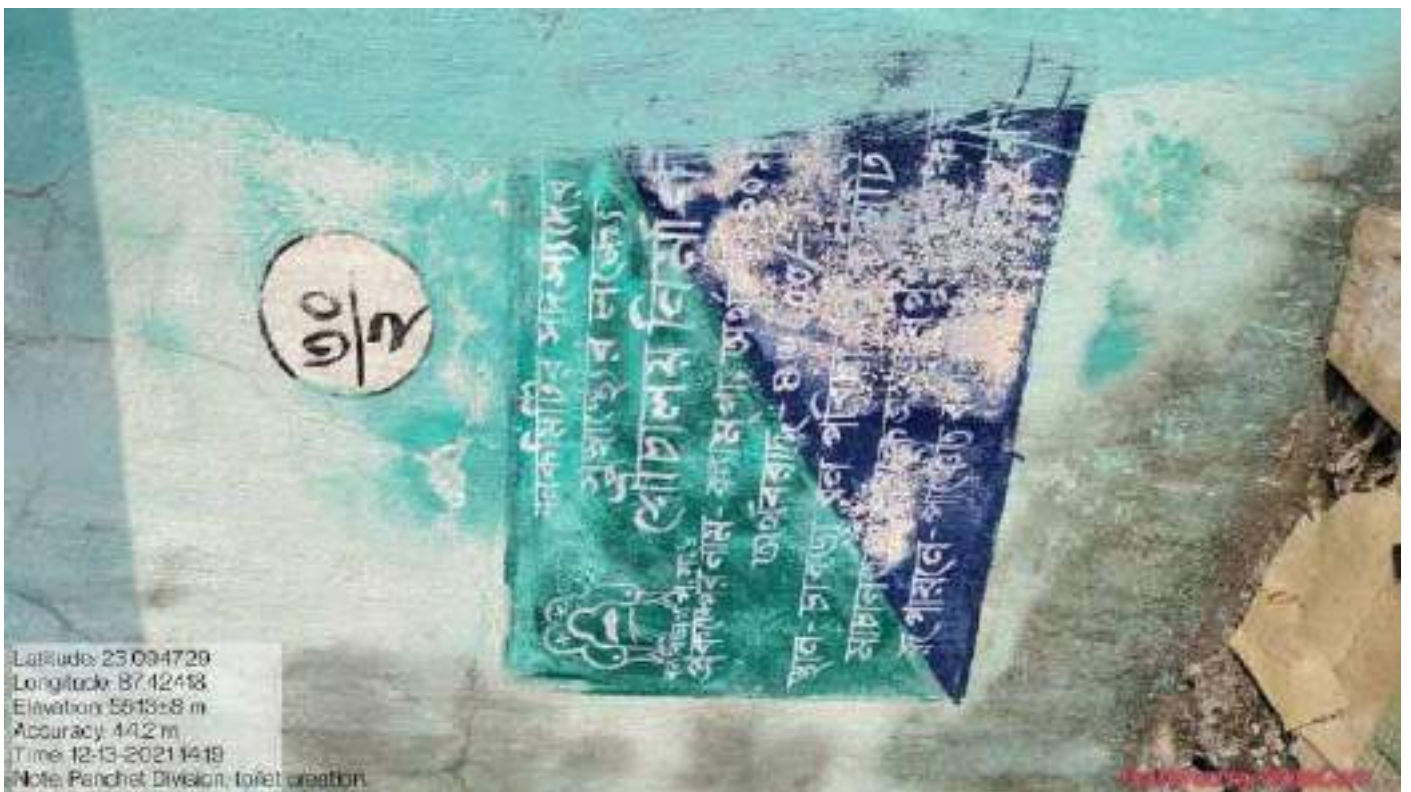
Panchet Division: Construction of JFMC toilet
