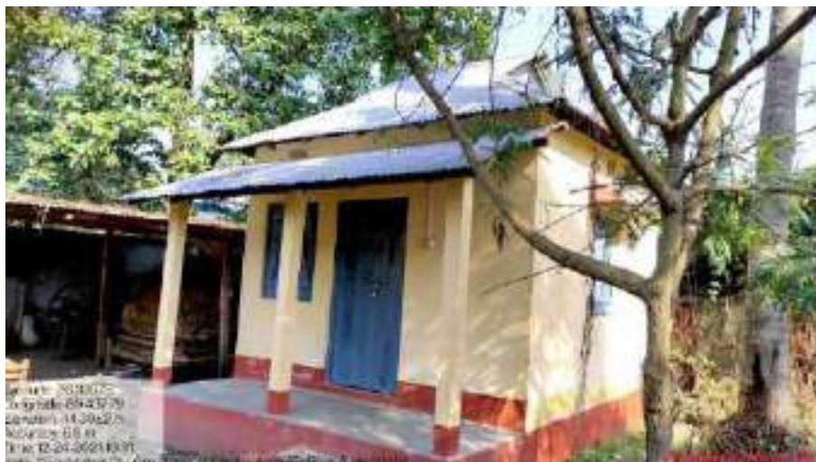
Cooch Behar Division: Maintenance of staff quarter
