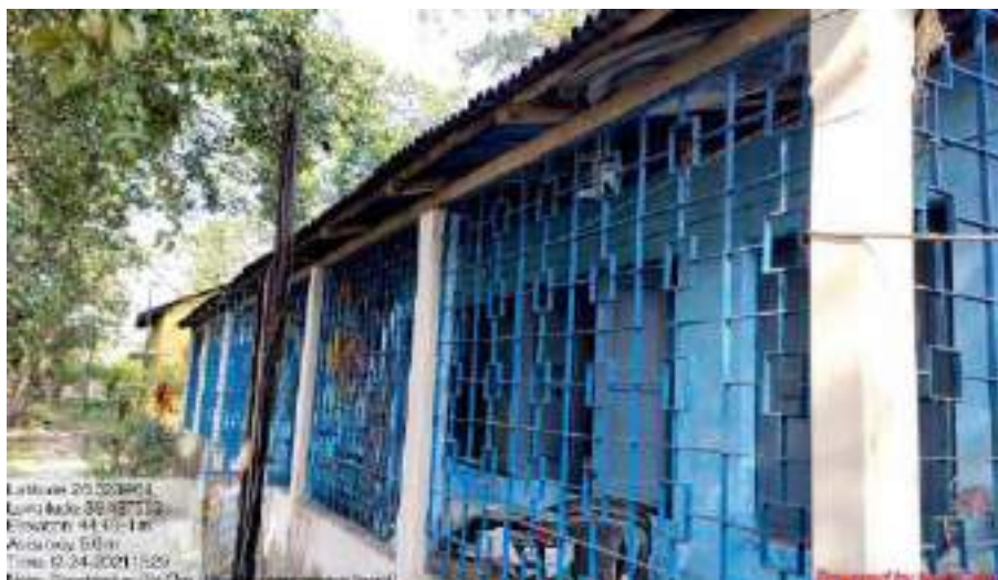
Cooch Behar Division: Maintenance of staff quarter
