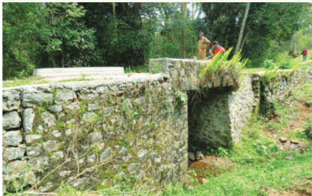
Bridge at Kalyanappara, Thekkady Range in Iddukki to improve connectivity
