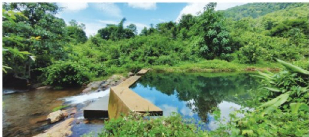
Construction of check dam at Kalaketty Parathode
