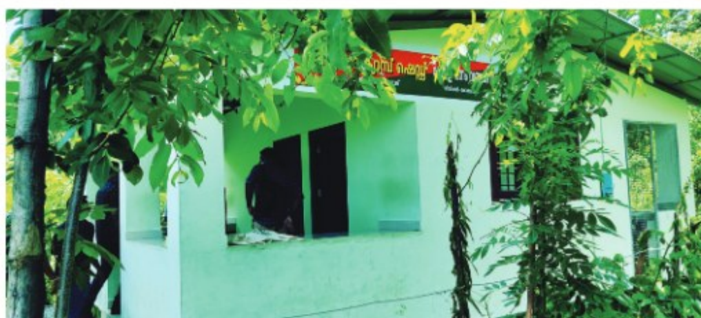
Construction of wireless repeater station cum Campshedat Kottappara in Neduvakkad Forest Station
