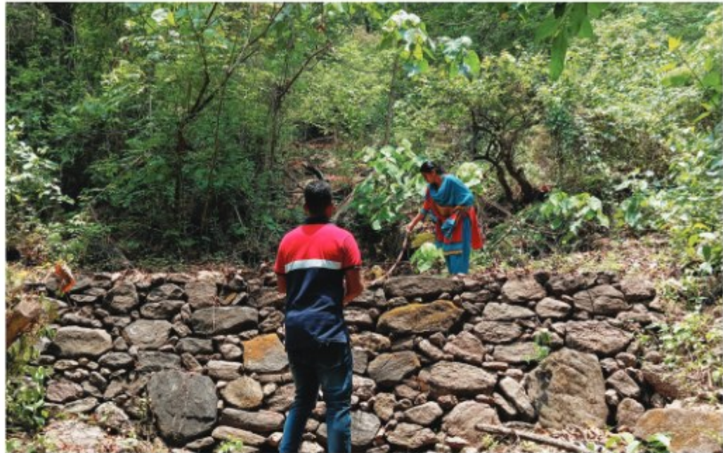
Inspection of gullies at Eco-restoration zone, Olavakkode
