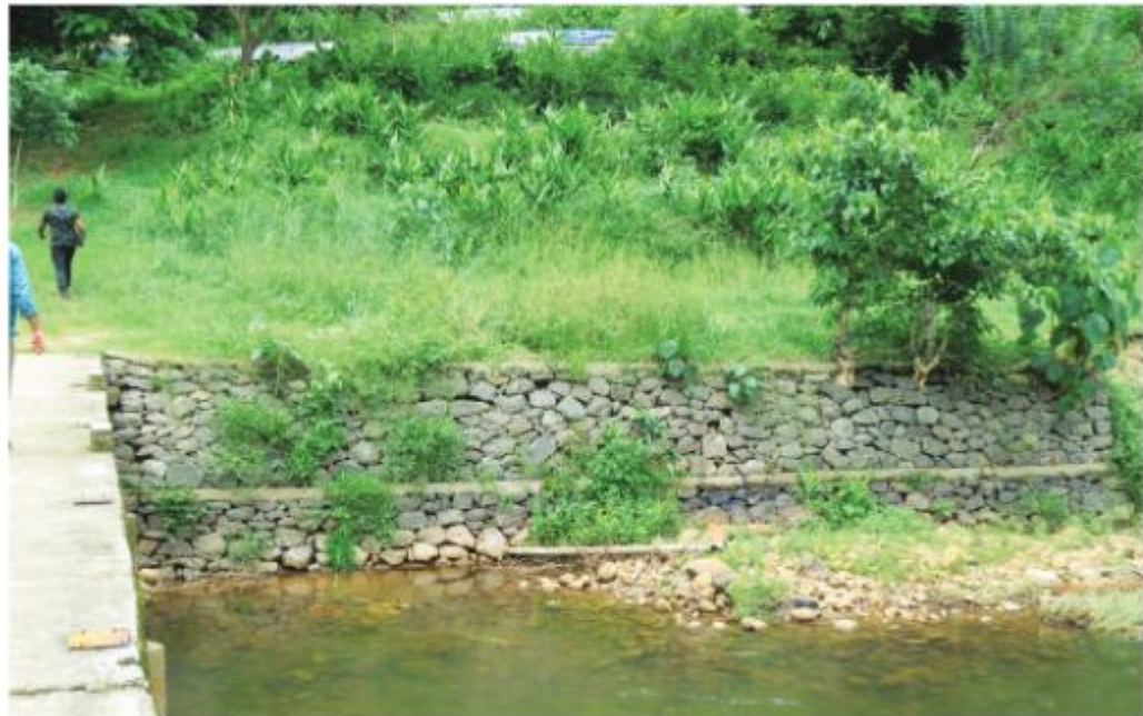
River bank stabilisation along Azutha River
