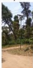
Provision of street lights
