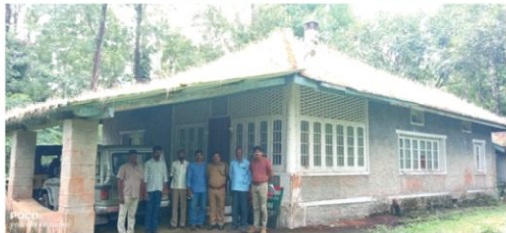
Sooryapara Camp shed at Nelliyampathy
