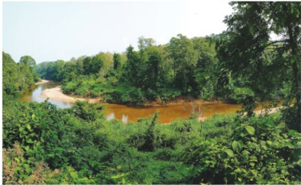
River Bank Stabilisation along Achenkovil river in Konni Division
