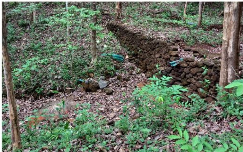
Gully plugging at Chimony
