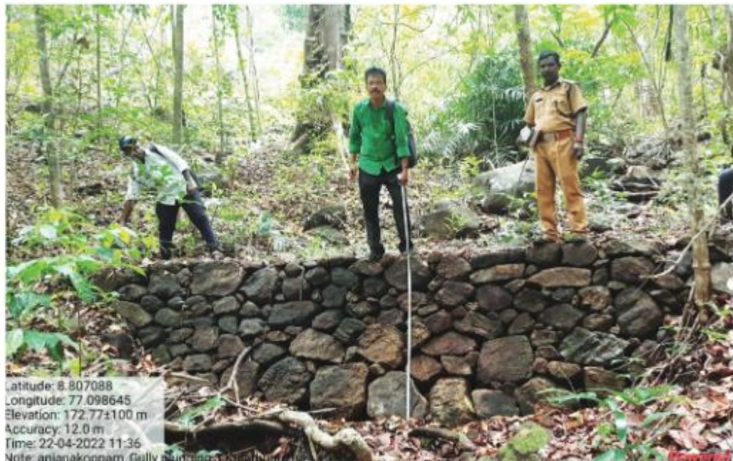
Gully plugging at Anchanakkoppam
