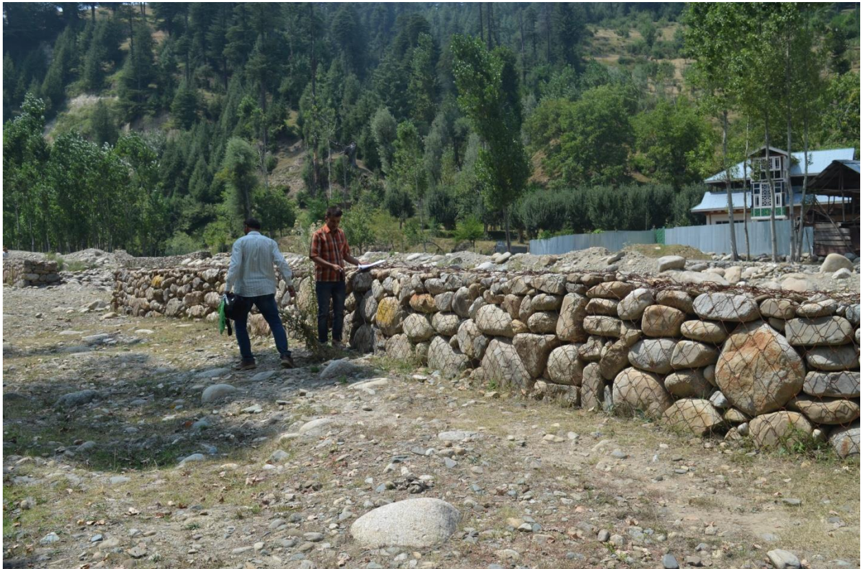
Closure 5-6 Dobi Mohalla DRSM work (2018-19) Soil & Water conservation division (Kupwara)
