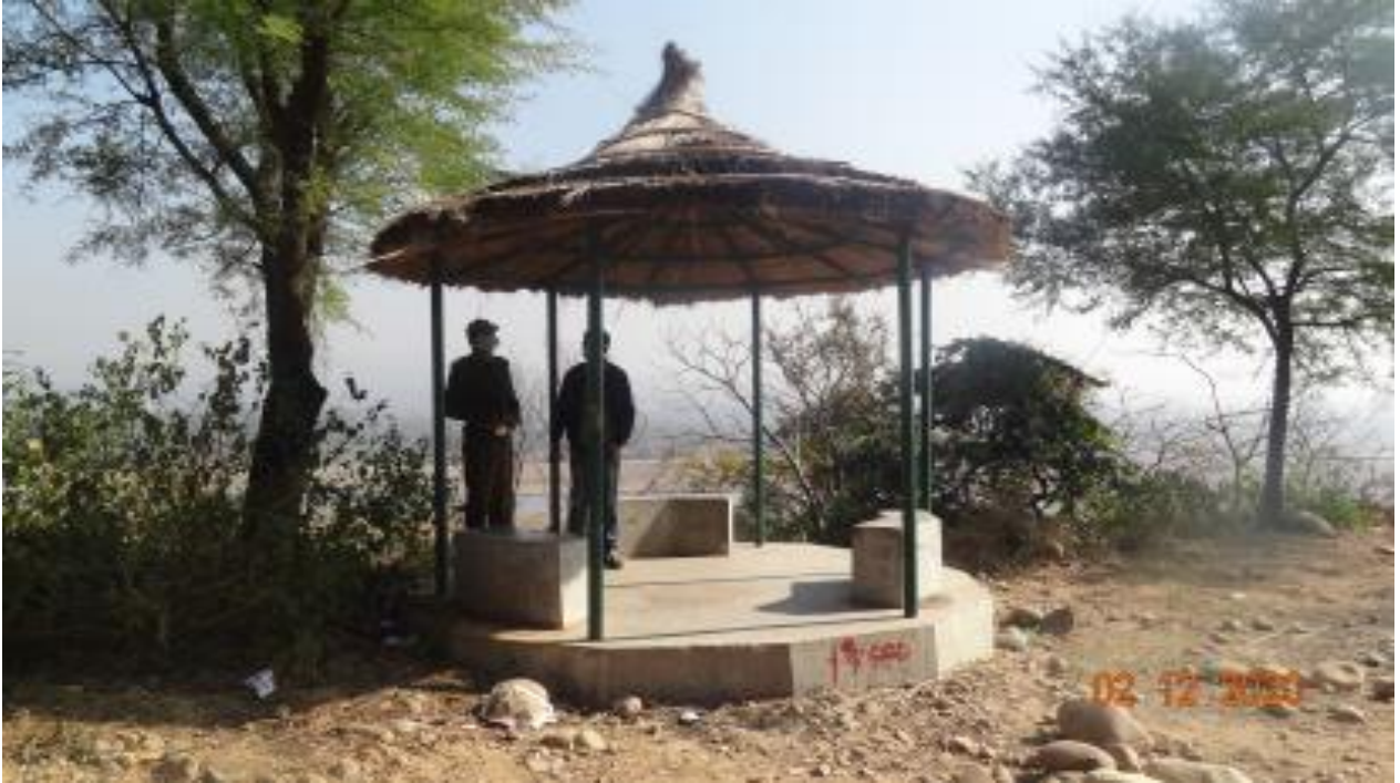
Construction of View Point, Jasrota (Kathua Wildlife Division)
