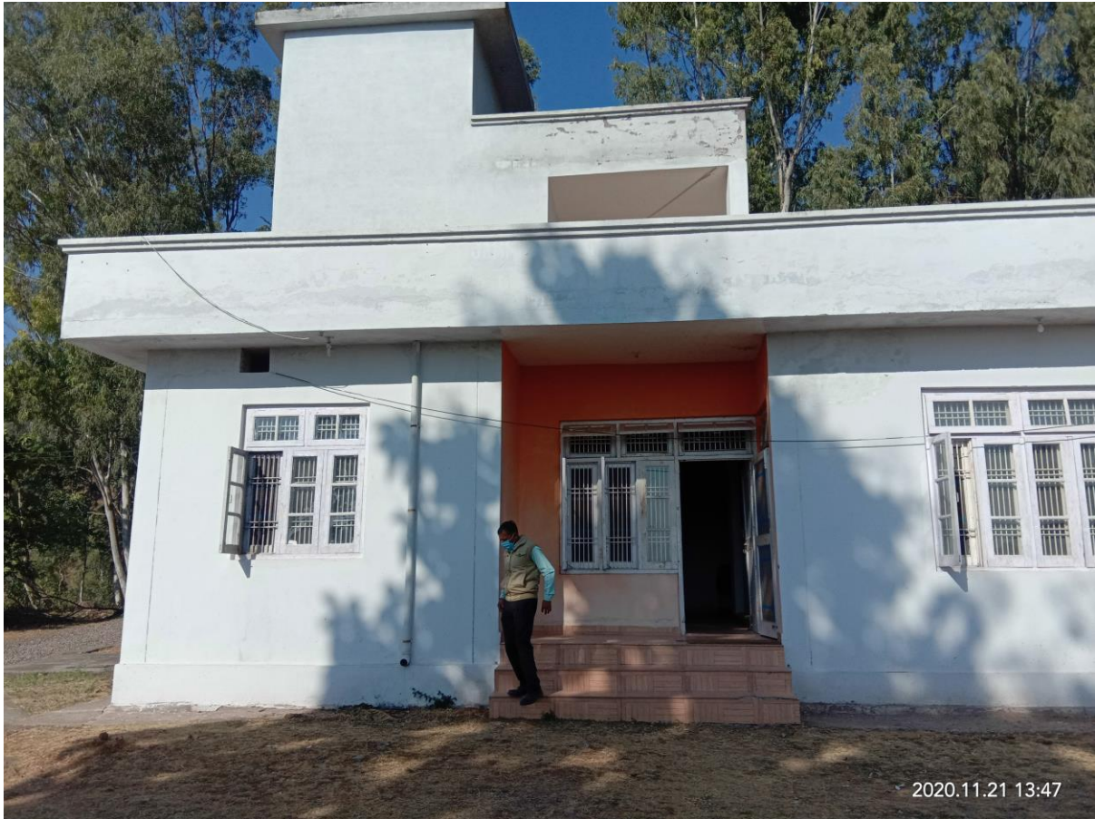
Range Office Building at Billawar
