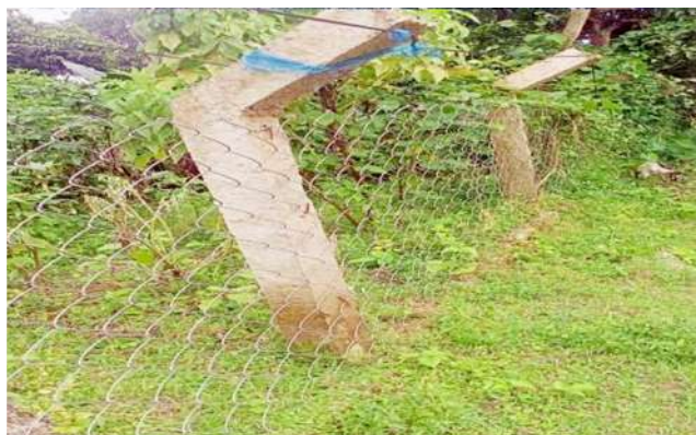
Chain link mesh fencing
