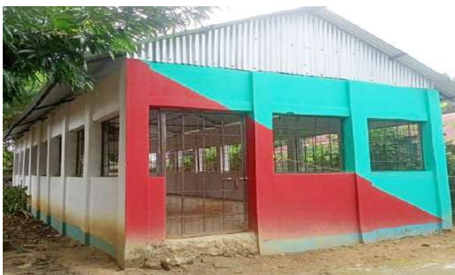
Timber Shed with GCI sheet roofing
