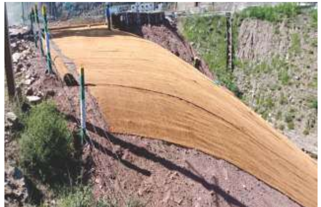
Co. 14/Btt. Nashri Adjacent to Tunnel (Batote Forest Division)
