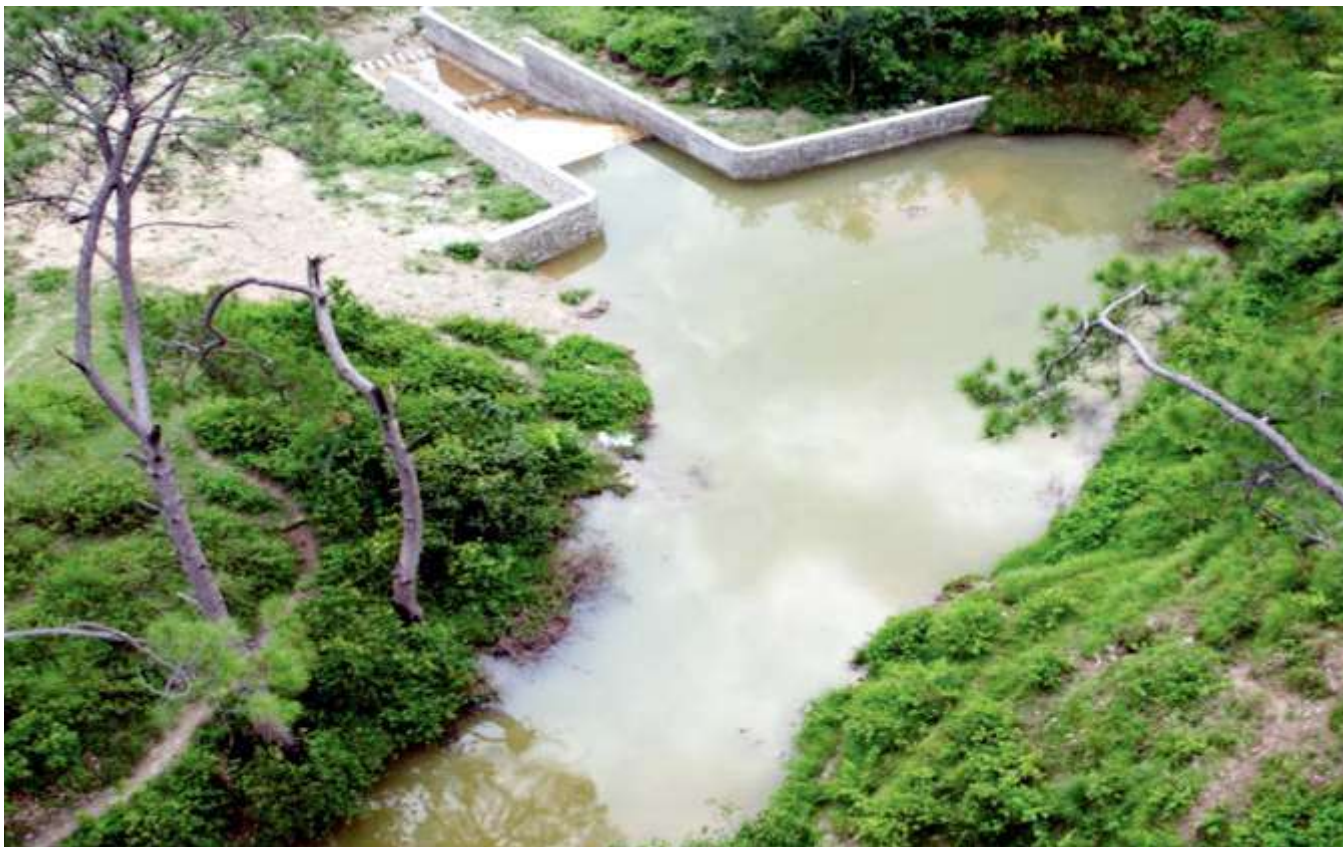
Construction of Pond at Bajoka Chak, Kathua
