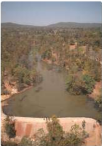
EARTHEN DAM AURA NAALA
