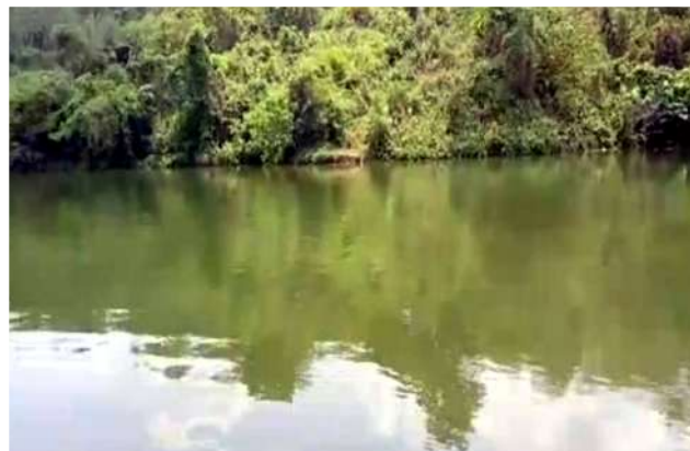
Check Dam at Silaguha JFMC under Silachari VC Forest Sub-Division, Jatanbari-2022-23)
