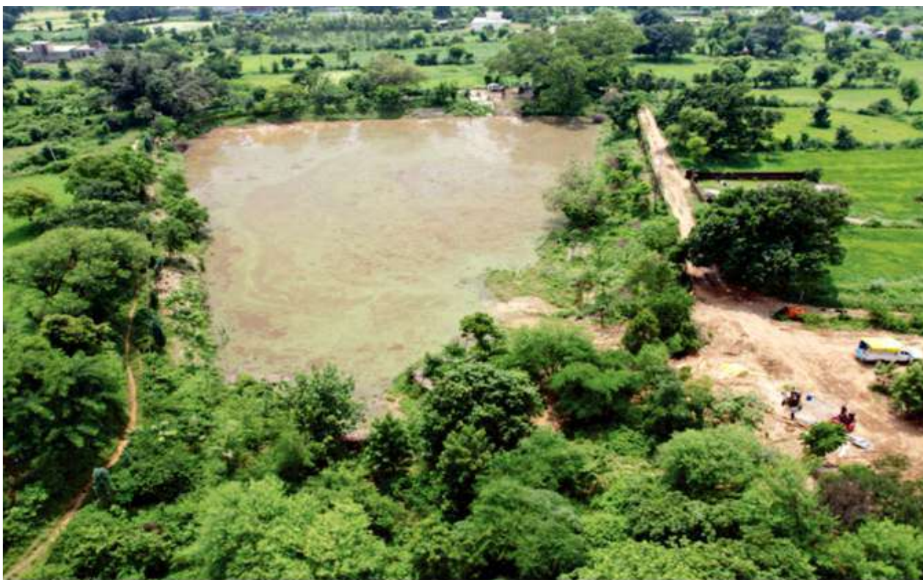
Construction of RCC Check Dam at Phangeri, Kathua
