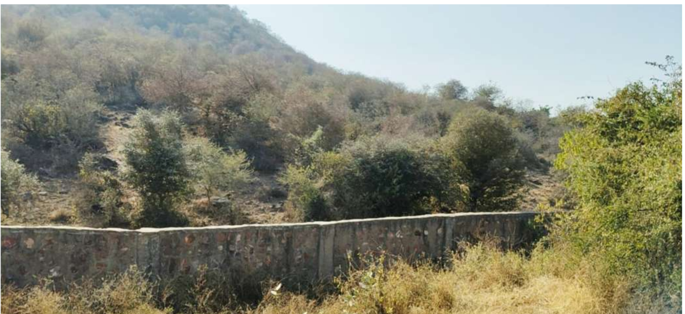
Figure : Construction of Boundary Wall in Bharatpur
