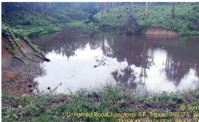
Check Dam at Jamircherra JFMC- CAMPA- 2021-22
