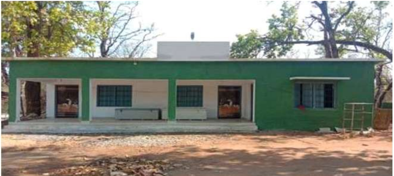
Range office construction: Range Pataur, 2022-23
