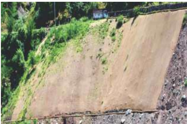
Co. 14/Btt. Nashri Adjacent to Tunnel (Batote Forest Division)
