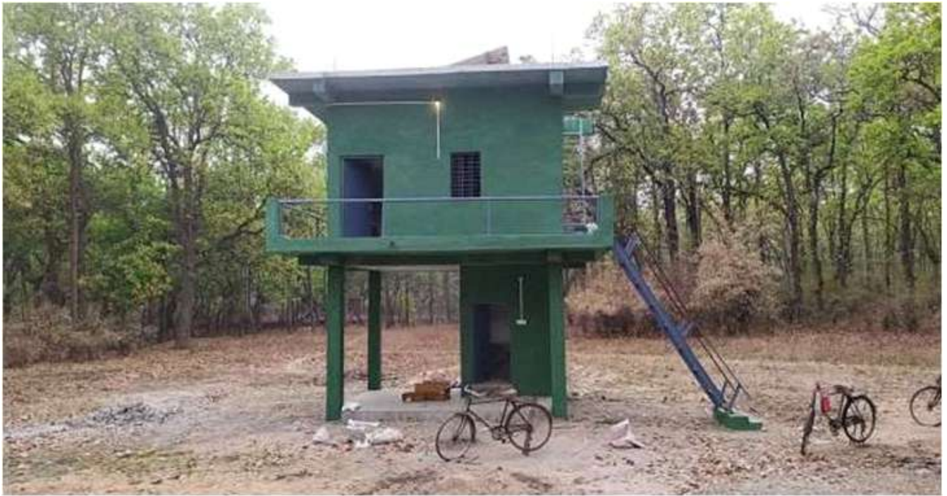
Range: Tala, Beat: North Gohdi, Mahaman Camp, 2021-22 Raised patrolling camp with Solar power installation 2022-23
