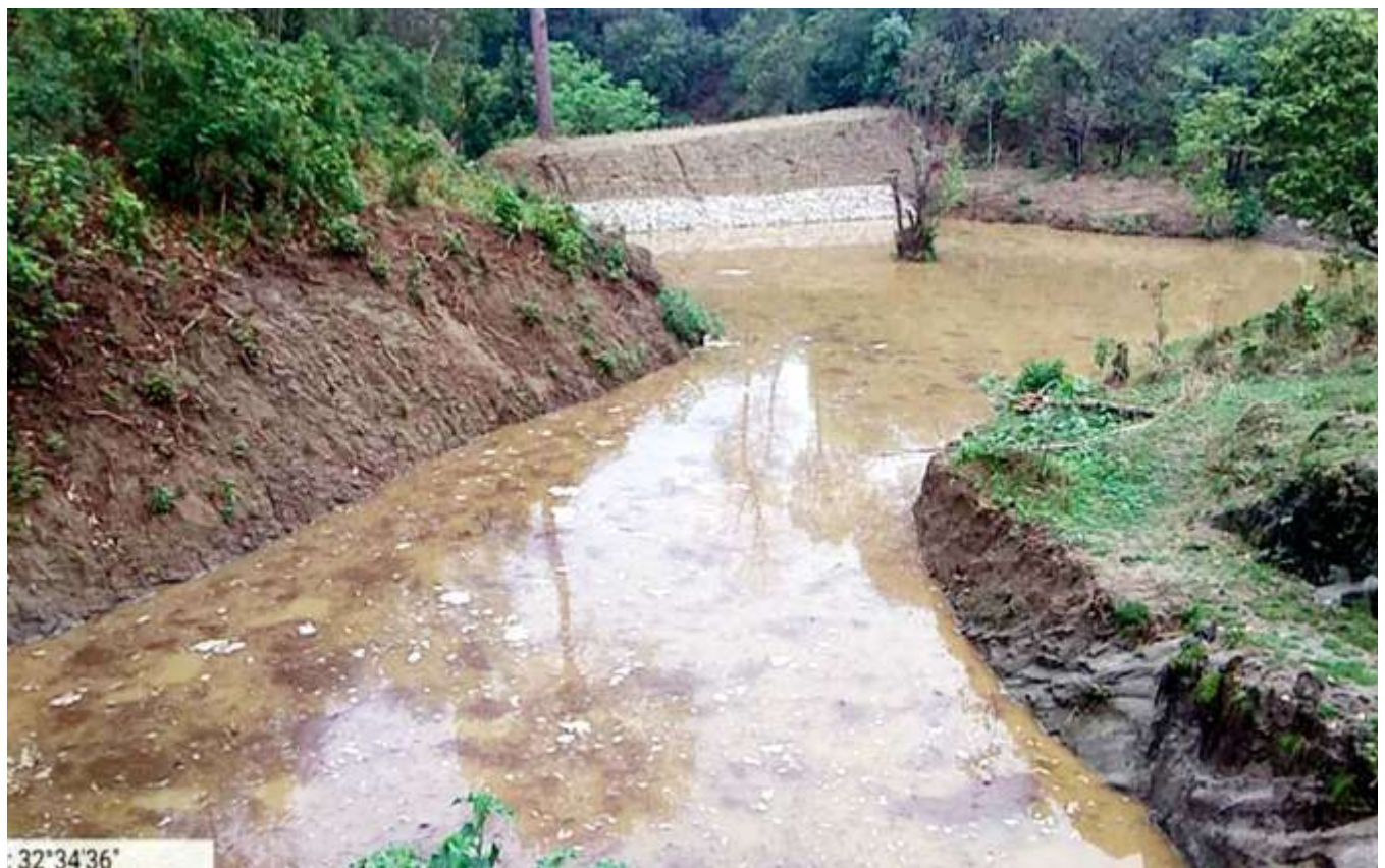
Construction of Pond at Bajoka Chak, Kathua
