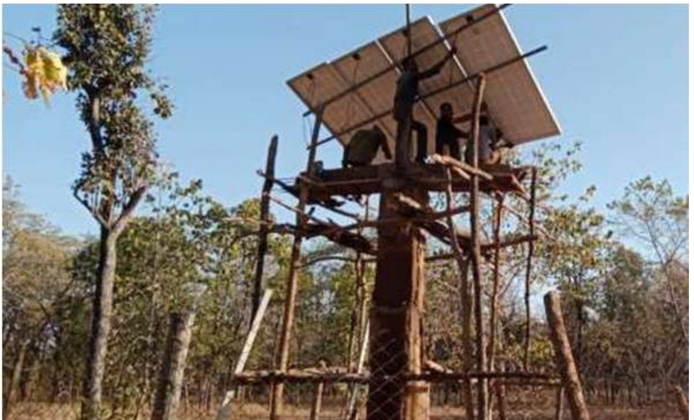
Range: Tala, Beat: Elephant camp Bathan, Year 2021-22 Raised Solar power plates a strategy adopted to save it from wild elephants
