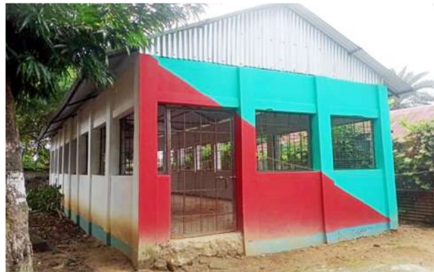
Timber Shed with GCI sheet roofing
