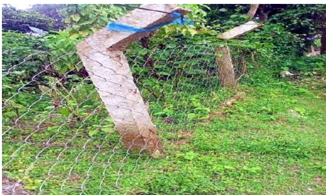
Chain link mesh fencing
