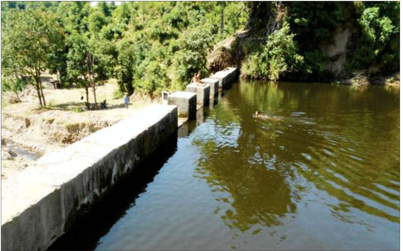
Earthen dam for gully control and water harvesting at Kathua
