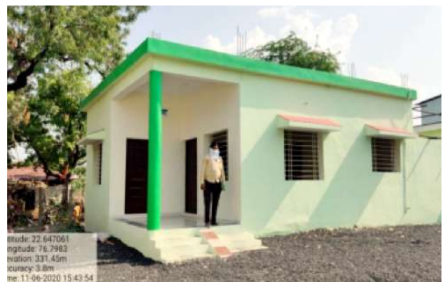
Forest Guard Residence (Kannod) Dewas Division, Kannod Range 2020-21
