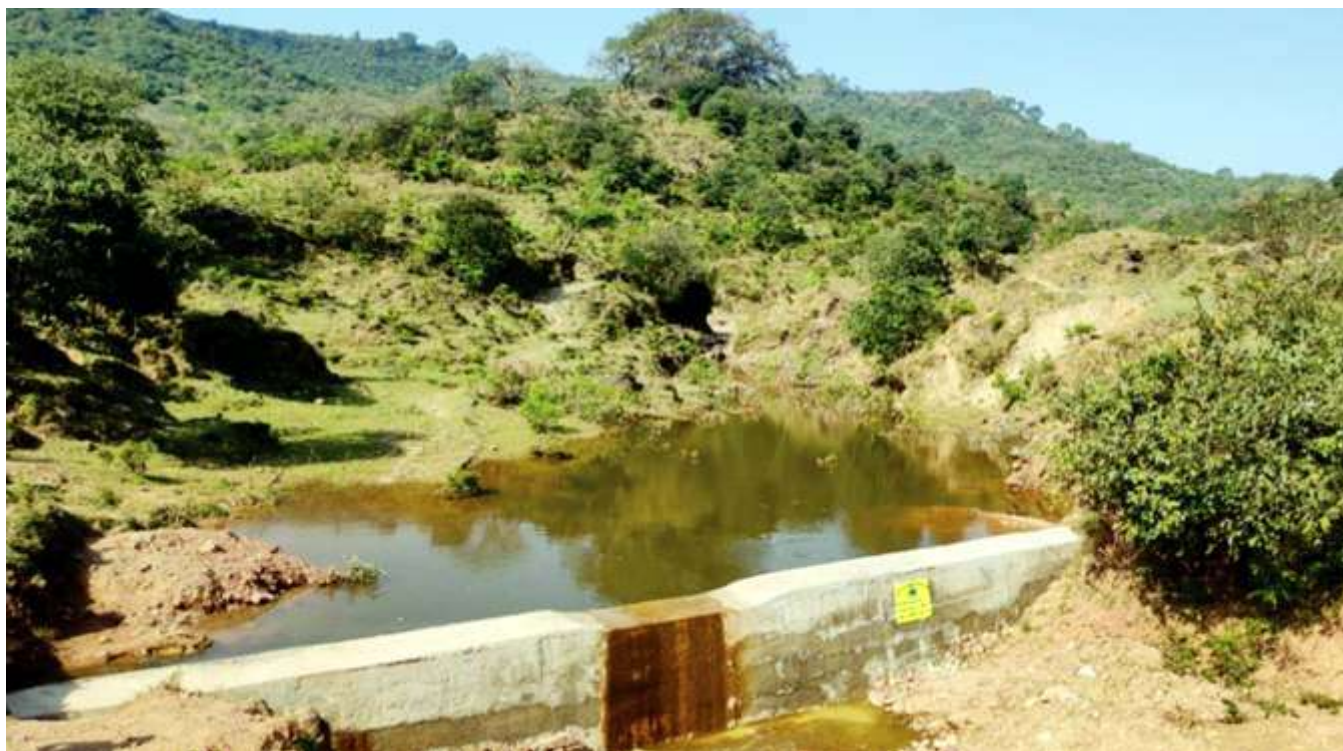
Construction of RCC Check Dam at Simble Lehar Jammu
