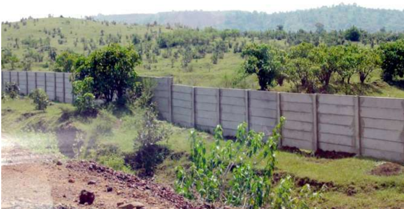
Boundary Wall Construction in Highly Sensitive Forest Areas
