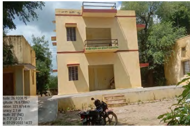
Construction of Office-cum-Residence at Sikarai in Dausa Division (Year 2021-22)
