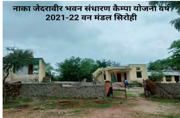
Maintenance of Naka Jedaraveer Building in Sirohi Division (Year 2021-22)
