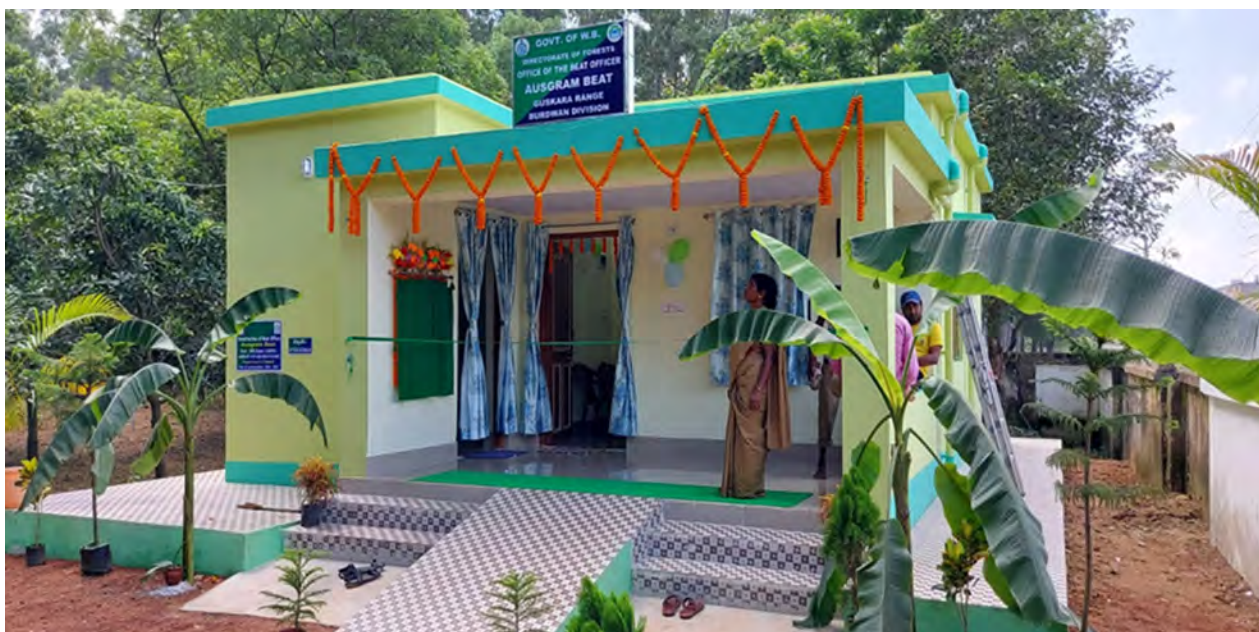
New construction of Beat Office at Ausgram, Guskara Range, Burdwan Division.
