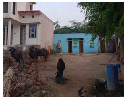
House construction in Behro
