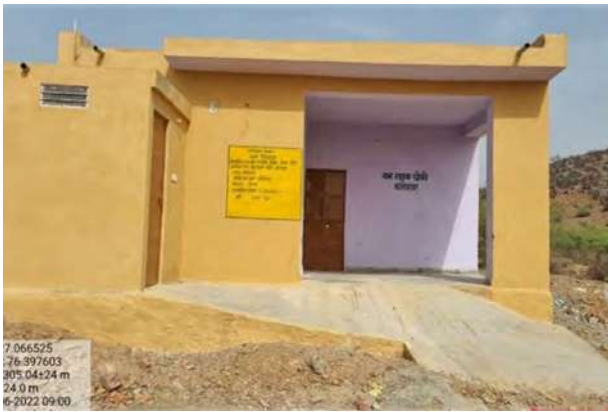
Construction of Forest Guard Chowkie at Koleswar, Dausa Division (Year 2021-22)
