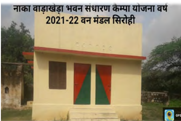
Maintenance of Naka Wadakheda Building in Sirohi Division (Year 2021-22)
