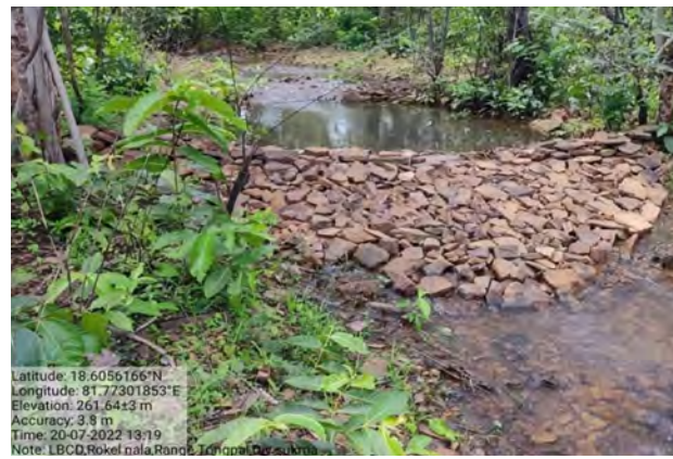
Loose Boulder Check Dam
