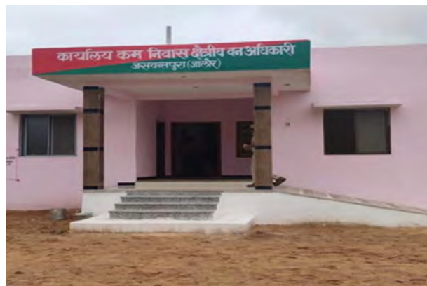
Construction of Office-cum-Residence at Jaswantpura, Jalore Division (Year 2020-21)
