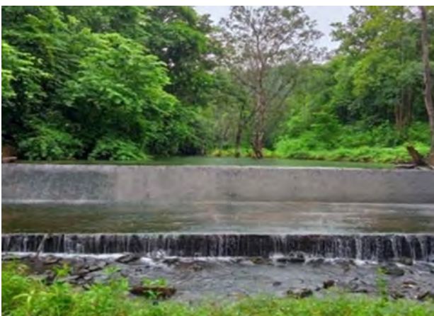
Check dam in Jamshedpur
