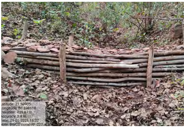
Brush Wood Check Dam
