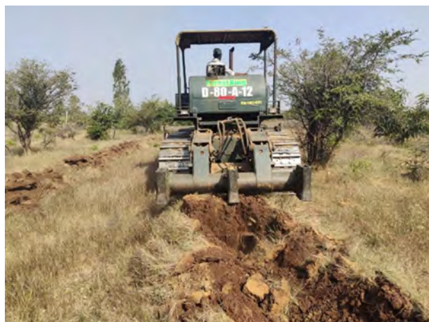
Advance works using D-80 bull dozer
