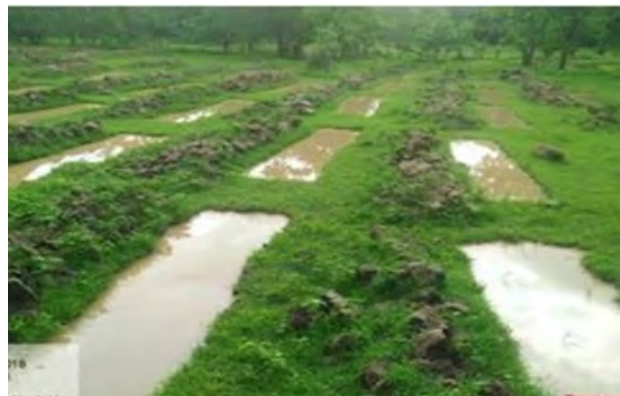
Soil & Moisture Conservation Works: Staggered Contour Trenches-342000 nos
