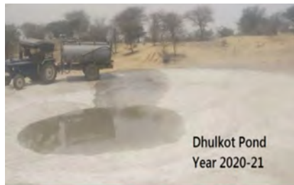
Water pond Fartiya Dhulkot Distt. Bhiwani
