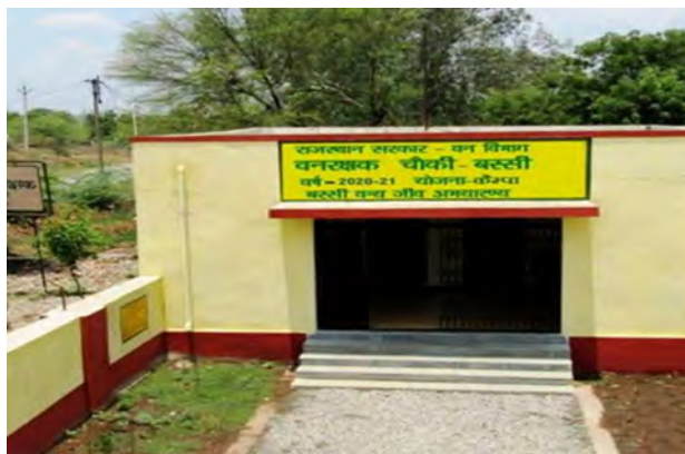
Construction of Forest Guard Chowkie at Base WL Sanctuary (year 2020-21)
