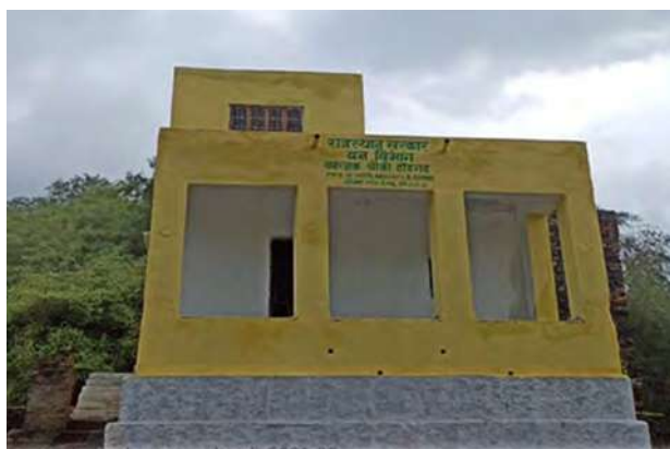
Construction of Forest Guard Chowkie at Todgarh, Rajsamand Division (Year 2020-21)
