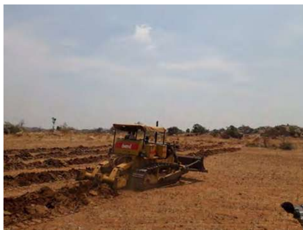
Continuous trenches formed
