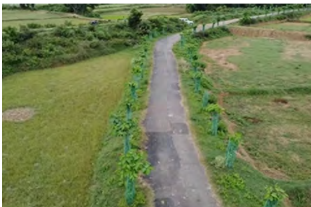
Avenue plantation (single row) along rural road in Berhampur Division
