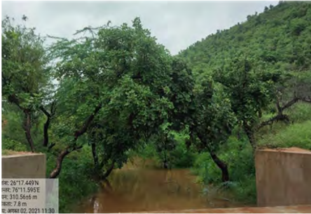
Construction of Anicut in Jaisamand Sanctuary, Udaipur (Year 2020-21)
