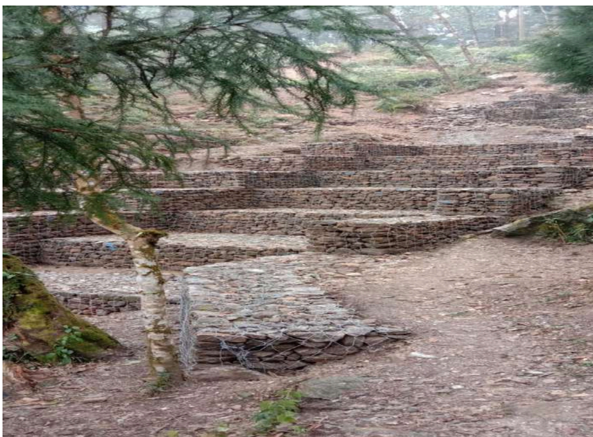
SMC works (boulder sausage wall), Mahaldiram-II (Lower Section), East Balason Catchment Range, Kurseong Soil Conservation Division, West Bengal
