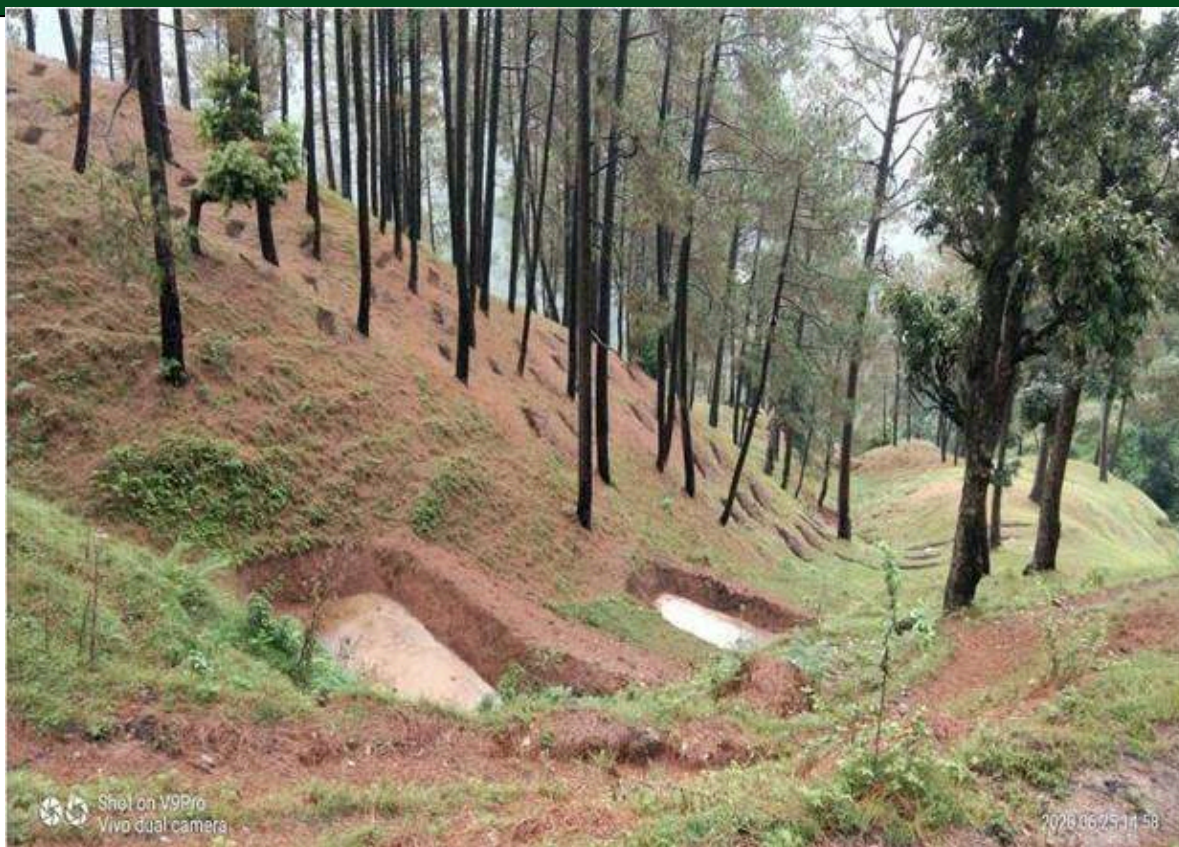
SMC Works (contour trenches and chal khal works), Bhowali Range, Nainital Forest Division, Uttarakhand
