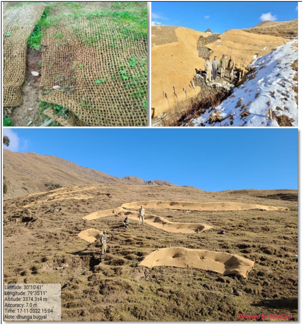
Coir/Geo Jute netting techniques to stabilize landslide & erosion, Uttarakhand
