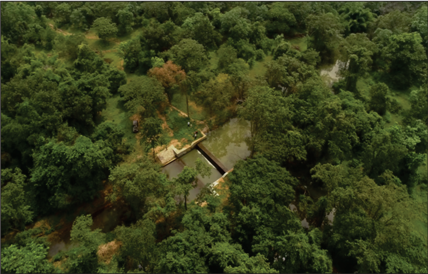
Check Dam, Balod, Chhattisgarh
