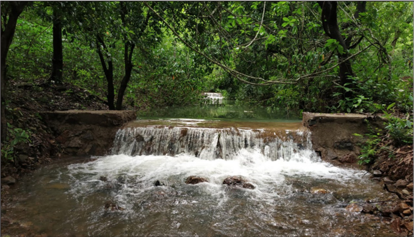
Cement Mortar Check Dam at Dharbandora, North Goa, N – 150 22'58.18" E – 0740 8'53.85"
