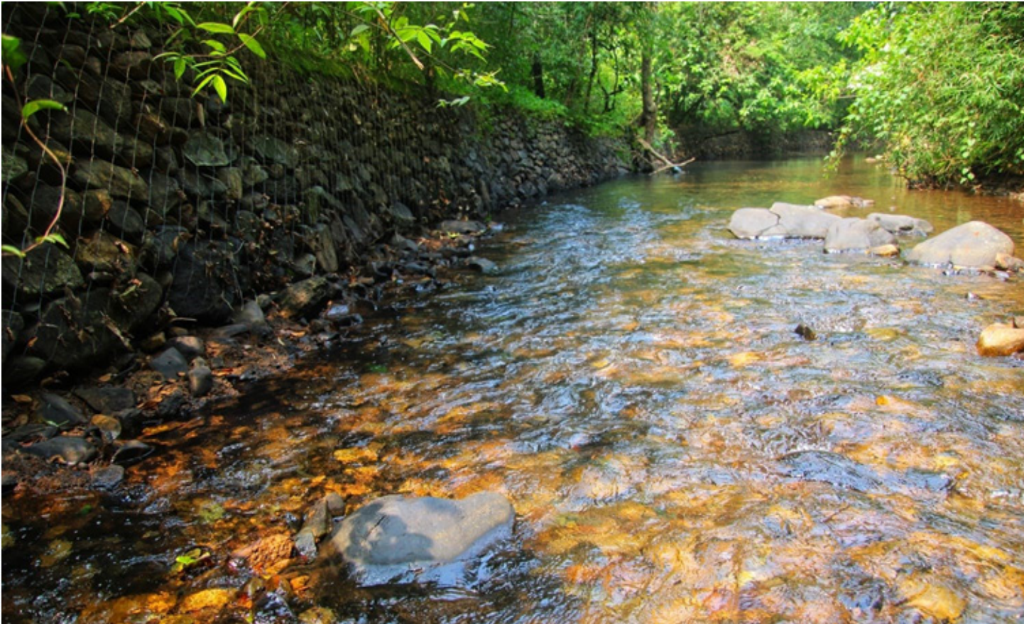
Retaining Wall at Gurkhe-Dharbandora, North Goa, N – 150 25'44.30" E – 0740 7'43.00"
