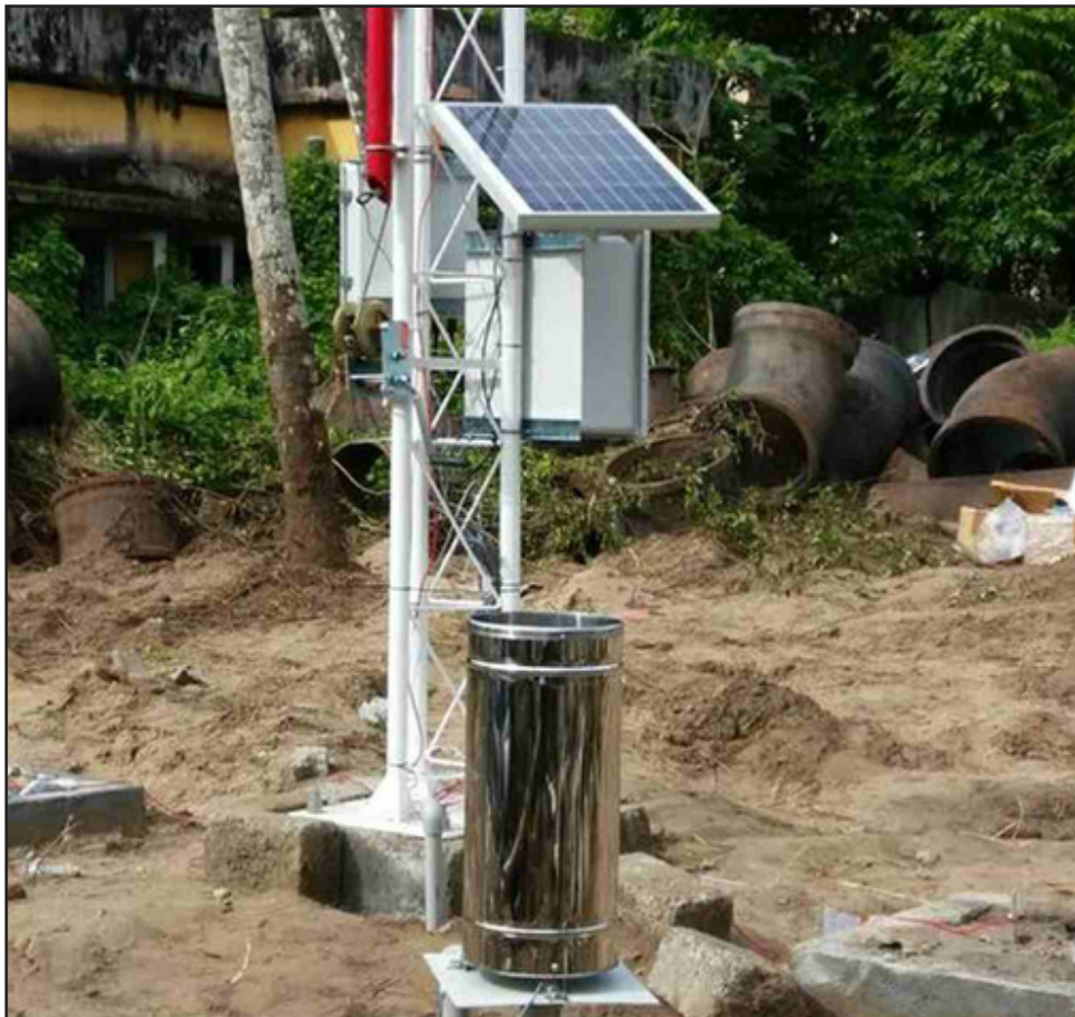
Automatic Weather Station, Goa
