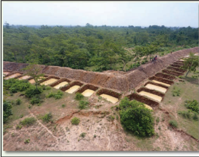
Graded Earthen bund along foot hills under Keonjhar WL Division, Odisha
