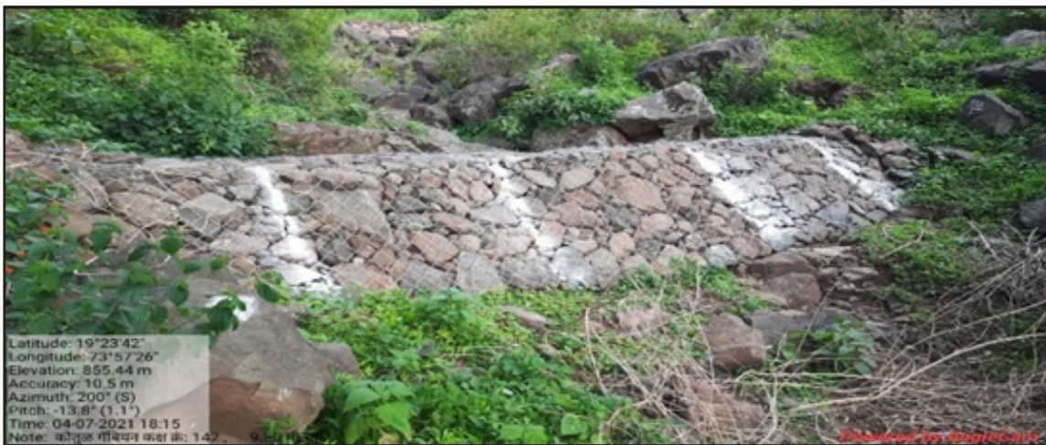
Gabion at Bandhara, Bhore Division, Maharashtra
