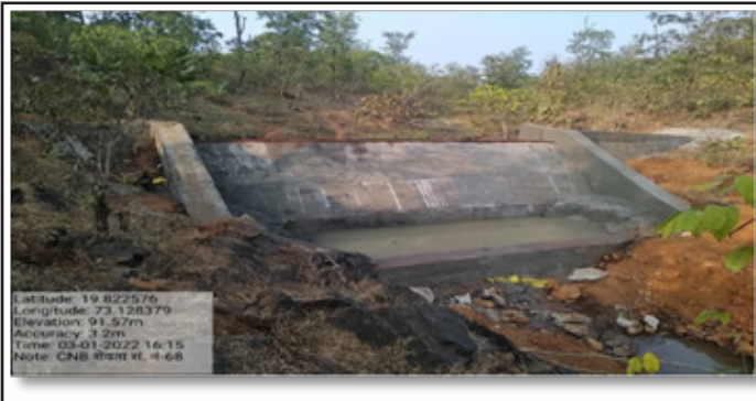
Check Dam Chauk, Maharashtra
