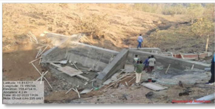
Check Dam Shevta, Maharashtra
