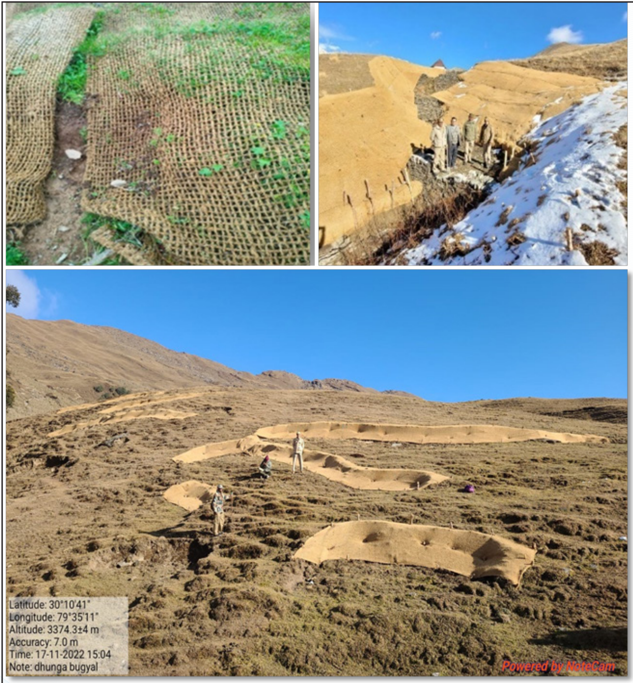
Coir/Geo Jute netting techniques to stabilize landslide & erosion, UTTARAKHAND
