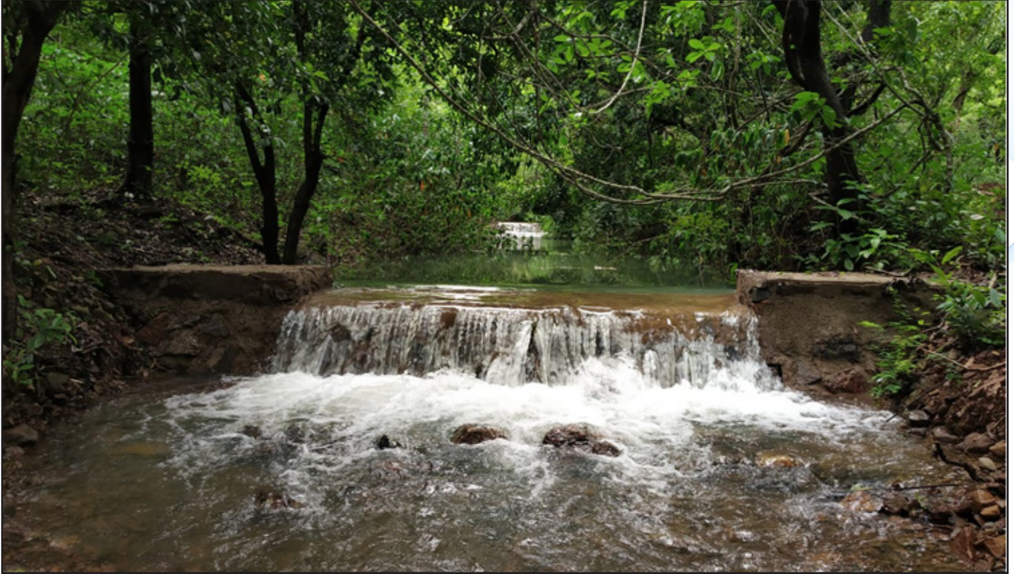
Check Dam at Dharbandora, NORTH GOA, N – 150 22'58.18" E – 0740 8'53.85"
