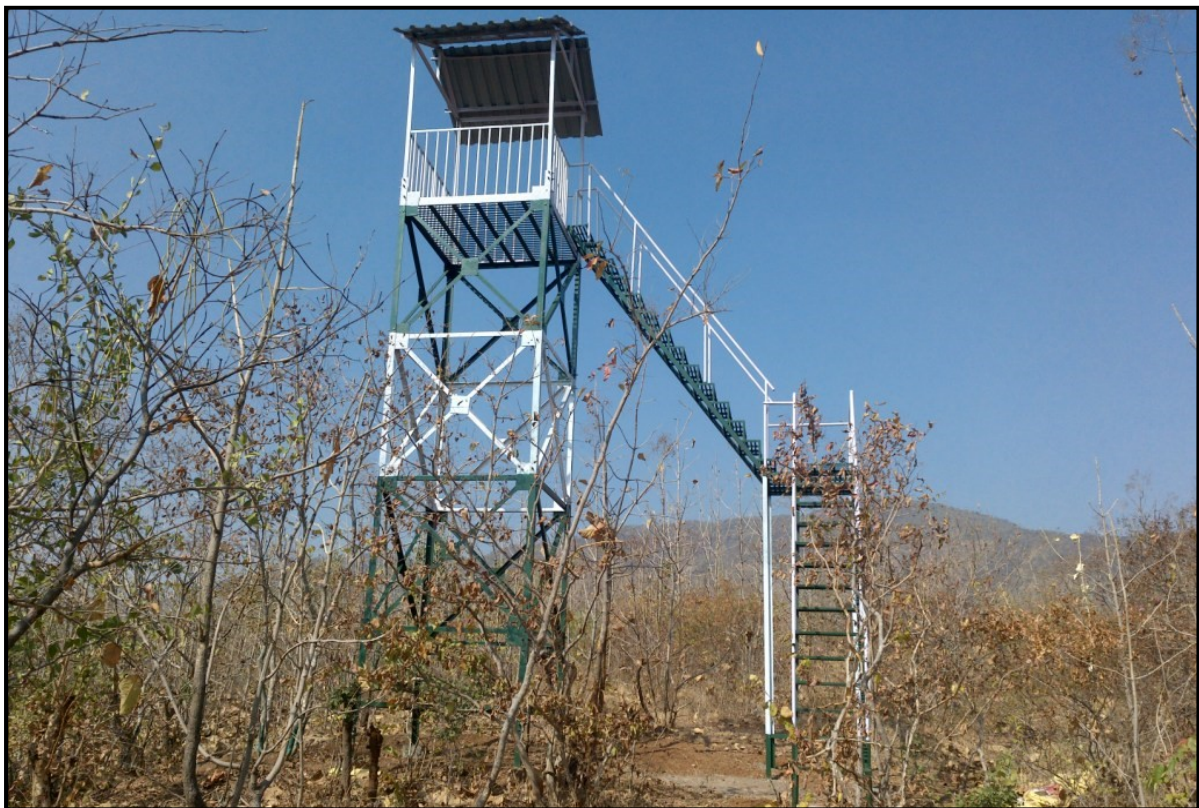
Watch Tower at Nagadevi in Yaval Division, Dhule Circle.
