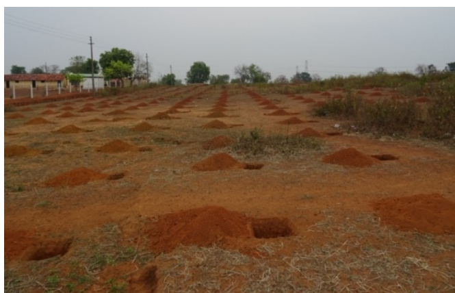
P.P.O. Works in Wadsa Division, Gadchiroli Circle, Compartment No.: 812
