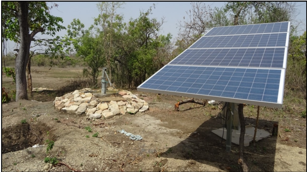
Creation of Borewell with solar pump in Chandrapur Division, Chandrapur Circle.
