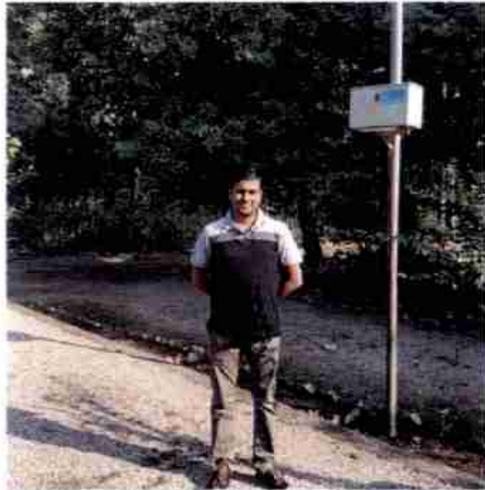
Fig 8: Division- Sonbhadra, Solar Unit location- DFO office
