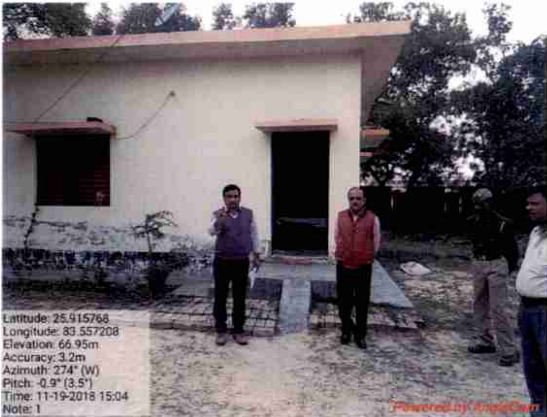
Fig.11: Division- Mau, Staff Quarter Location- Range Mau
