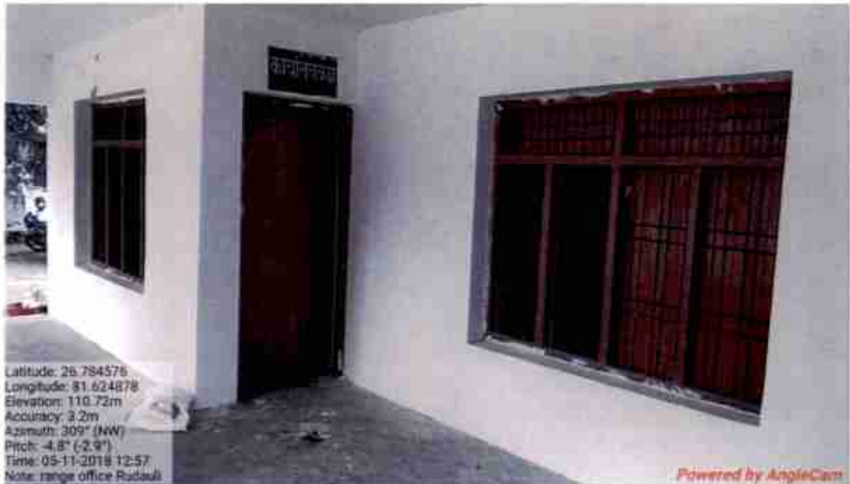
Fig 9: Division- Faizabad- Staff Quarter Location- Type-3 Quarter at Range Office Rudauli
