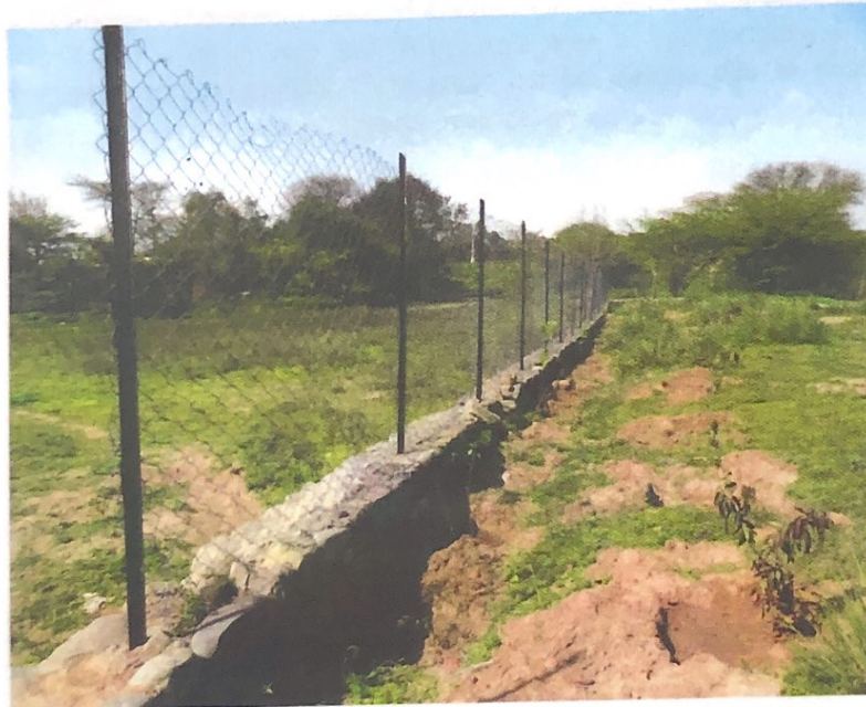
View of chain link wire fencing at Maloya CAMPA site
