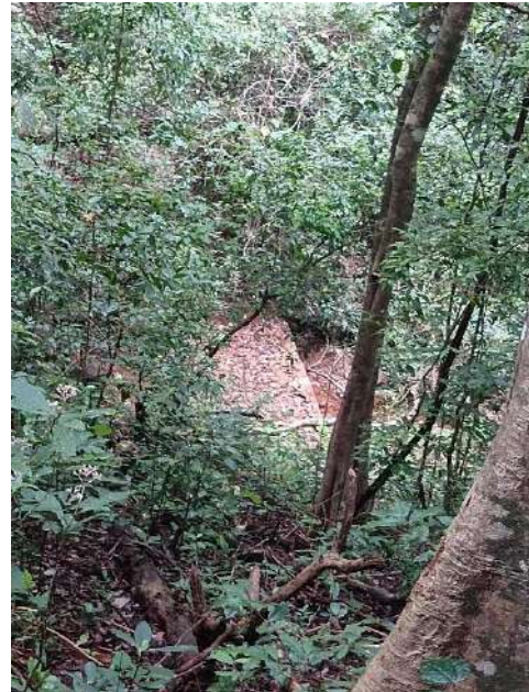
Gully Plugging at Vakkalar
