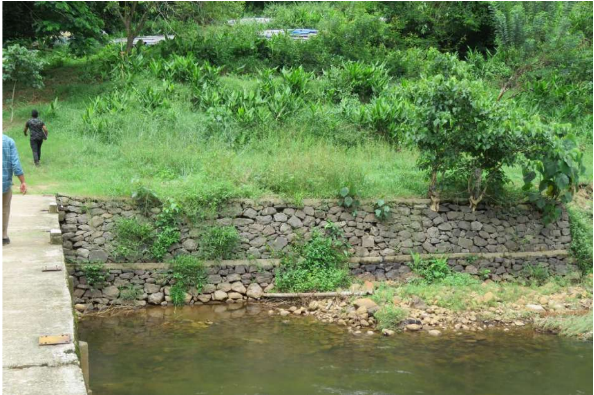
River bank stabilisation along Azutha River
