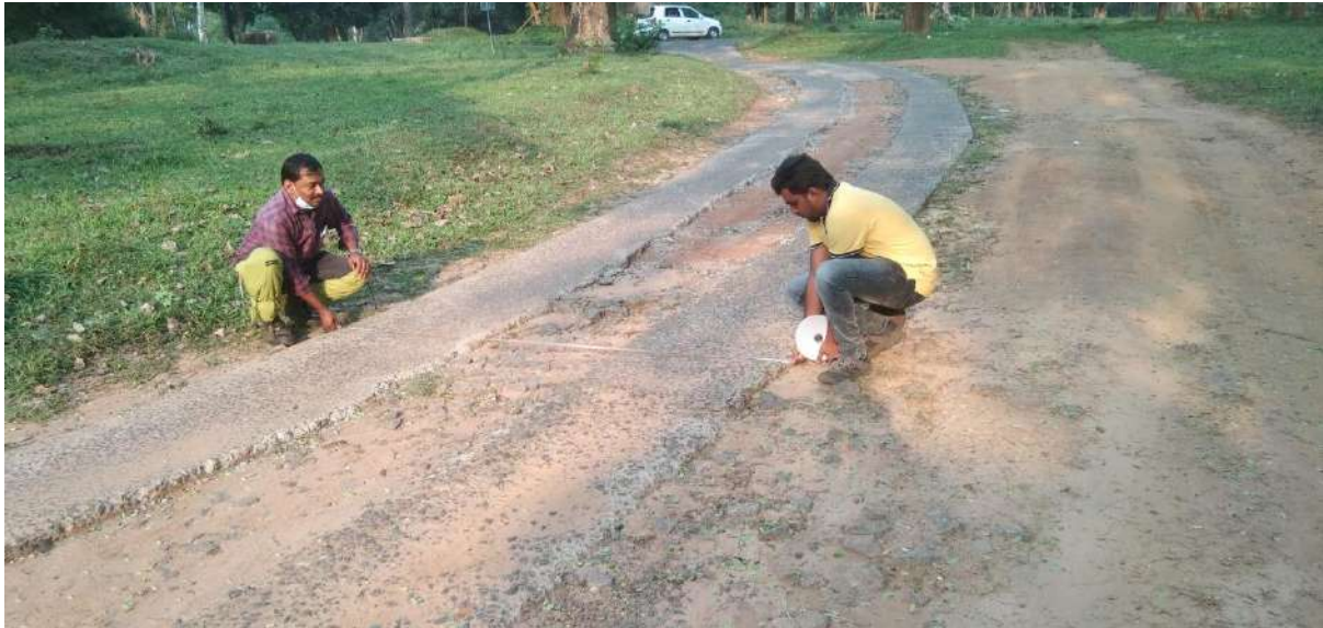
Wheel track concrete near tribal colony
