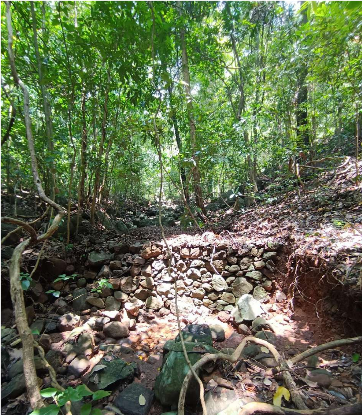
Gully Plugging at Kattikuzhy
