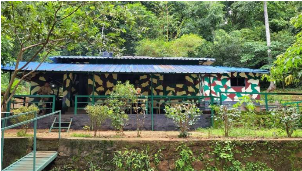
Campshed at Site 4
