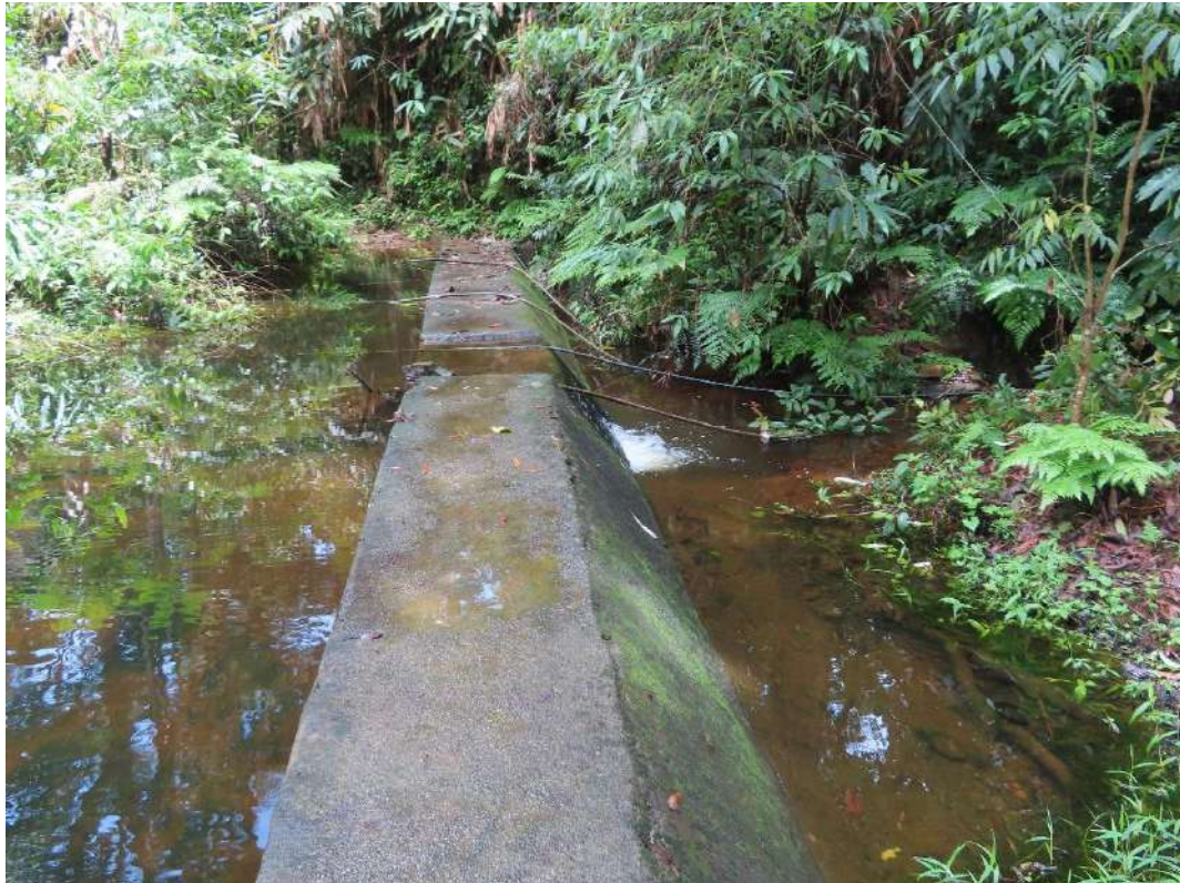
Check Dam at Kambany Kudy
