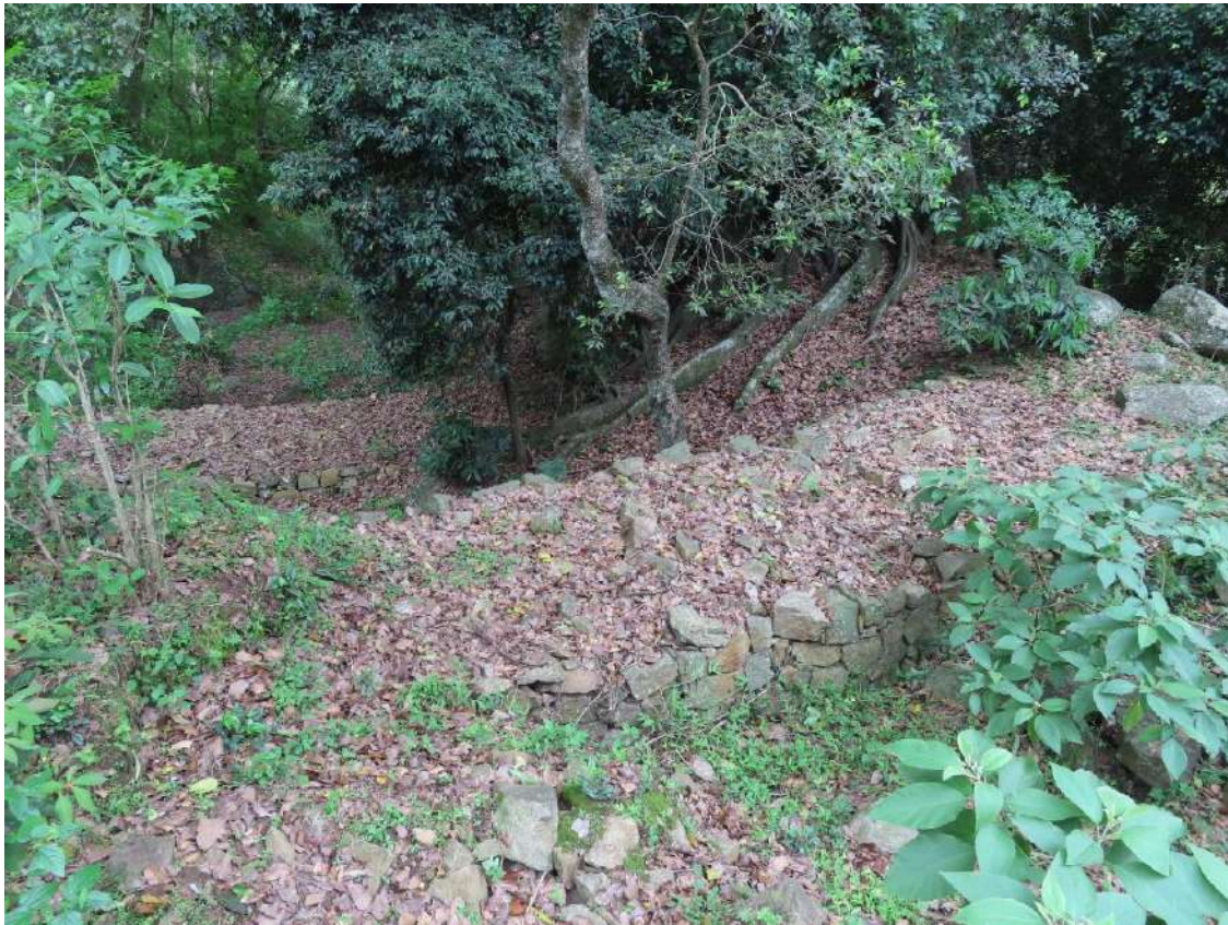
Present status of gully plugging at Pobson Oda Thodu at Marayoor
