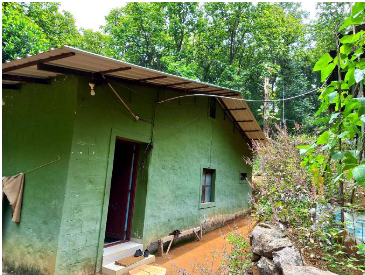
Camp shed at Thudukki
