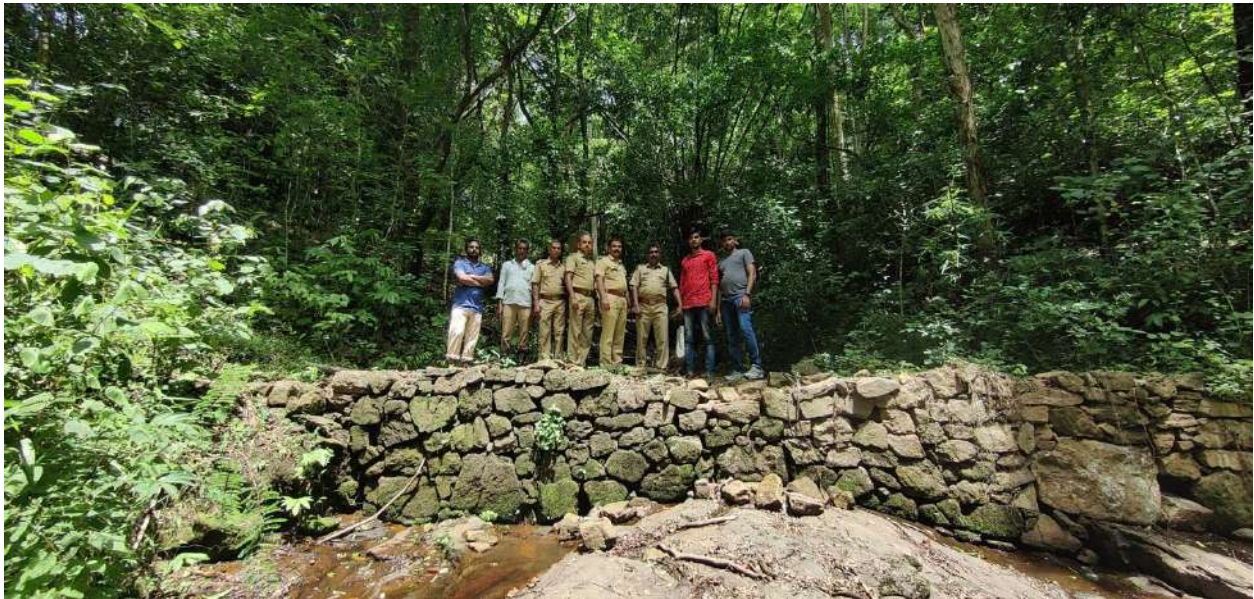
Gully Plug at Ayyapancoil
