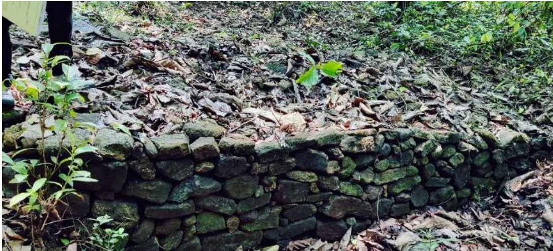
Present status of gully plugging at Kozhippanna Thodu at Marayoor
