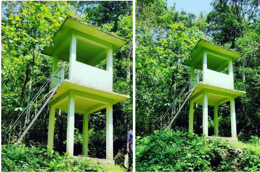
Forest Watch Station at Kothamangalam
