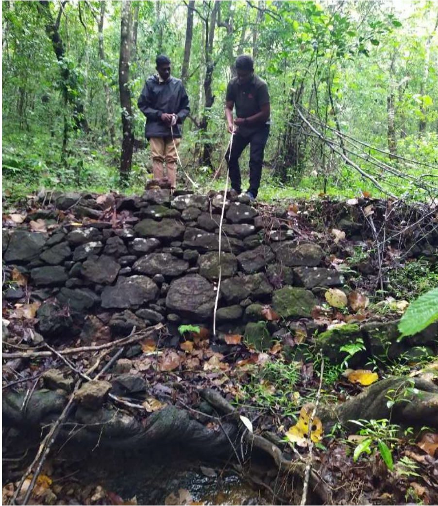
Gully Plugging at Idukki WLS
