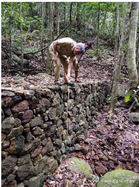
Gully plugging in four different locations
