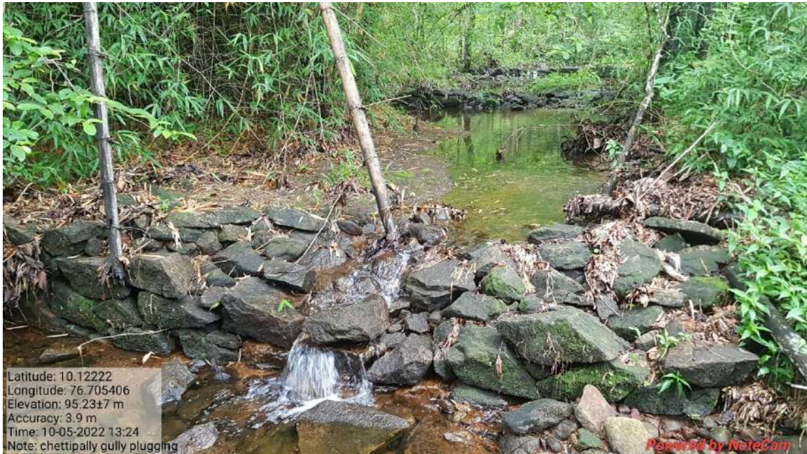
Chettipally gully plugging
