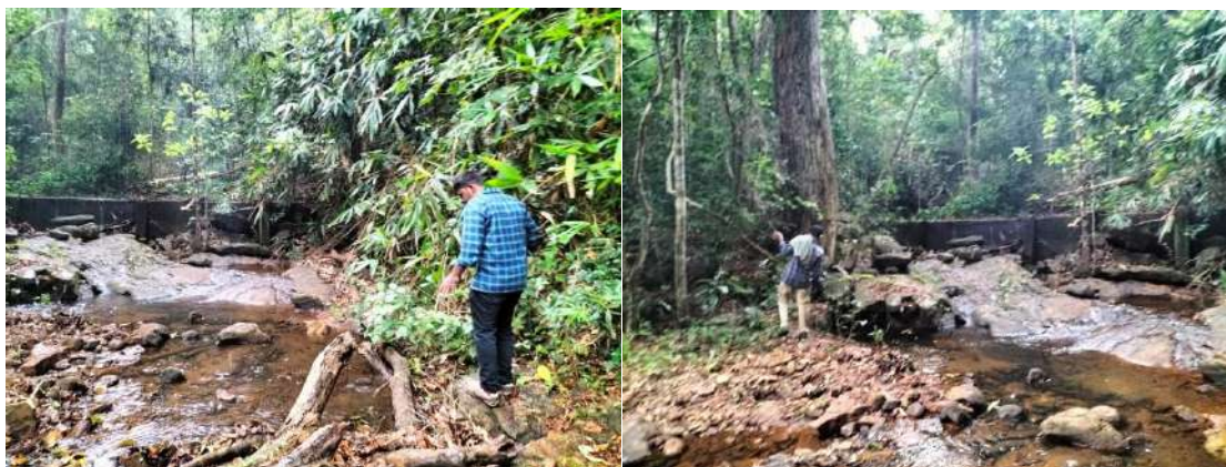
Check Dam at Site 5
