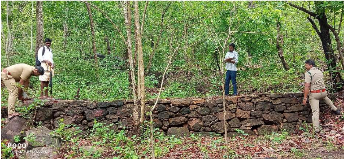
Inspection of the Kayyala at the site
