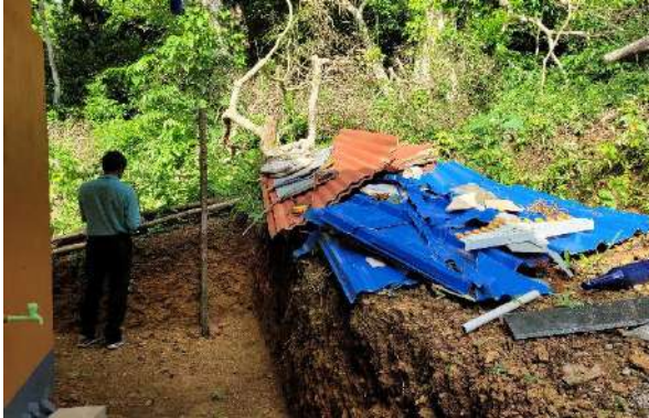
Debris of the Damaged structure at Site 2
