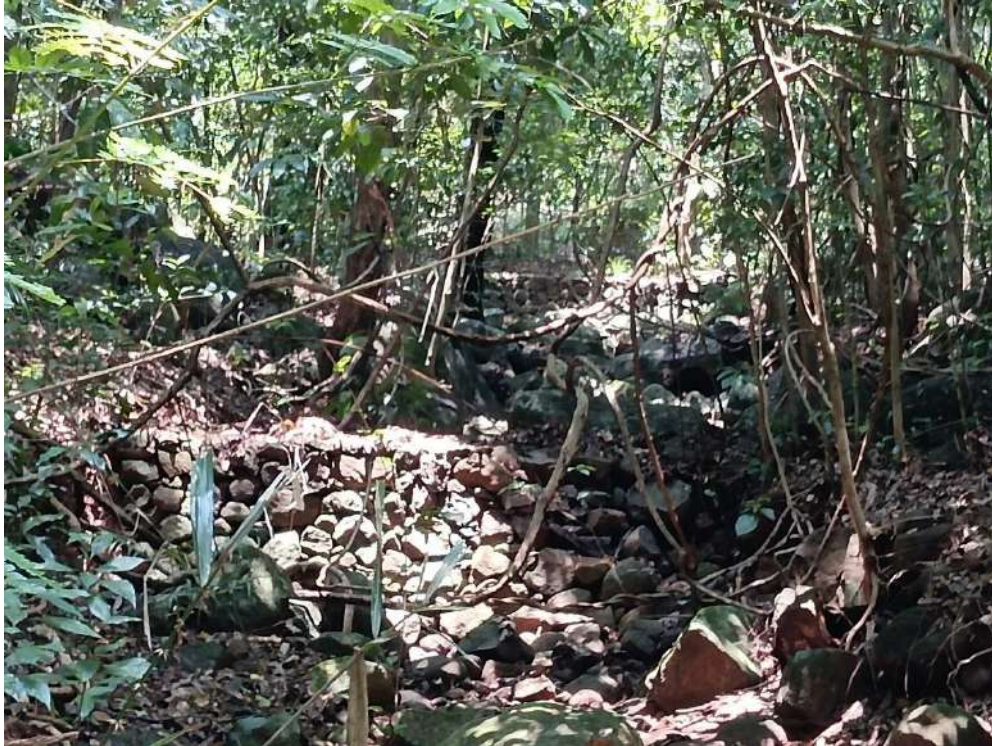
Gully plugging at Kattikuzhi
