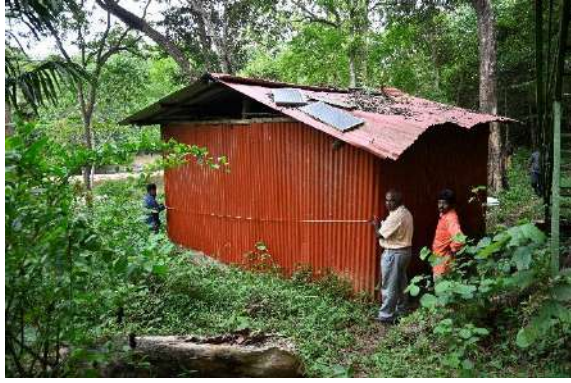
Campshed at Site 1
