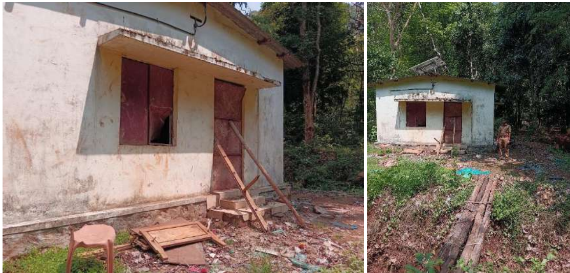
Camp Shed at Kattikuzhy with elephant trench
