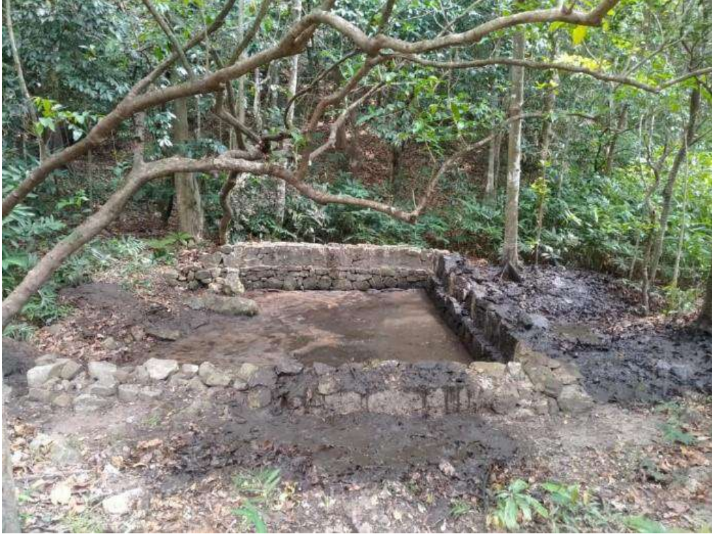
Water retention Structures
