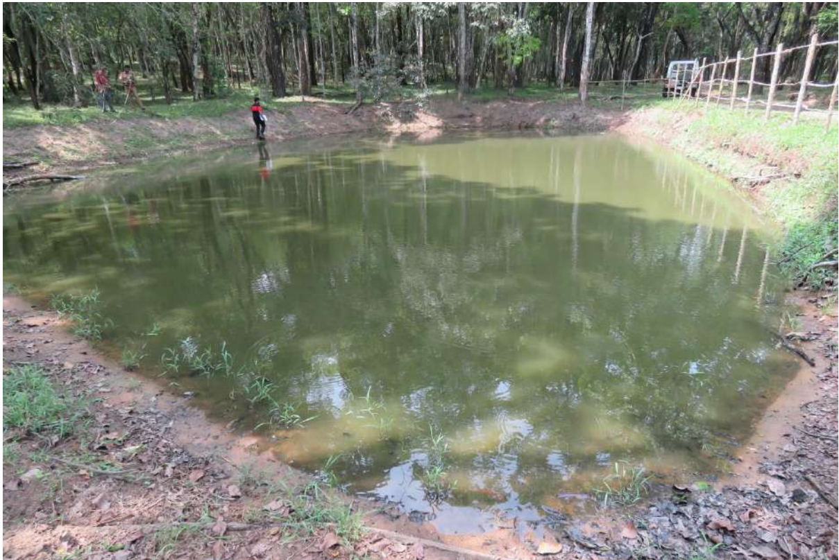
Desiltation of pond
