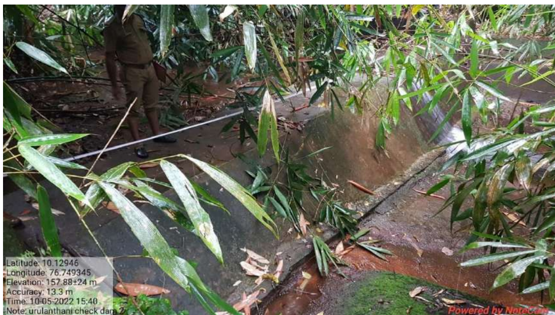
Urulanthanni Check Dam
