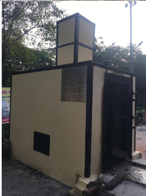
View of Green Crematorium at Green Park New Delhi which uses only 60-70 Kg/ Cremation of Cowdung Sticks
