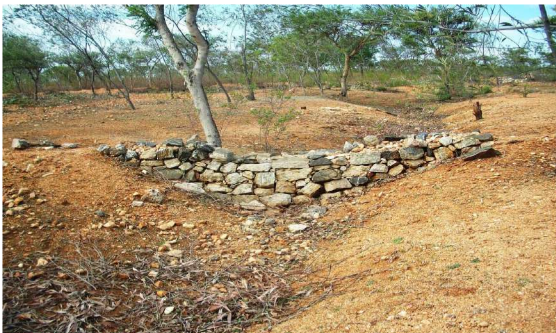
Fig 3.9: Loose Stone Check Dam
