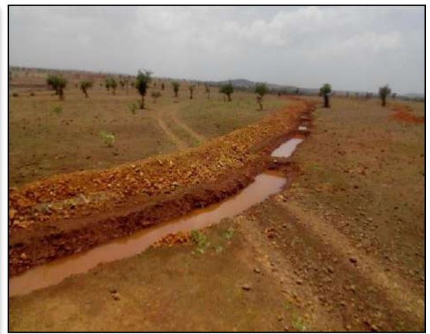
Fig 3.7: Continuous Contour Trenches (CCT)
