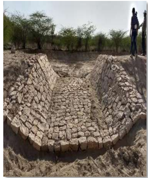
Figure (3.10): Mini-Percolation Tanks with waste weir
