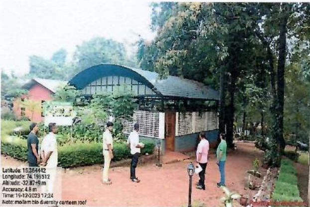
Physical evaluation of Canteen works in Bio Diversity Park
