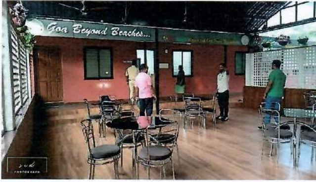
Verification of flooring and steel work inside canteen at Biodiversity Park
