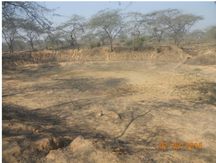
SMC Work (Pondage area of water pond)
