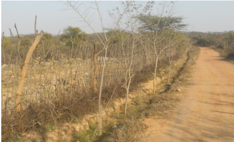
Barbed wire Fencing strengthened with locally available biomass
