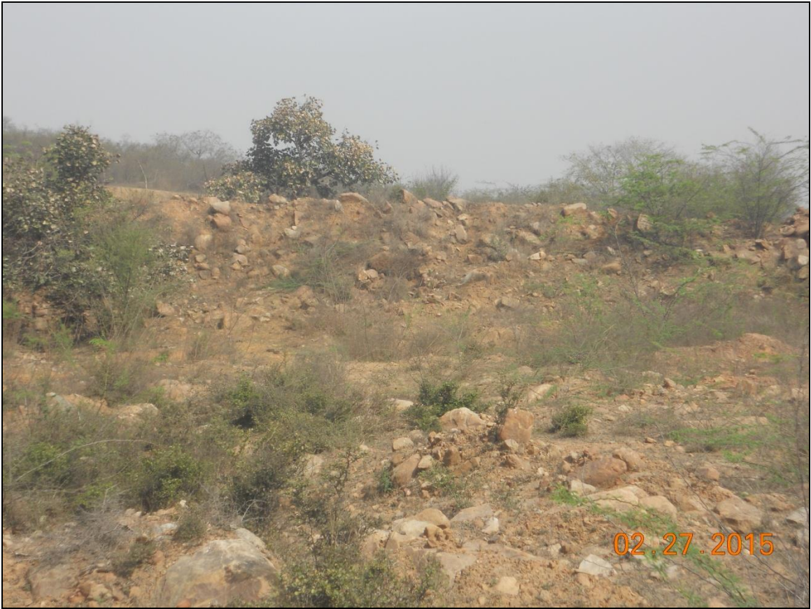
Earthen Check Dam
